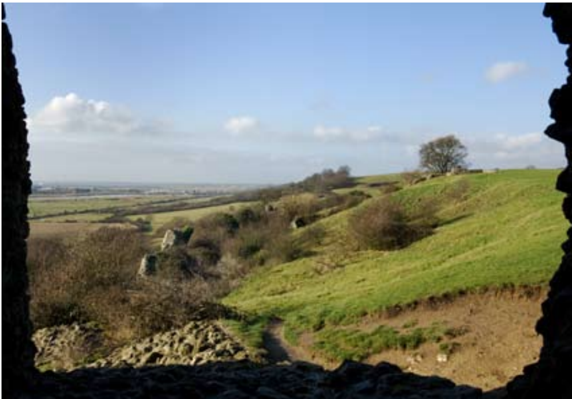
Figure 21 – Slumping on the south side of the bailey, from within the south east tower (© EH - DP068090, photographer Patricia Payne)
