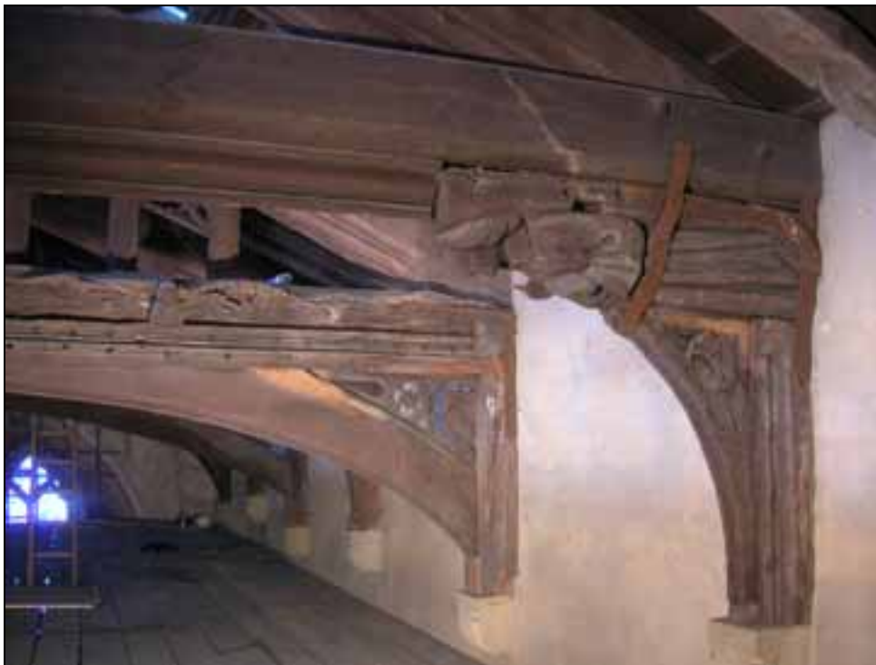
Figure 5: Nave roof; intermediary truss 6
