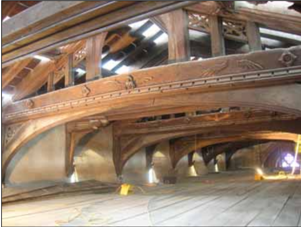
Figure 4: Nave roof; principal truss 3 in the foreground
