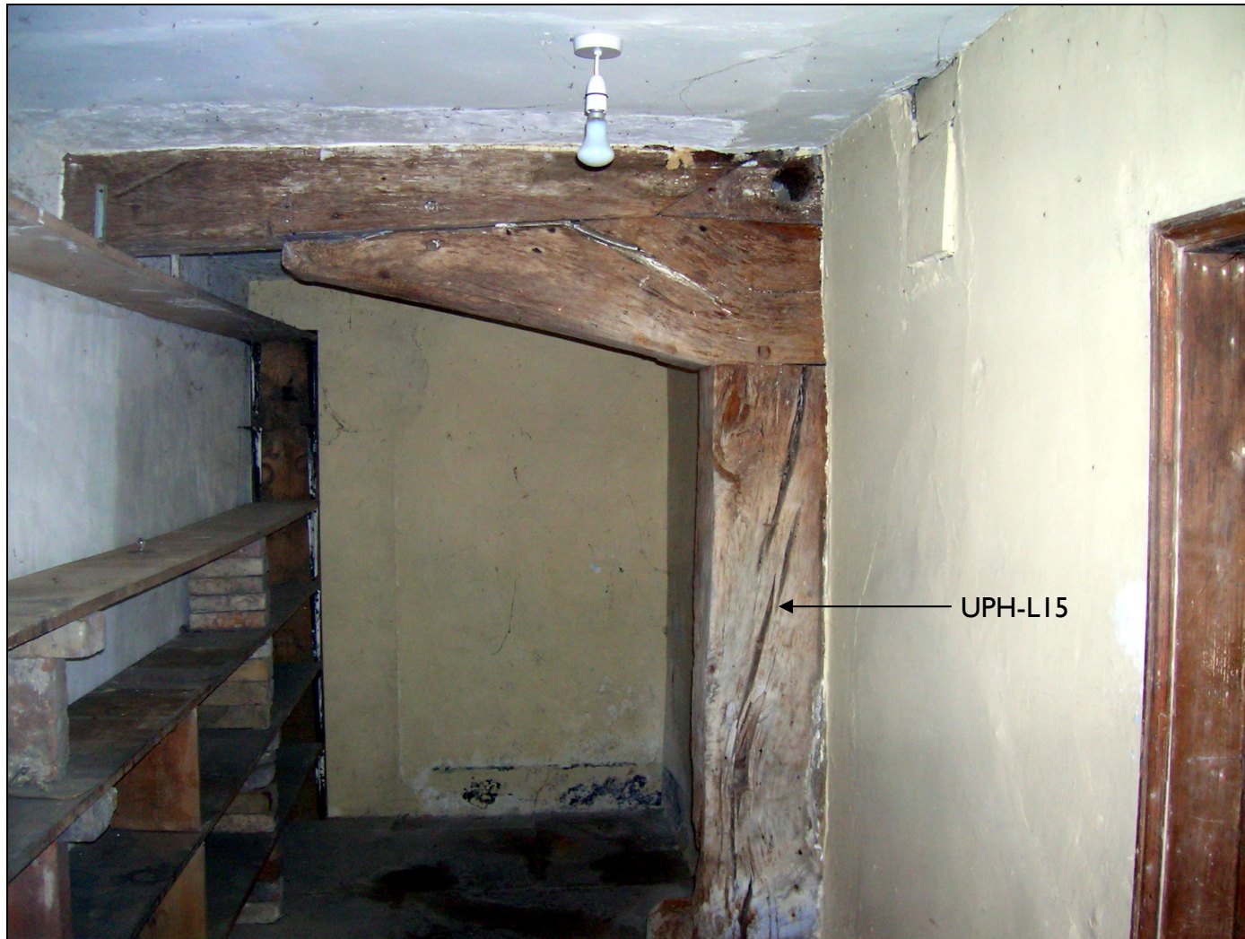
Figure 7: Solar range; floor structure, showing the location of sample UPH-L15, taken from the west
