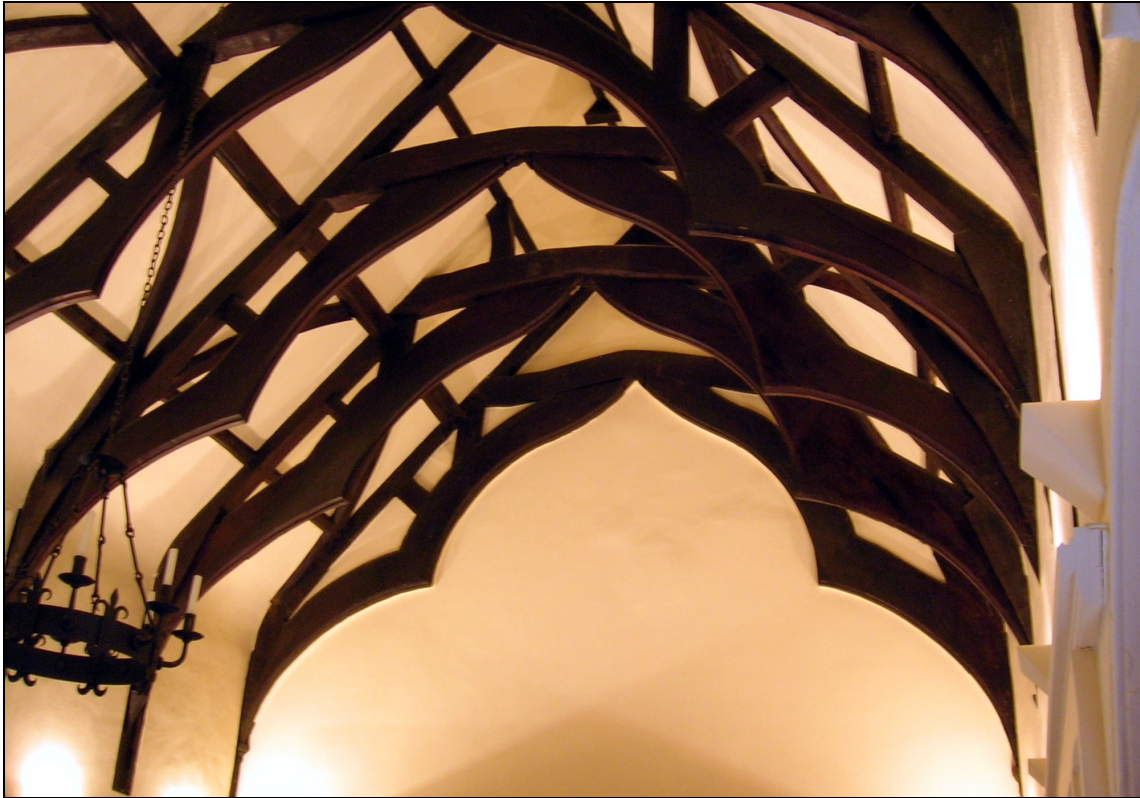
Figure 5: The Great Hall, roof, taken from the south
