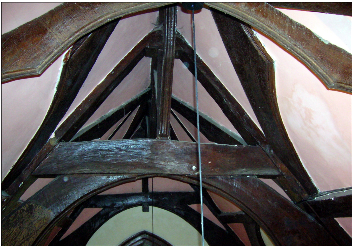
Figure 6: Uphill; the Solar roof, taken from the west
