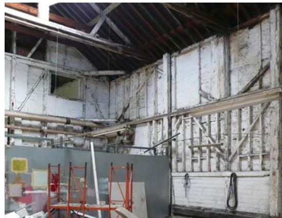
Figure 70: The late 18 th century timber-framed walls of the carpenters' shop (formerly vat house). DP070428.
