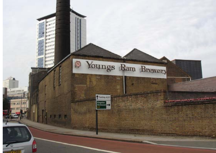
Figure 68: The double-hipped form of the cooper's shop.. DP070426.
