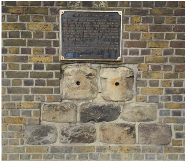
Figure 6: Stone sleepers of the Surrey Iron Railway, set into the east wall of the Ram Brewery on Ram Street. DP0703779
