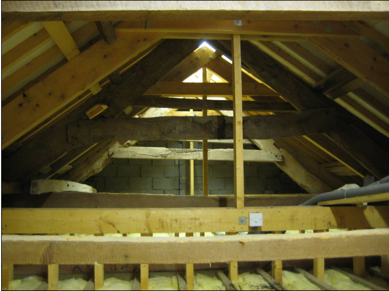
Figure 7: North range; looking east
