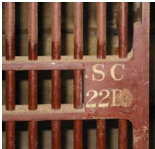
Figure 76: Detail of strong-room door, Building 2. (DP098895).
