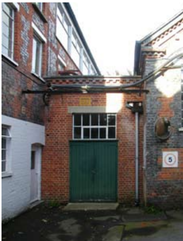
Figure 38: Building 10, south elevation (DP098886).
