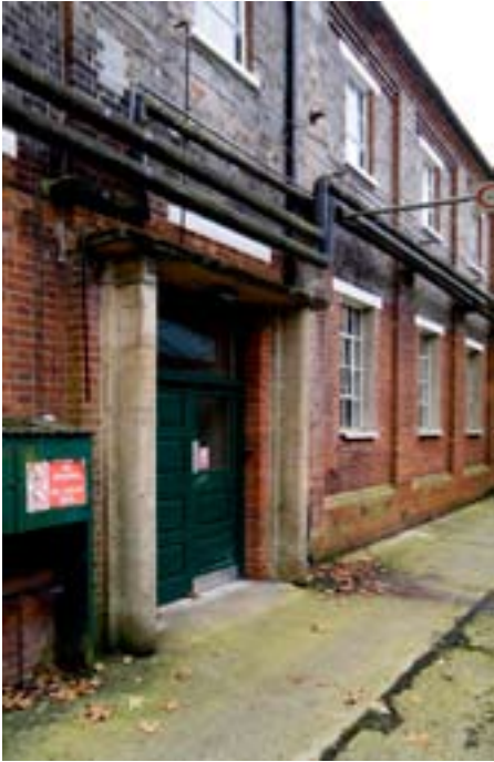
Figure 67: Building 22, north elevation (photograph: Derek Kendall; DP017525).
