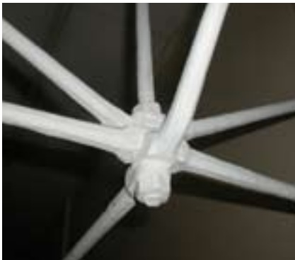
Figure 54: Building 3, detail of wrought-iron truss connectors (DP098890).
