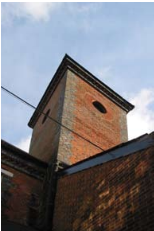
Figure 56: Building 7, watertower (DP098891).
