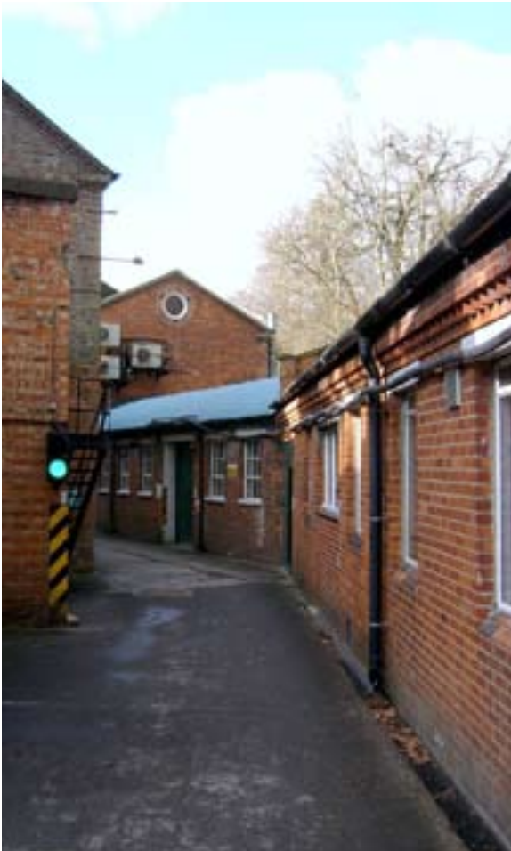
Figure 65: South elevation of Building 25 (to the right). In the background is Building 26 (photograph: Andrew Barber, B&DBC).
