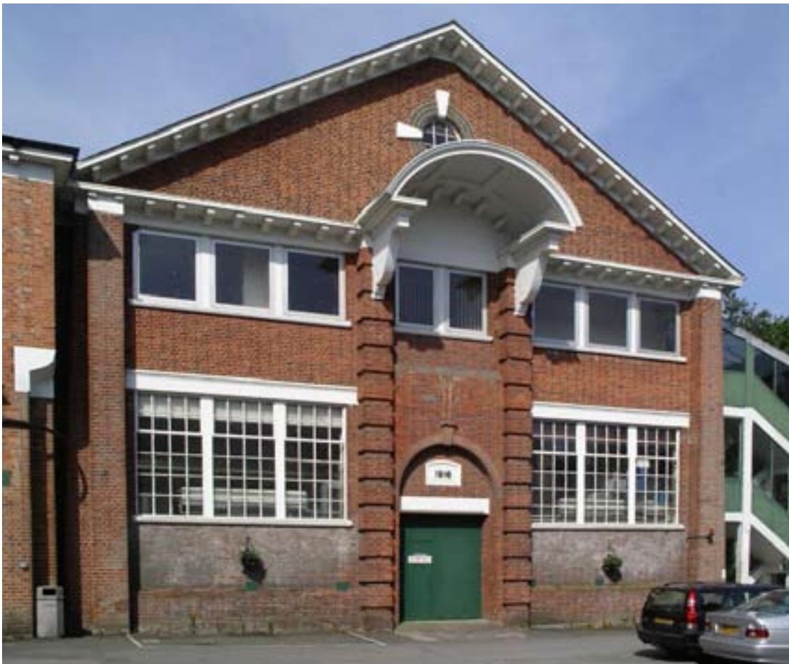
Figure 69: Building 14, east elevation (photograph: Andrew Barber, B&DBC).
