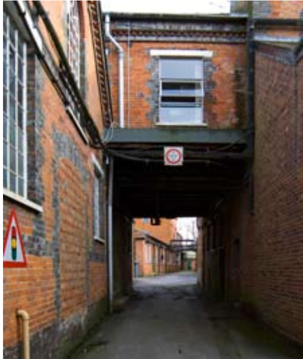
Figure 6: A Laverstoke Mill 'streetscape' (photograph: Derek Kendall; DP017476).
