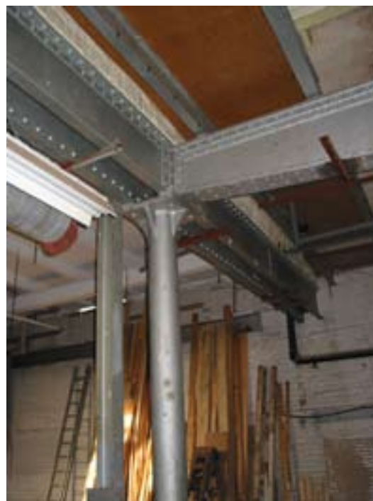
Figure 32 Building 9: fish-bellied beams (DP098884).
