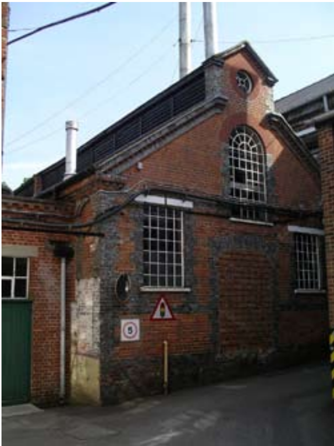
Figure 31: c.1854 element of Building 9, south elevation (photograph: Andrew Barber, B&DBC).
