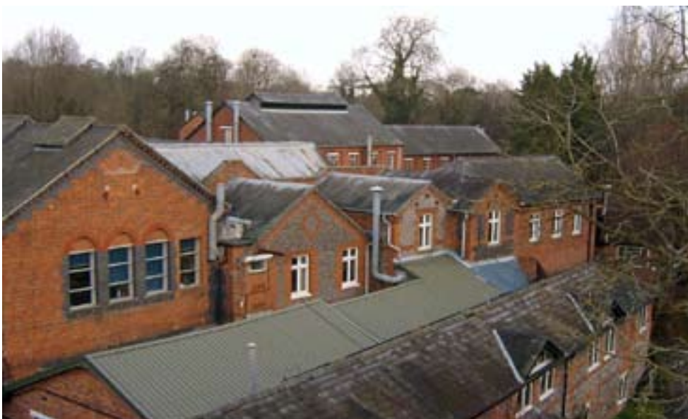
Figure 47: Building 2, south elevation. In the foreground are Buildings 19 (with metal roof and 18 (slate roof). (photograph: Andrew Barber, B&DBC).
