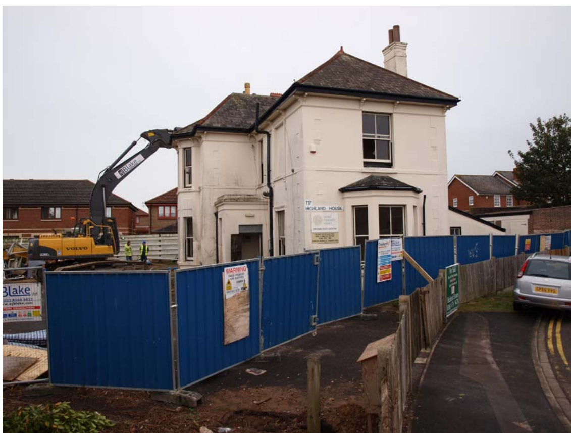
Figure 1. Highland House, 117 Lidiard Gardens, Southsea in October 2009
