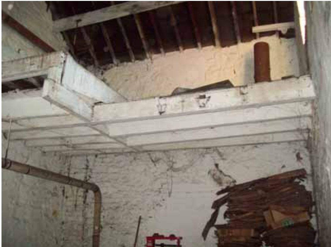
Figure 10: View of the remains of the third-floor frame of the 'tower'
