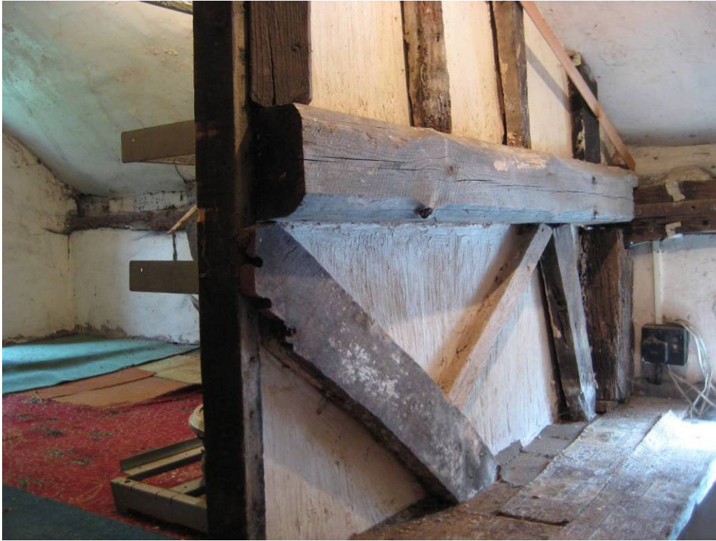
Figure 5: Stairway stud partition wall with sampled brace in the foreground viewed looking south east
