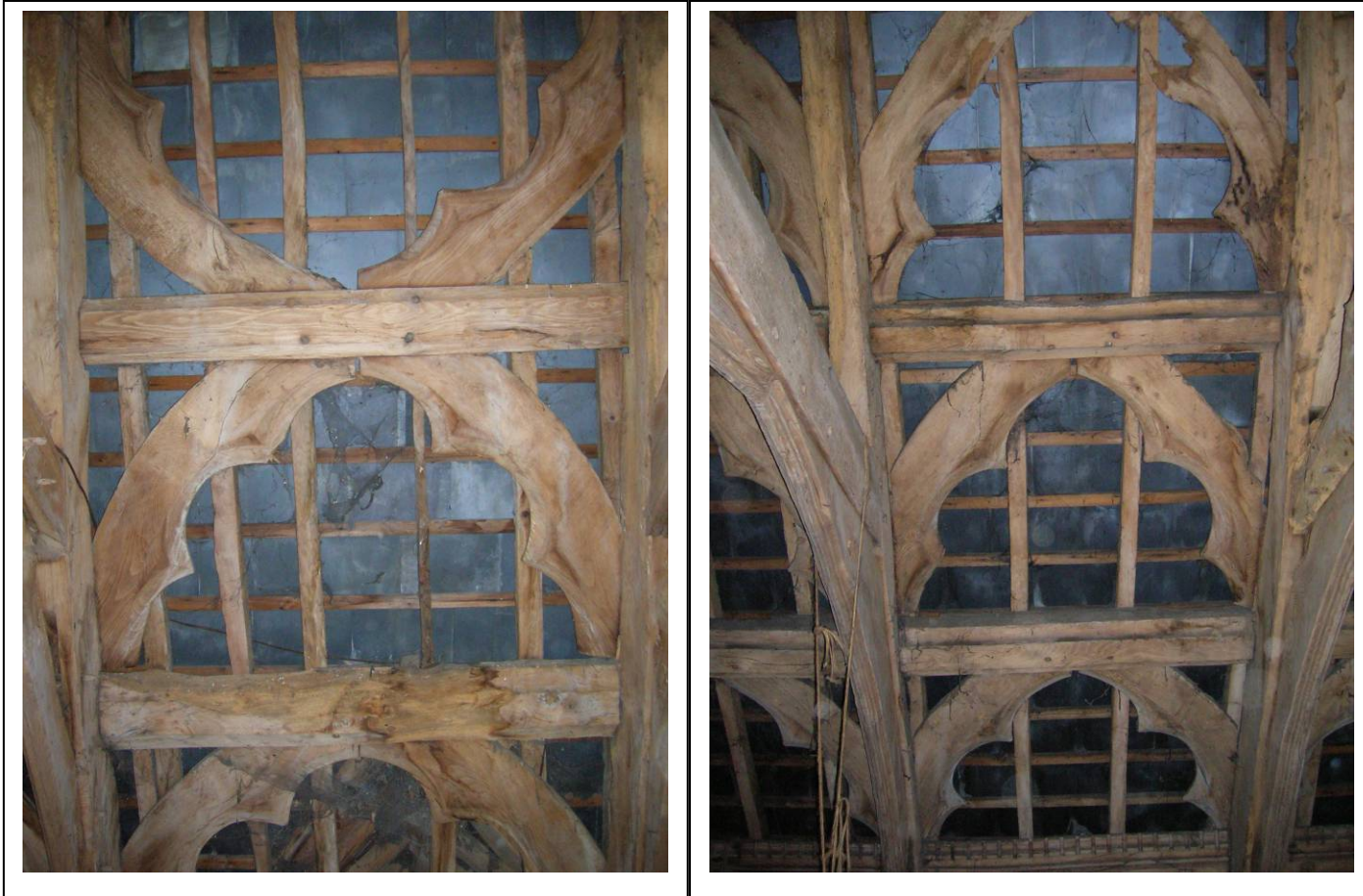
Figure 6 (left): Windbraces to the great chamber roof
