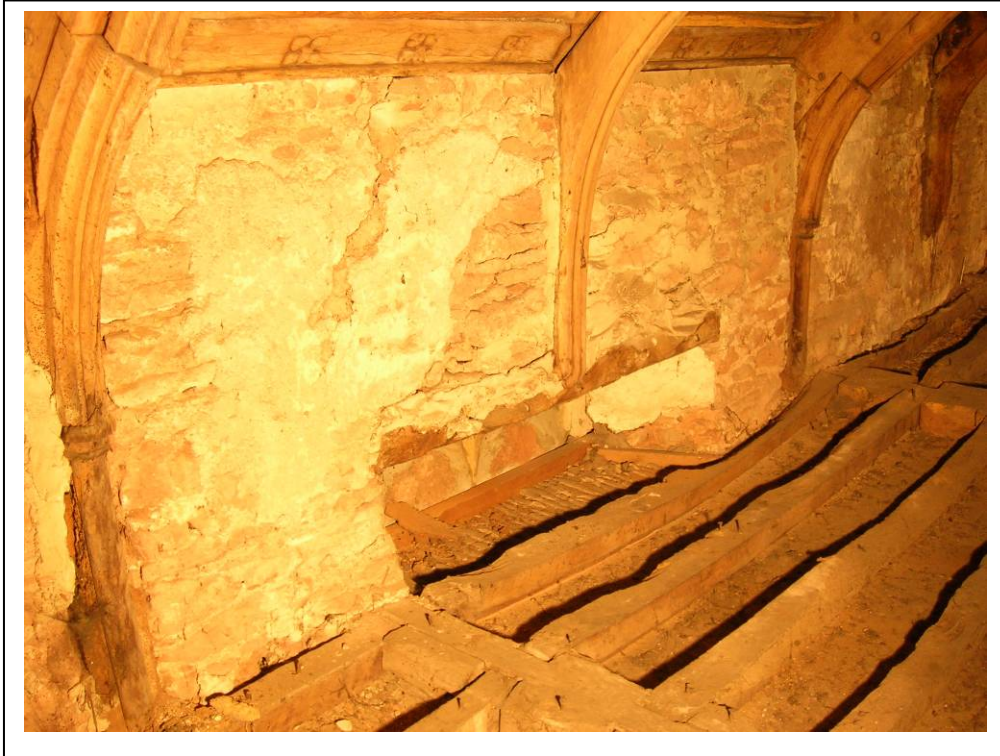
Figure 9: The attic floor frame cutting across a window of the great chamber
