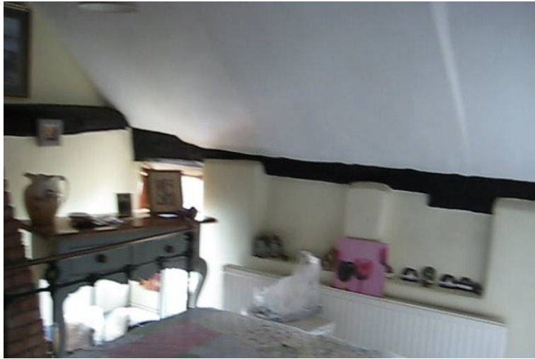
Figure 5: Bay 2 first-floor south wall plate and cross-frame 3 tiebeam, viewed looking south-east
