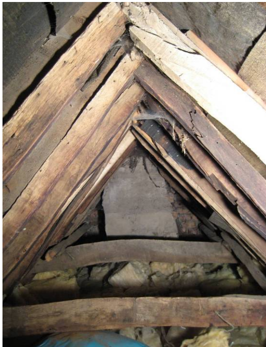
Figure 6: General view of Bay 2, viewed looking towards the east gable wall
