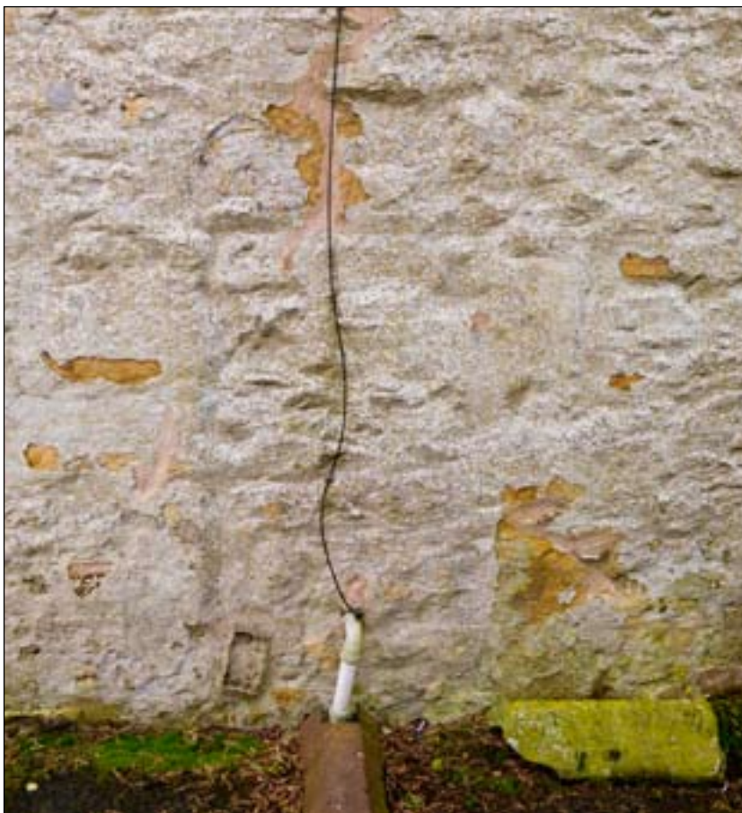
Fig. 11: the blocked byre doorway in the east gable wall of the bastle. [DP072097]
