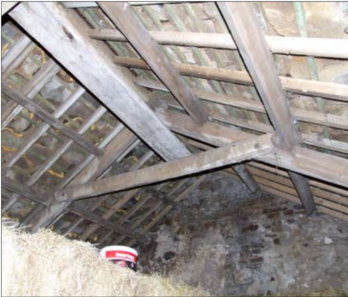
Fig. 26: View into the roofspace of the mineshop, showing one of the softwood trusses and traces of plaster on the east gable. [DPI35352]
