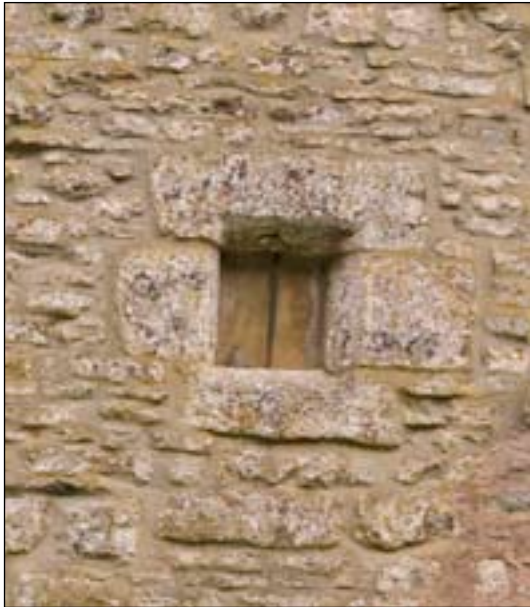
Fig. 9 : detail of the fire window on the first floor of the south elevation. [DP072082]
