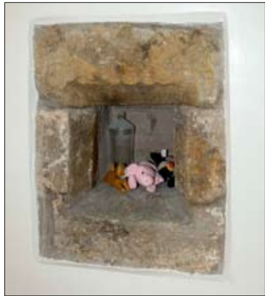
Fig. 10: detail of the chamfered window on the first floor of the north wall of the bastle, blocked when the northern addition was built. [DP072099]
