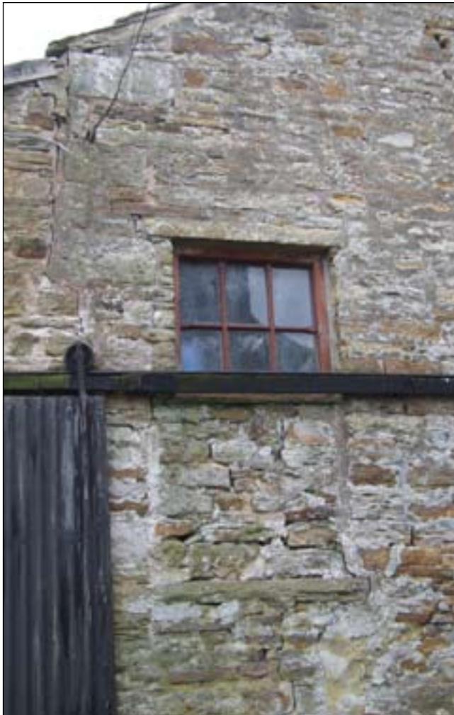
Fig. 24: The blocked first-floor doorway, now a window, in the west gable wall of the mineshop, [DPI35349]
