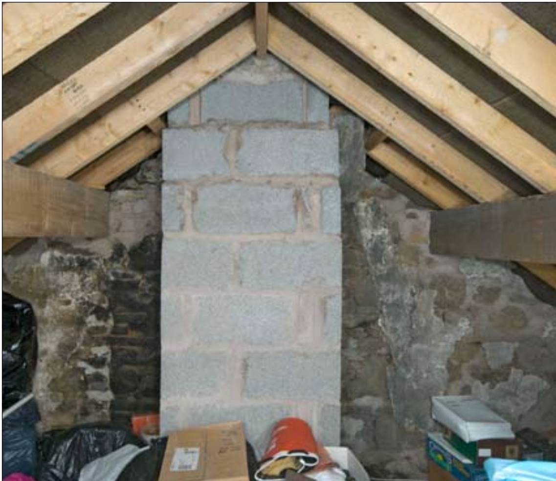
Fig. 12: view within the roof towards the west. The diagonal plaster scar to either side of the modern stack shows the form and position of the removed smoke hood. [DP072104]
