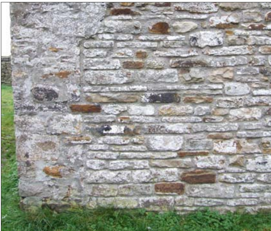
Fig. 23: The south-western corner of the mineshop, showing the straight joint denoting one of the original ground-floor doorways. [DPI35350]
