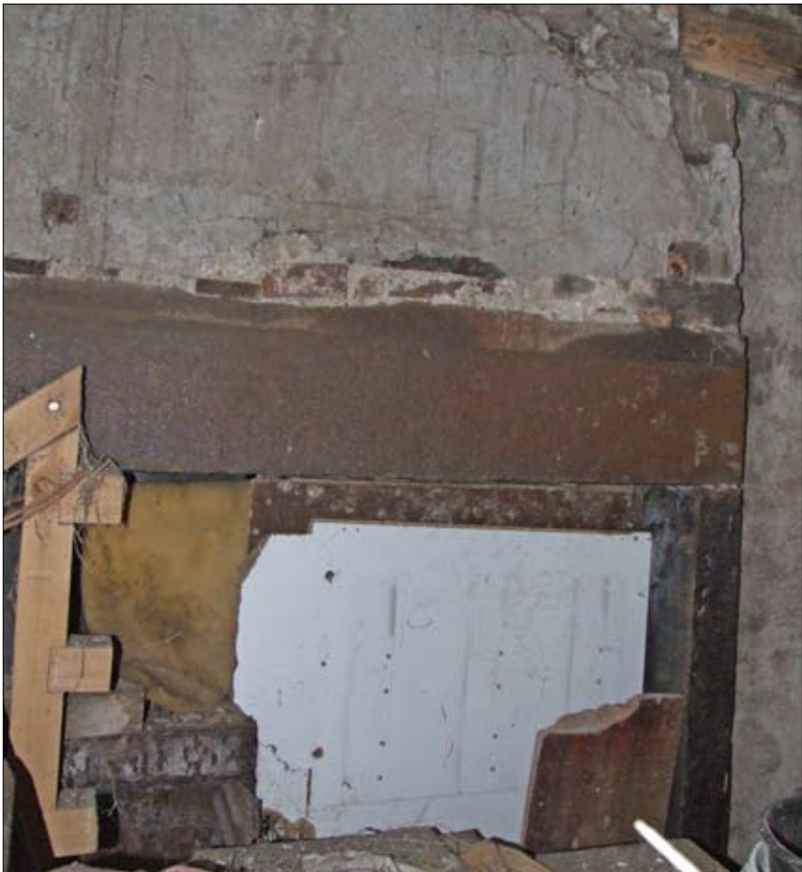
Fig. 25: The first-floor fireplace, with monolithic jambs and lintel, at the west end of the mineshop. [DPI35351]
