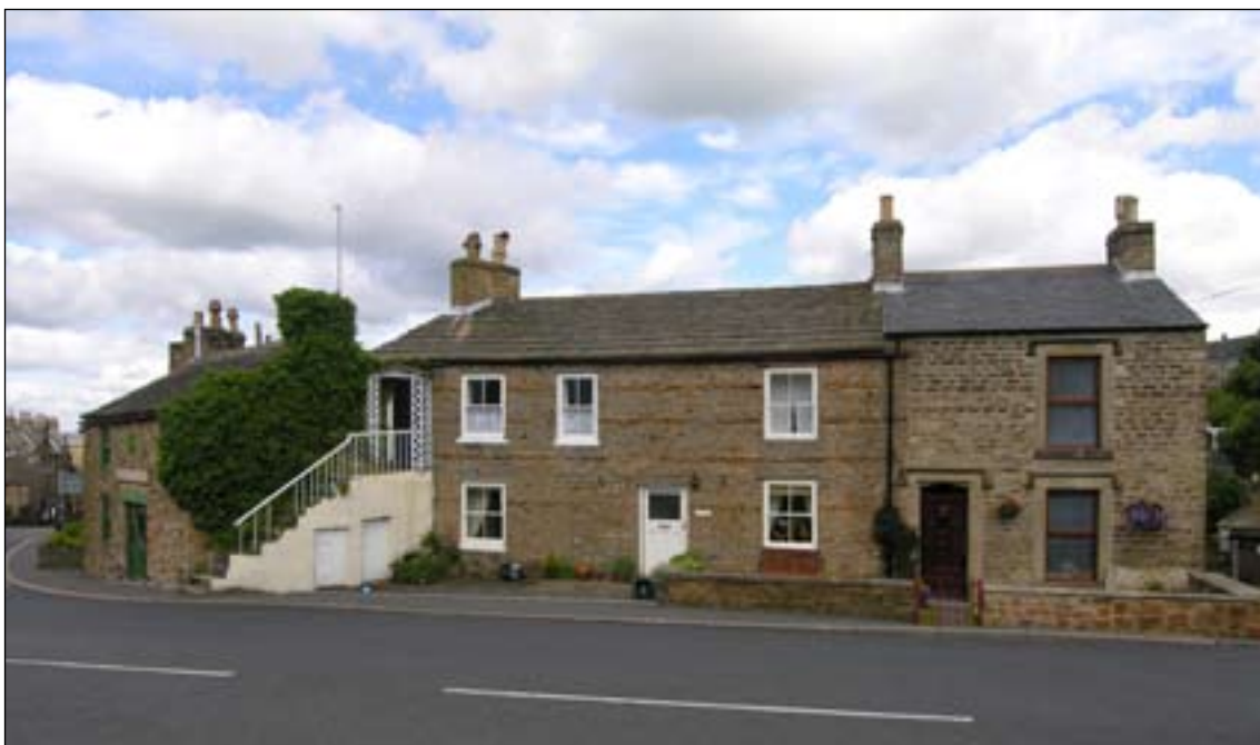
Fig. 97: Houses on Victoria Square turning into Nenthead Road: a lower density area with more open space than around the Market Place. [DPI35473]
