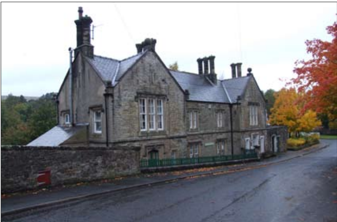
Fig. 53: The railway station, Alston, designed by Benjamin Green. [DPI35391].
