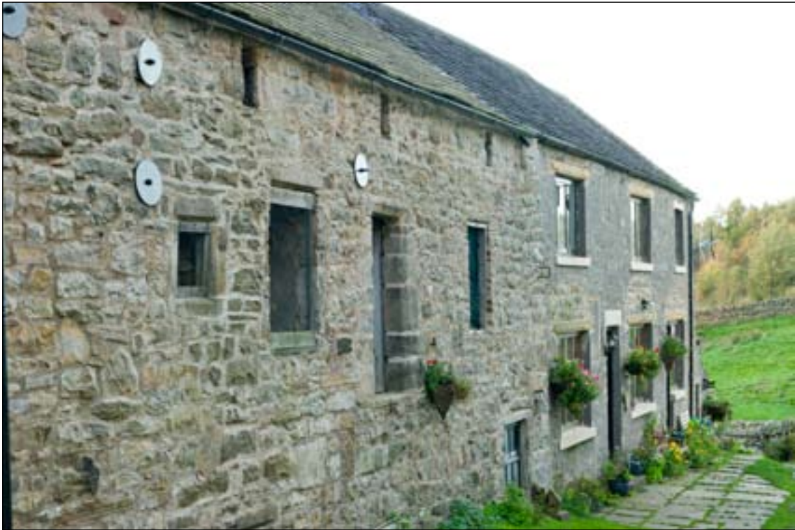
Fig. 20: the eastern elevation of the farmstead at Annat Walls [DPI09787].
