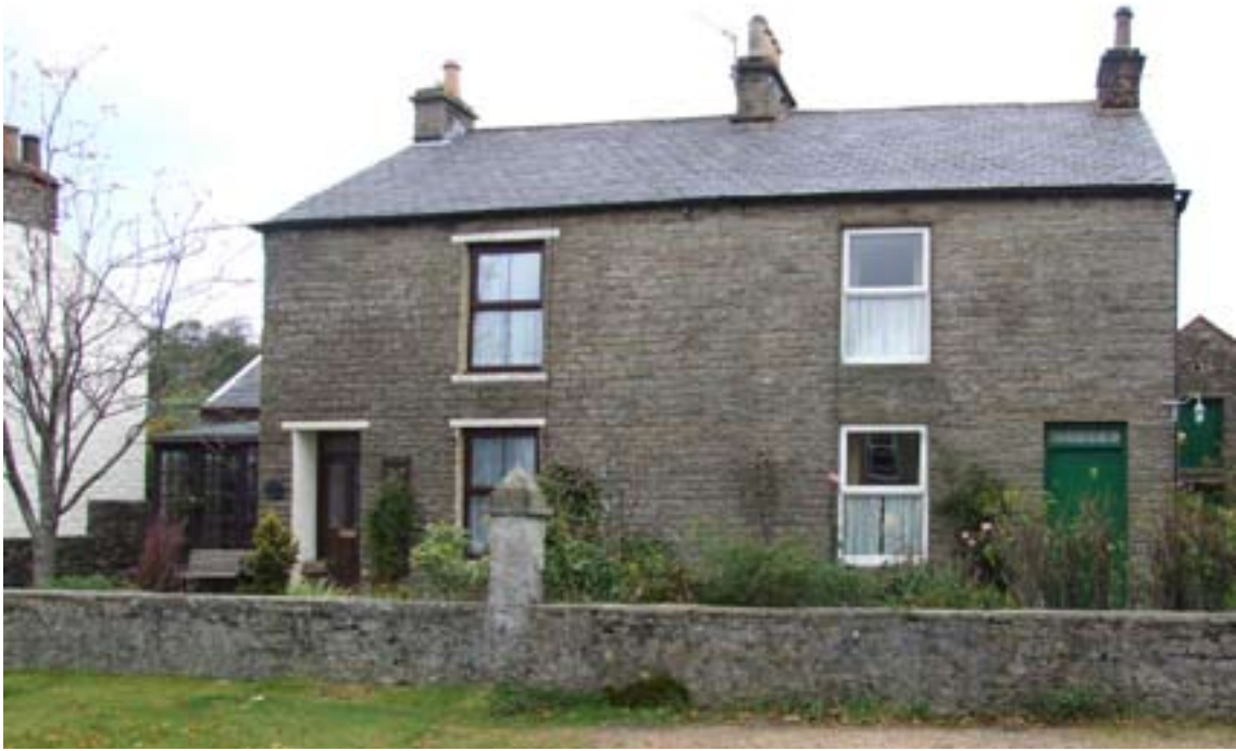
Fig. 12: Coursed rubble and Welsh slates used in this pair of mid-19th century houses, Rosedale House and Cottage, facing the Green in Garrigill. [DPI35359]
