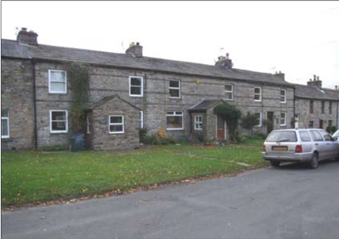
Fig. 103: Housing on the western end of the Green, Garrigill, showing coursed coloured stonework, revealing a subtle corporate influence in the village. [DPI35488]
