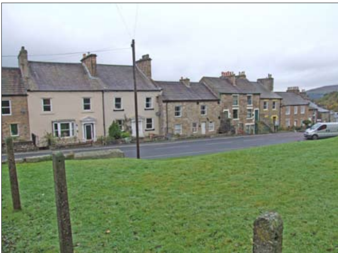
Fig. 92: Houses on the western side of Townfoot. Alston. [DPI35472]
