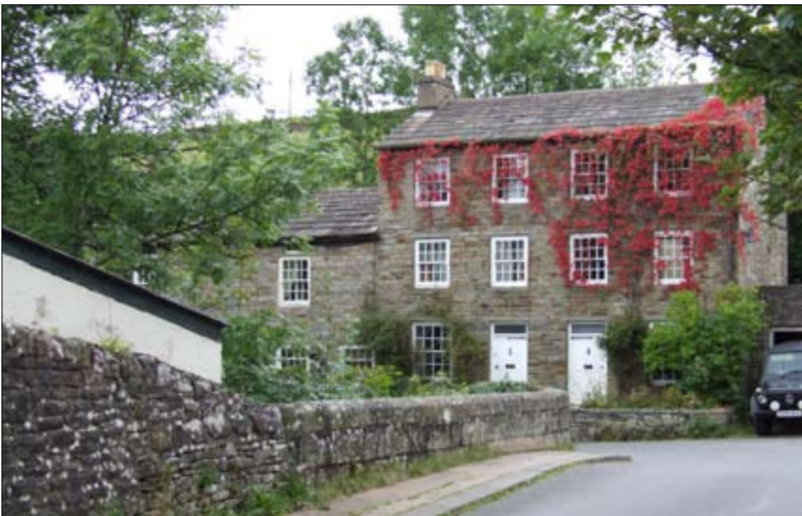
Fig. 42: Bridge House (R) and the adjacent Four Pines (L), Garrigill. [DPI35383].
