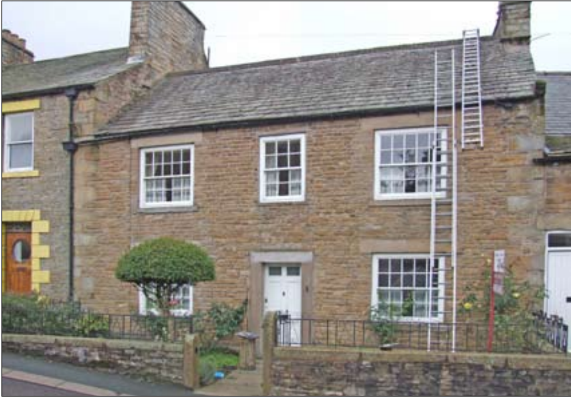
Fig. 31: Orchard House, Townfoot, Alston. The wide windows on this elevation are a later alteration, of c. 1800. [DPI35371].
