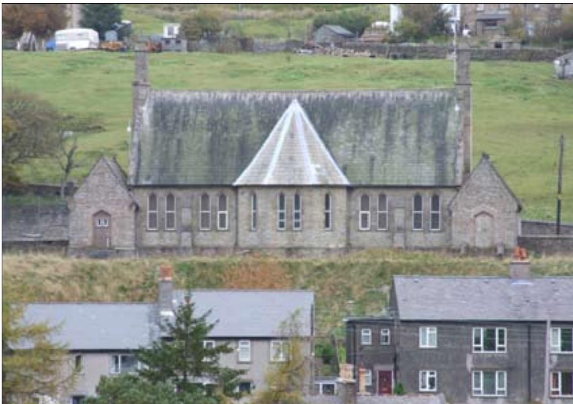
Fig. 72: Former school, now village hall, Nenthead. [DPI35409].
