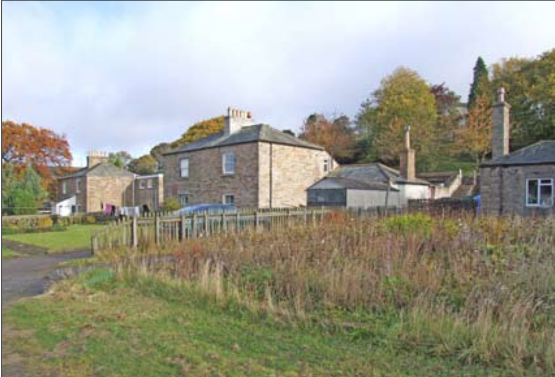
Fig. 109: Houses on Hillersdon Terrace, part of the London Lead Company's planned village development of 1825 [DPI35476].
