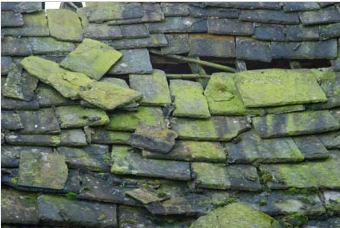
Fig. 10: Graded sandstone roof slates of the later 18th century at Middle Park, near The Raise. [DPI09731]
