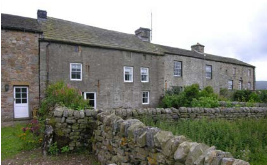
Fig. 25: Dryburn, seen from the SE. [DPI35365].
