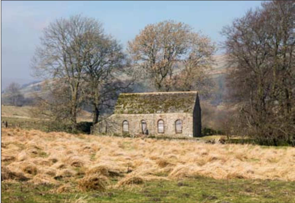
Fig. 49: Redwing Chapel, to the north of Garrigill. [DP071469].
