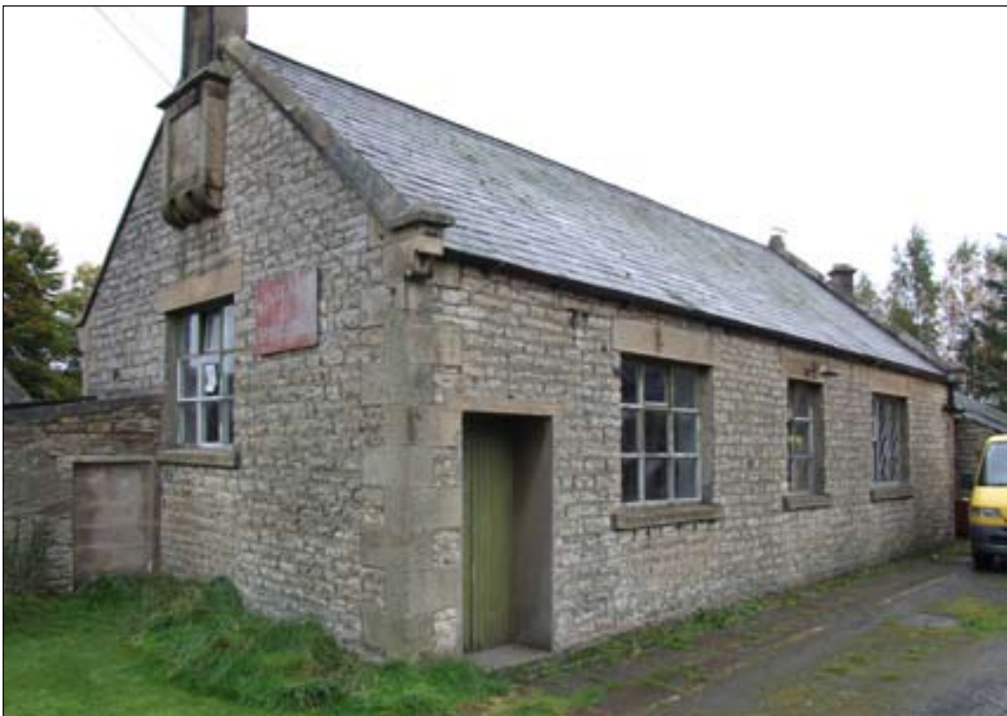
Fig. 71: Former Salvin School of 1851, King's Arms Lane, Alston. [DPI35408].
