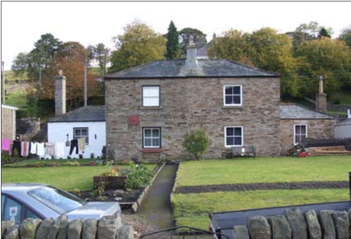
Fig. 58: A pair of overseers' semi-detached houses in Hillersdon Terrace, Nenthead. [DPI35395].
