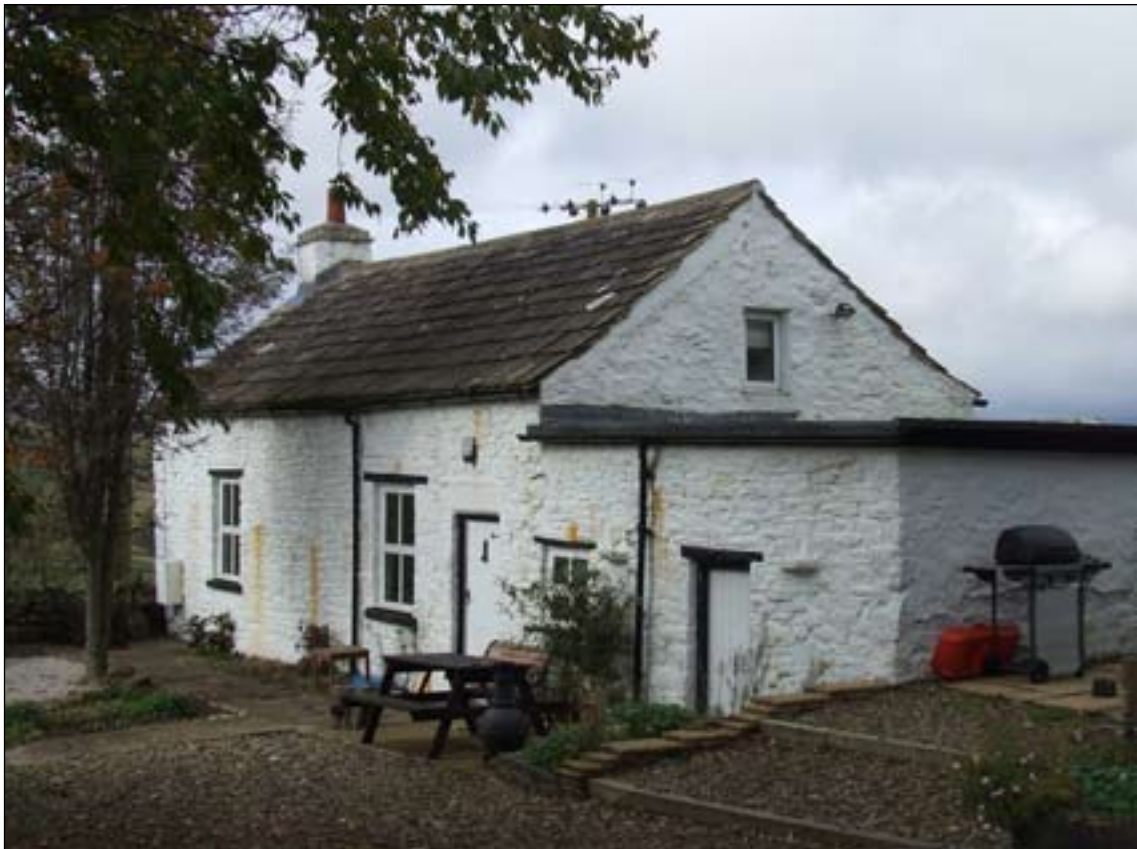
Fig. 4: The former Dissenting Chapel at Loaning Head above Garrigill, now The Cottage. [DPI35355]
