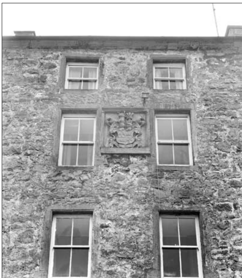
Fig. 48: Detail of the armorial carving on the tower at Randalholme. [BB99/02605]
