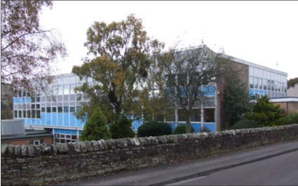
Fig. 84: Samuel King's School, Church Rd, Alston. [DPI35421].
