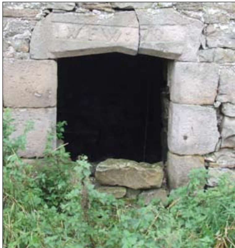
Fig. 22: the doorway, dated 1707, of the eastern of the pair of bastles near Annat Walls. [DPI35364].
