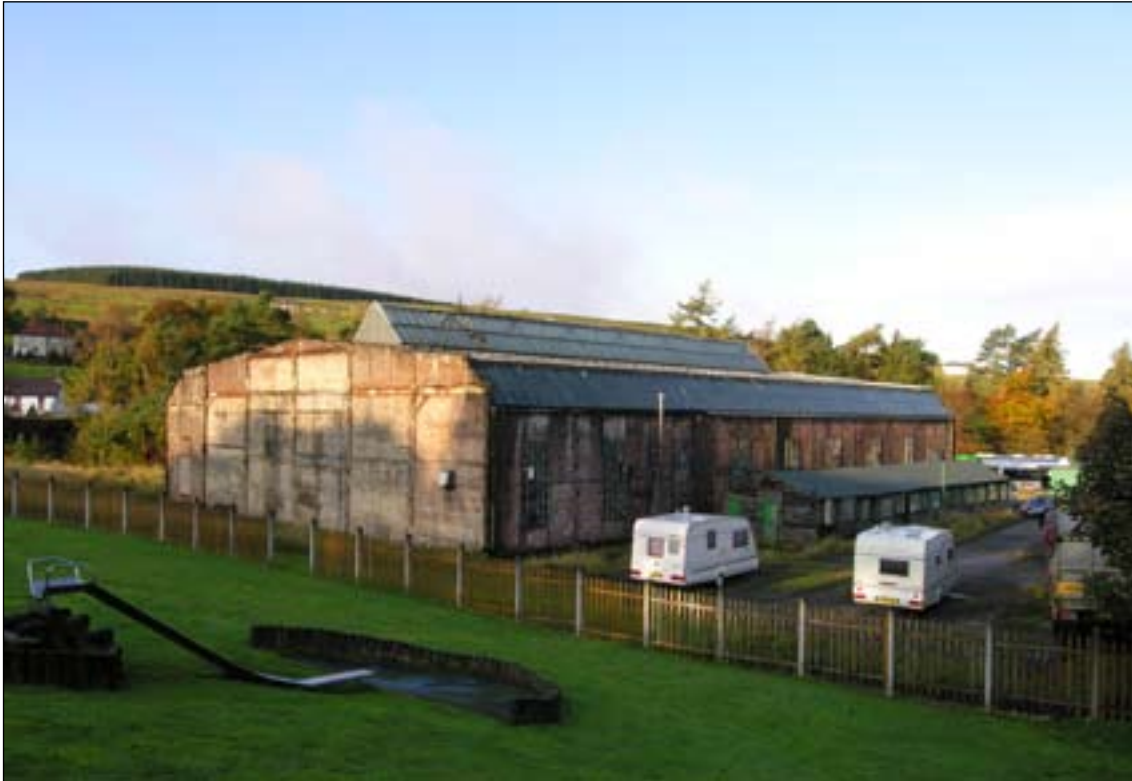
Fig. 79: The truncated remains of Vieille Montagne's former zinc ore dressing floor, now a bus garage, in Nenthead. The multi-storey gravity mill has been removed from the south end of the structure. [DPI35416].
