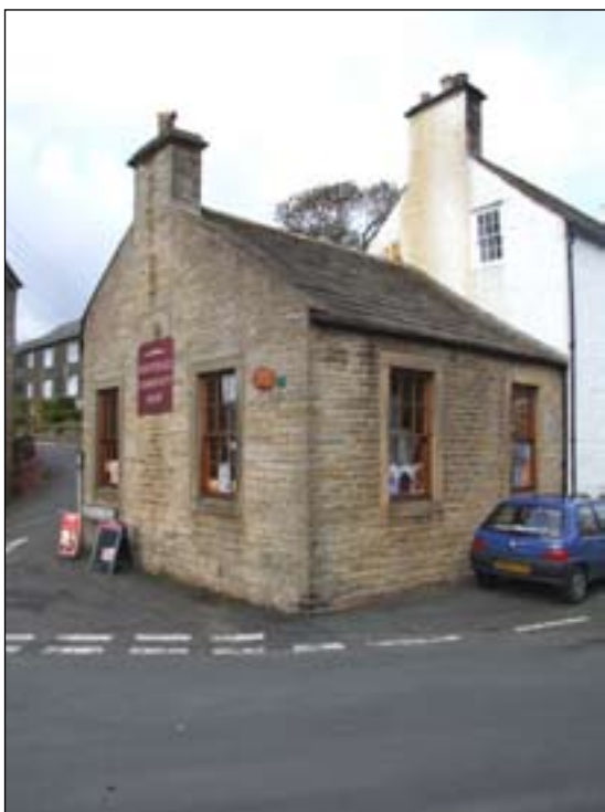
Fig. 74: Former Reading Room, now community shop, Nenthead. [DPI35411].
