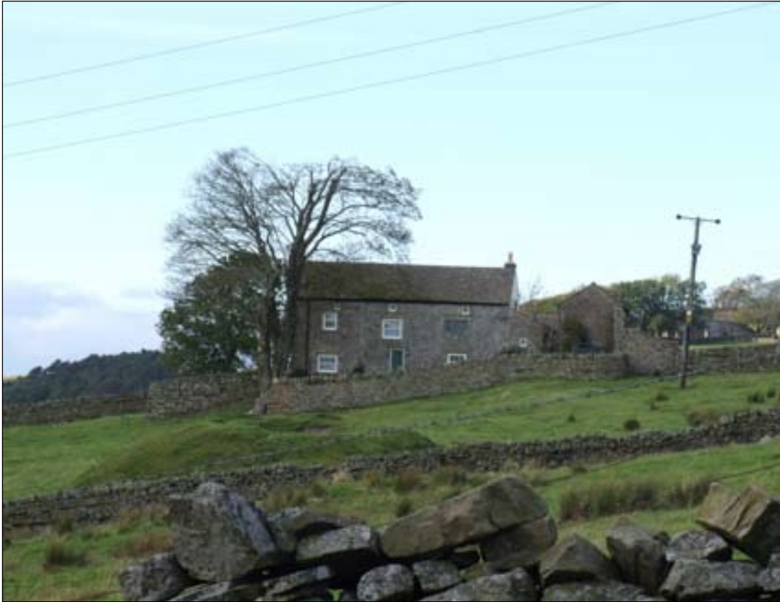
Fig. 121: Bunkershill, an example of a high-quality renovation of a bastle. [DPI35496]
