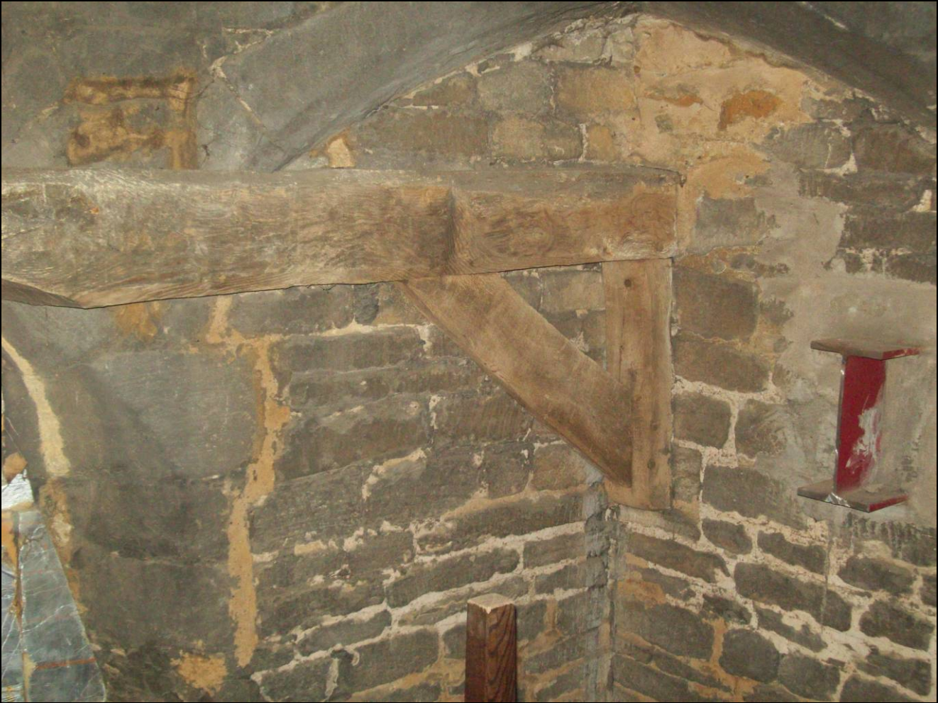
Figure 6: Upper in-situ timbers (south truss, west side)
