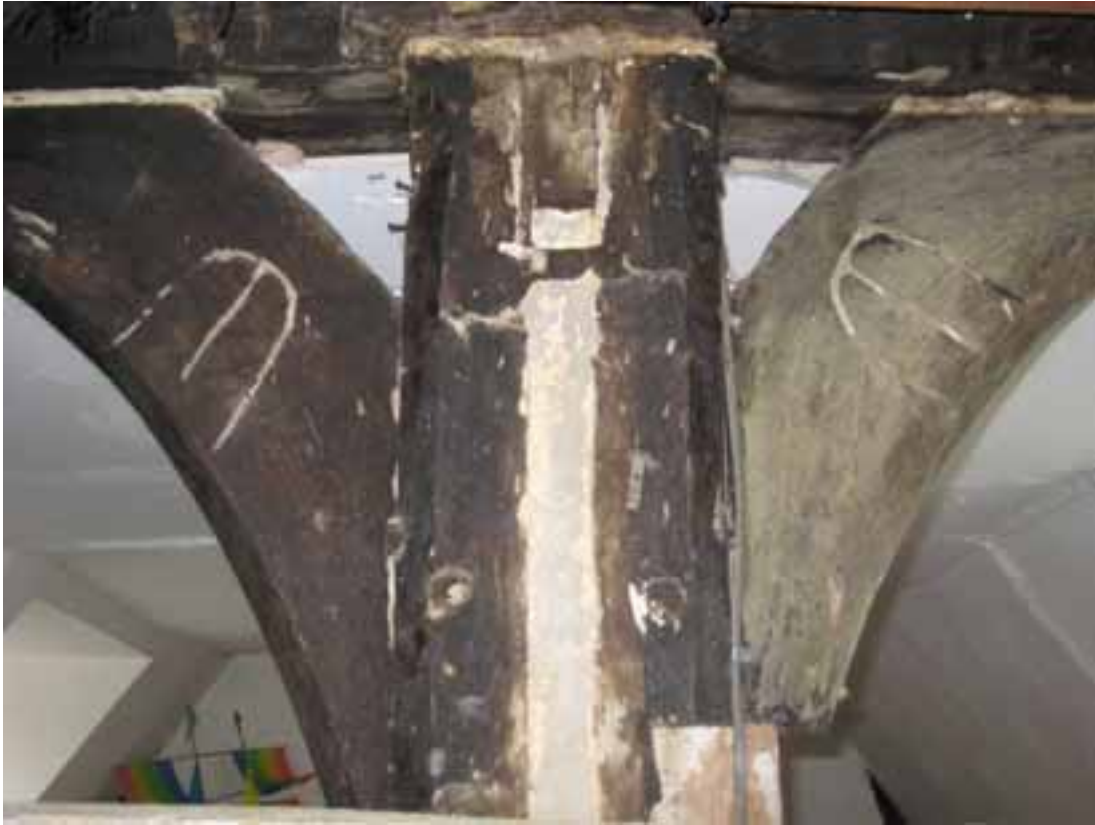
Figure 7: Detail of the Arabic assembly marks on the west face of the upward braces from the Truss B crown post to the upper crucks viewed looking east
