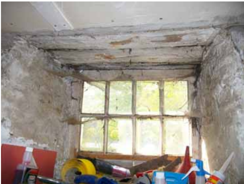
Figure 5a/b: Cruck truss (top) and window lintels (bottom) to the 'museum wing'
