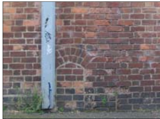
Figure 35 A blocked opening in the northern wall of block G. Hannah Waugh.
