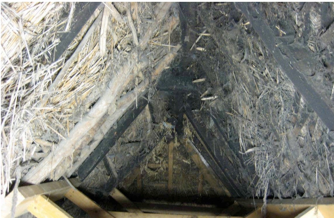
Figure 6: General view of the roof viewed looking west
