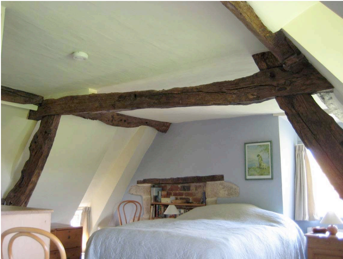
Figure 5: The east face of truss B viewed on the first floor
