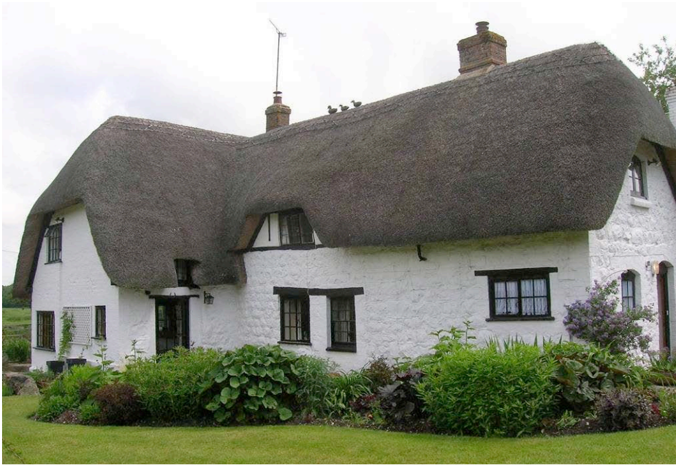
Figure 3: Castle Cottage, west elevation
