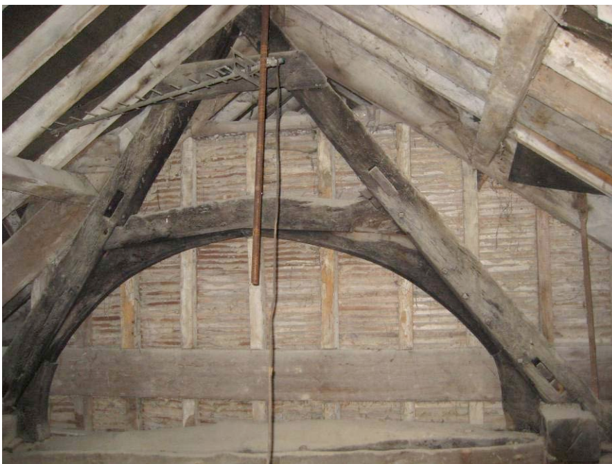
Figure 4: South face of open hall truss A
