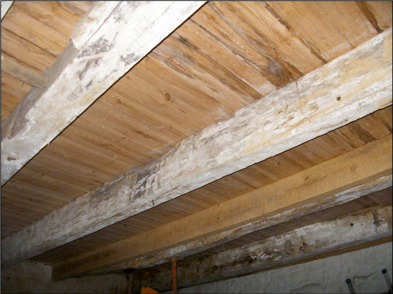
Figure 8: East range; ceiling beams (photograph taken from the north)
