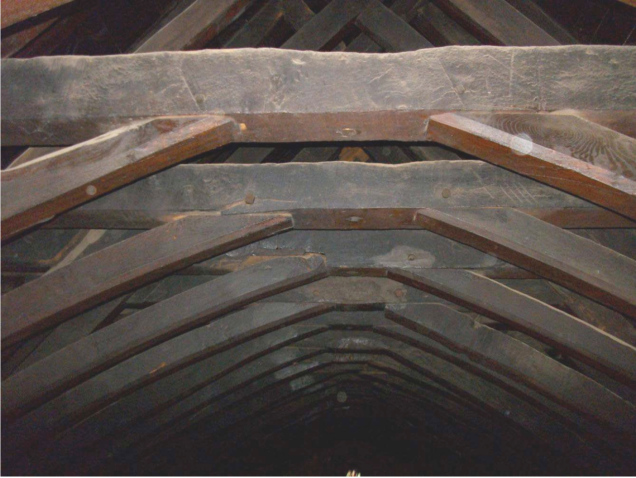
Figure 4: Photograph taken of roof, collar down
