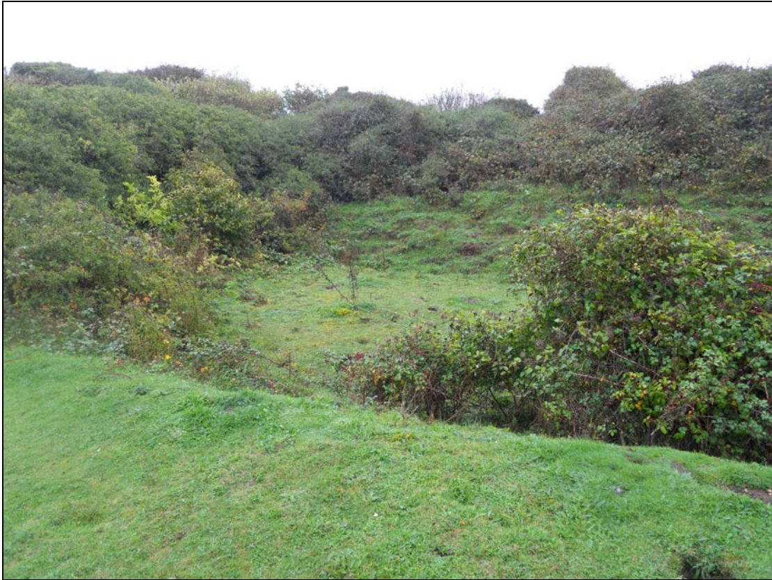
Fig 11: The deep building cut for the drying room associated with the battalion unit based around parade ground 10. Author's photograph.
