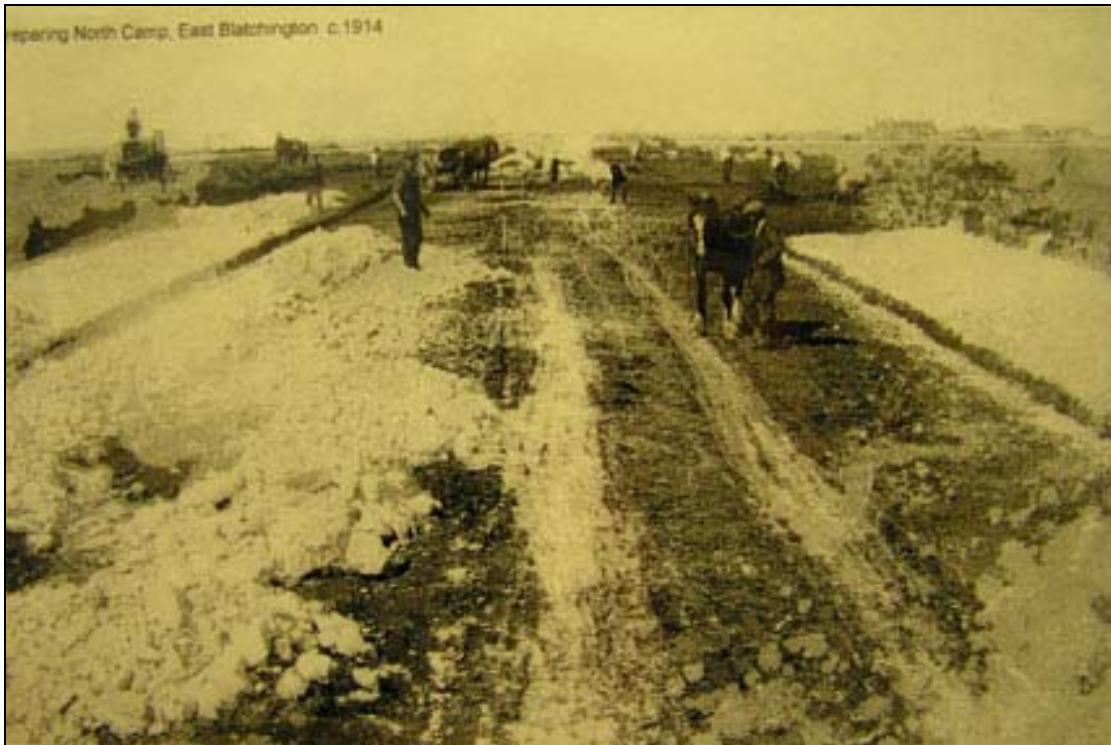
Fig 16: Postcard showing the laying down of a chalk road surface. Reproduced by courtesy of Luke Barber.
