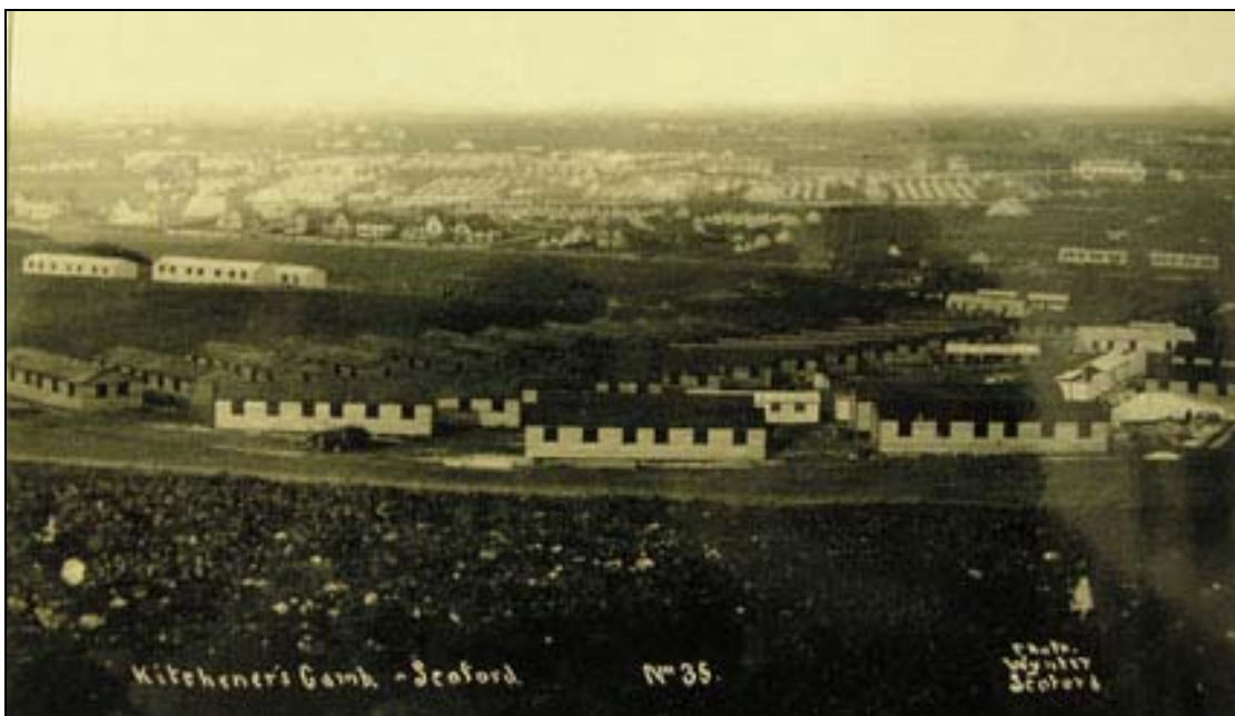
Fig 13: Postcard of South Camp with construction work in the foreground and a large tented area in the background. Reproduced by courtesy of Seaford Museum and Heritage Society.
