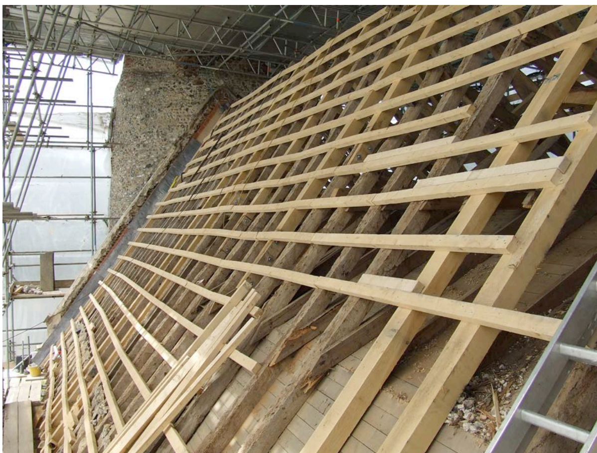
Figure 3. Photograph of the south side of the nave roof at the time of sampling, showing the small scantling of the rafters and braces
