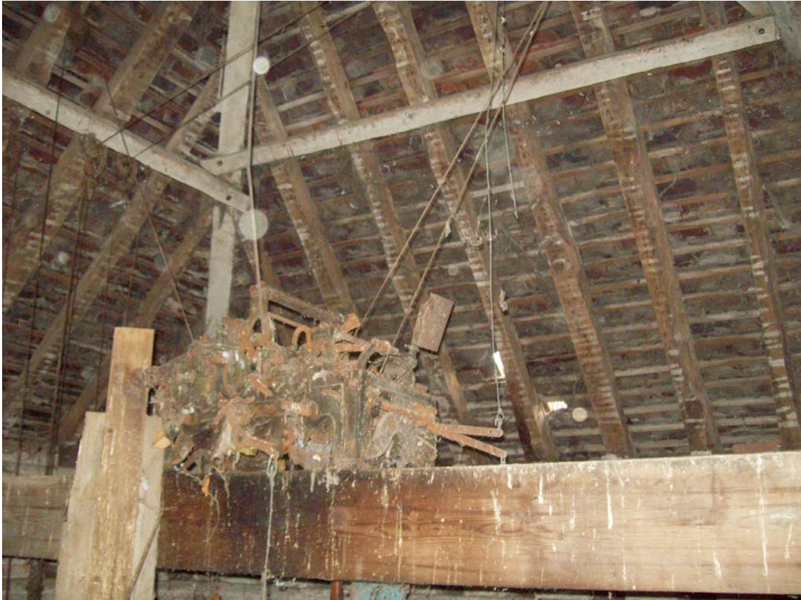
Figure 3: The dovecote roof viewed from the south-east
