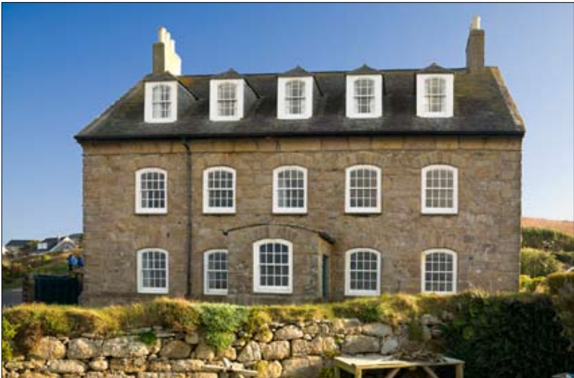
Figure 21. The Storehouse designed by Christian Lilly, now Newman House [DP116095]
