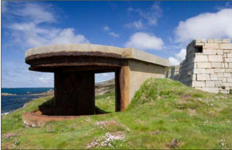
Figure 43. Defence Electric Light Position in front of the 1740s Woolpack Battery [DP022476]
