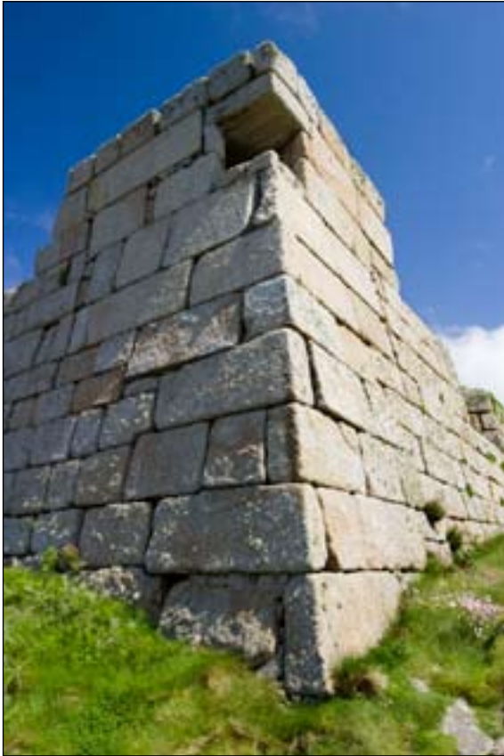
Figure 46. World War II pillbox set into tip of 18th century Woolpack Battery [DP022480]
