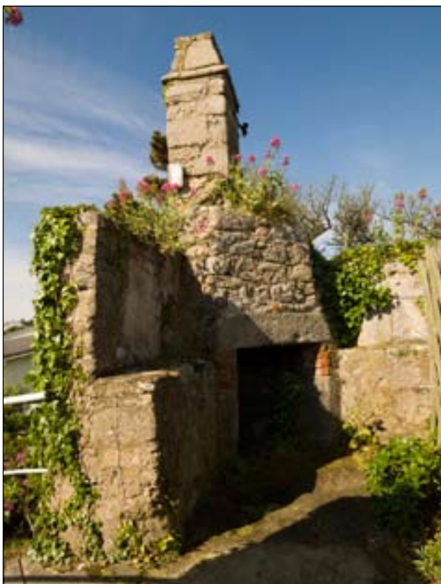
Figure 11. Small Barrack Block (unrestored) on ramparts of Star Castle [DP085306]
