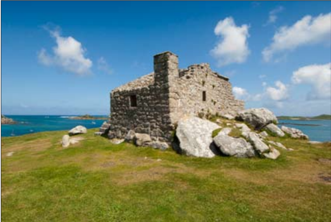
Figure 3. The Old Blockhouse, Tresco [DP085145]
