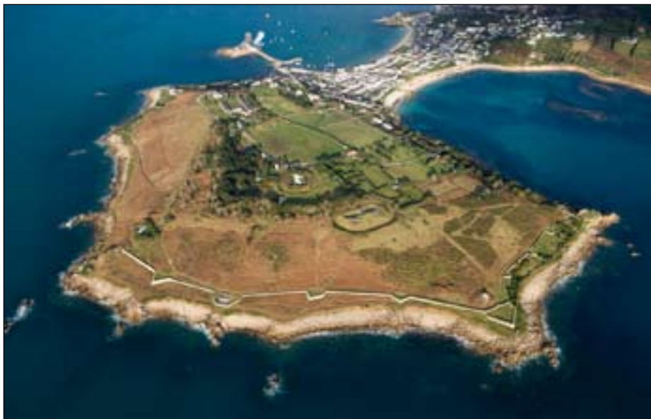
Figure 24. The Garrison with the walls of the 1740s in the foreground [NMR 26571/28]
