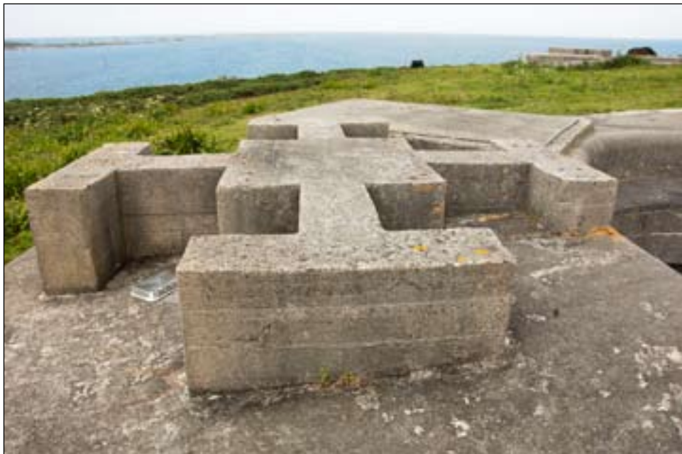
Figure 47. 'RACON' Beacon location on Woolpack Battery [DP085199]
