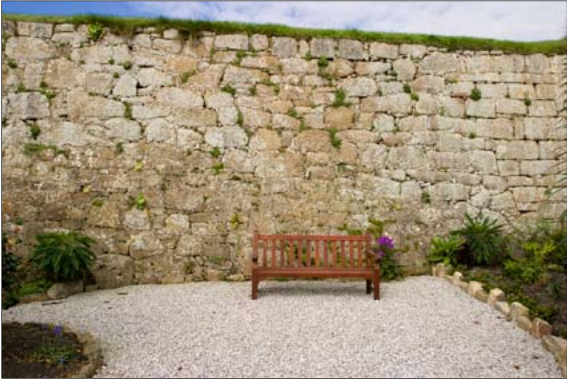
Figure 13. Wall to south of Garrison Gate [DP022358]
