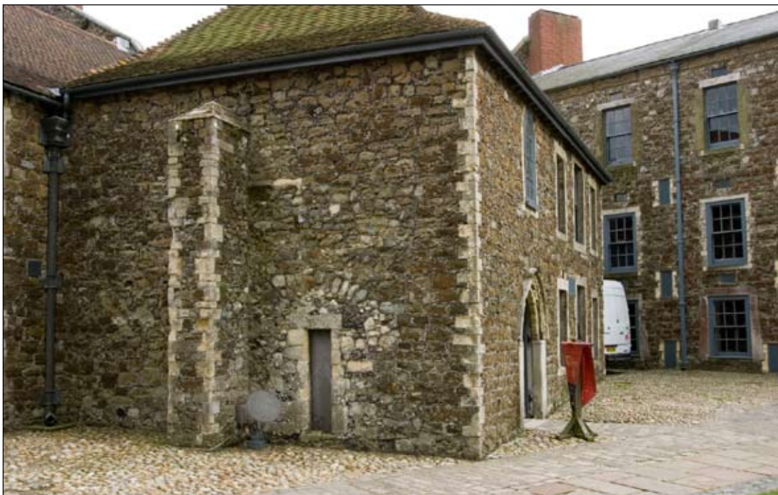
Figure 15. North-west wall of AV Building showing 'buttress' and remains of blocked arch into porch set in medieval walling with more regular, 18th-century fabric above
