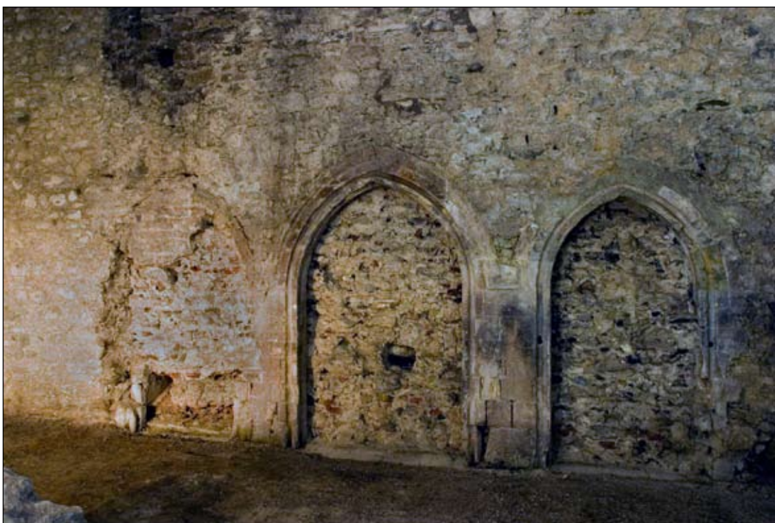
Figure 8. Service doorways at lower end of hall
