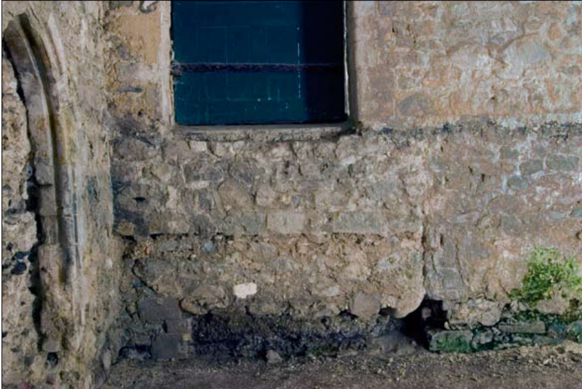
Figure 10. Joints marking site of 13th-century doorway
