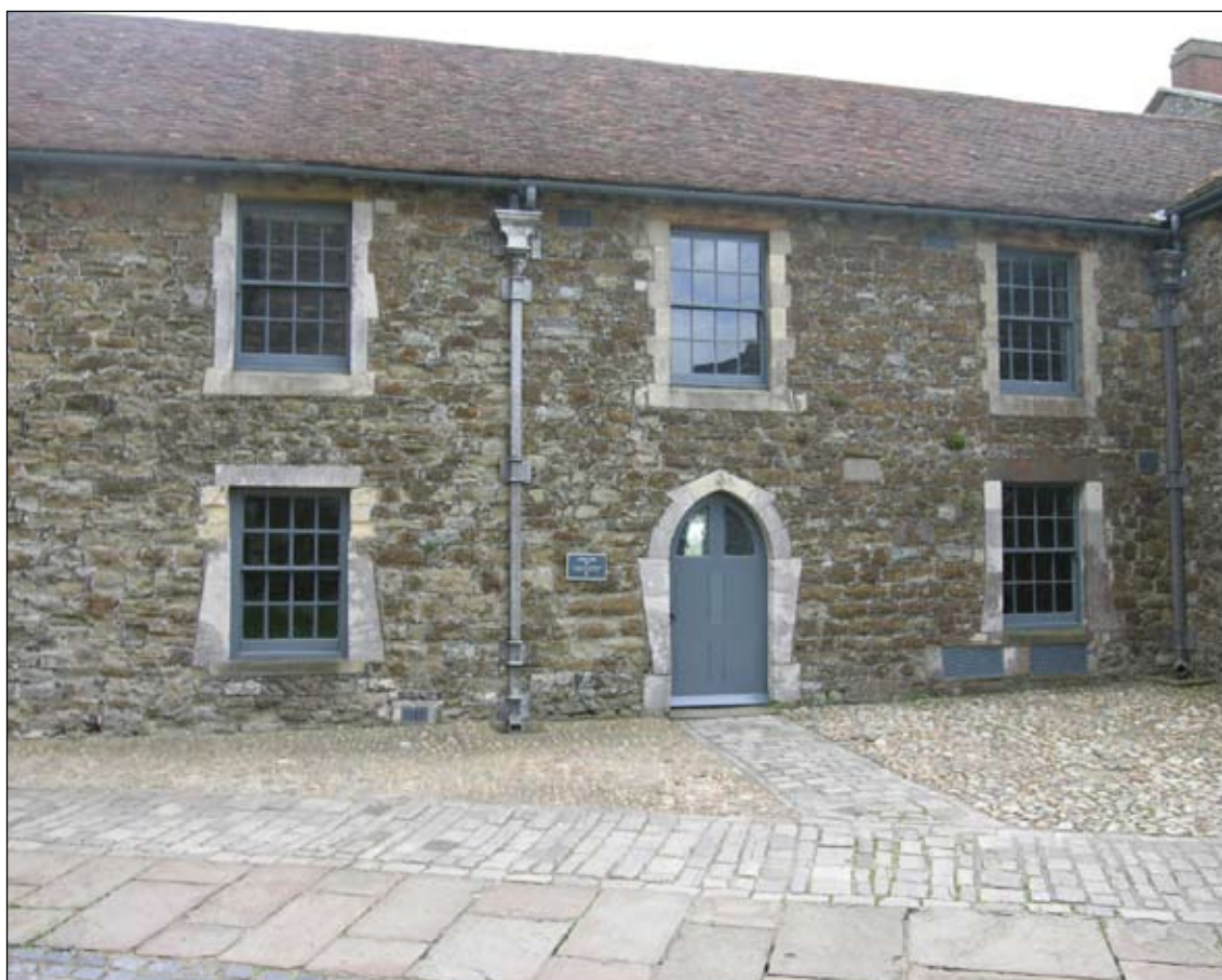
Figure 24. External face of south-west wall of Arthur's Hall. Coursed fabric to right, rubble to left
