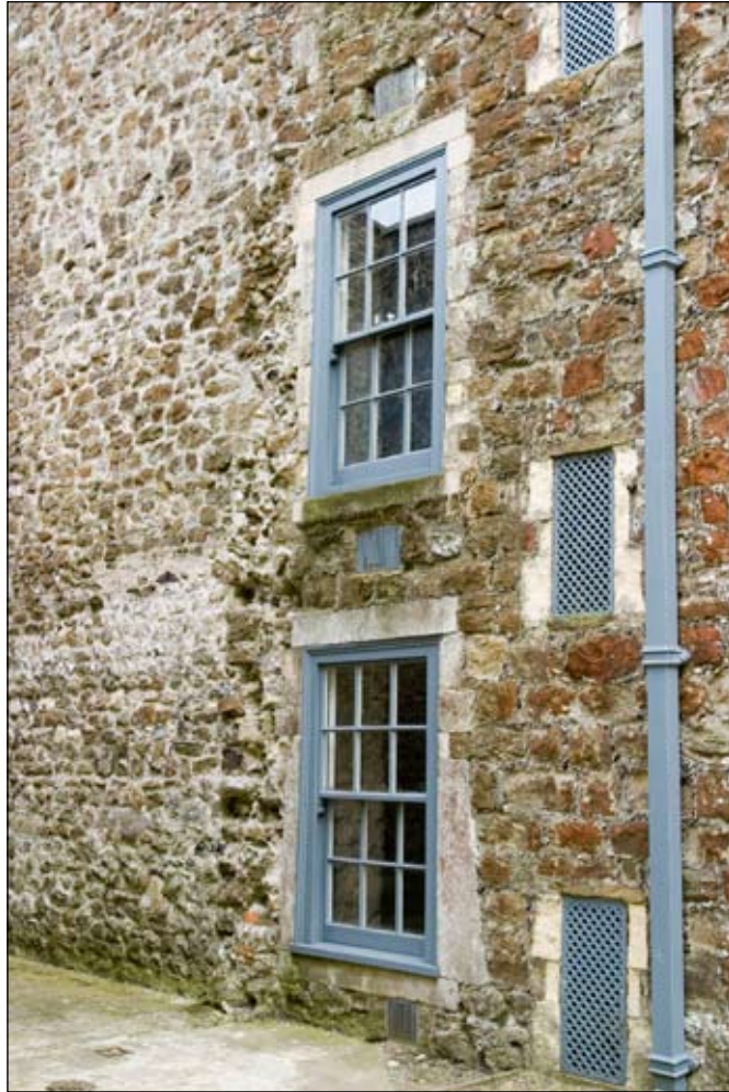
Figure 12. Vertical scar of former front wall of building, in south east corner of Inner Bailey
