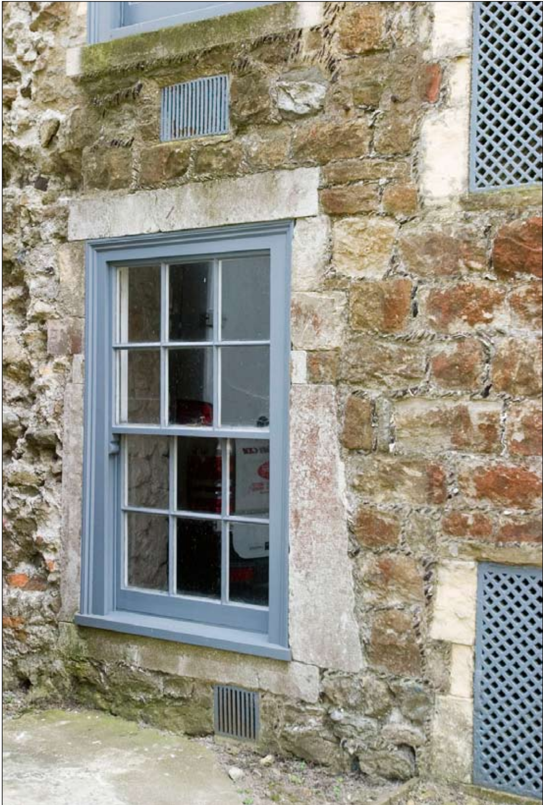
Figure 21. Window in Keep Yard 7
