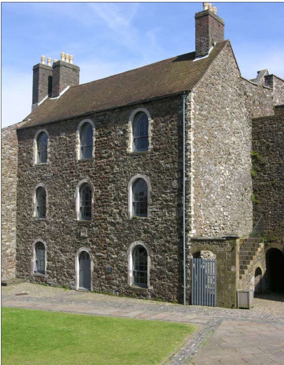
Figure 7. Keep Yard 8. Building on site of Old Armoury
