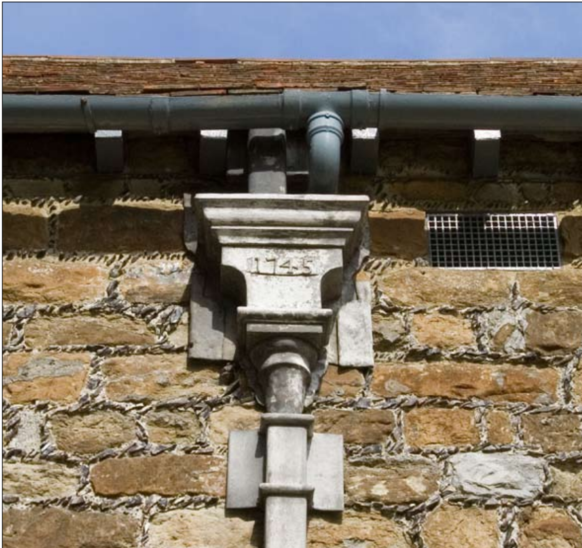
Figure 16. Rainwater head on Arthur's Hall
