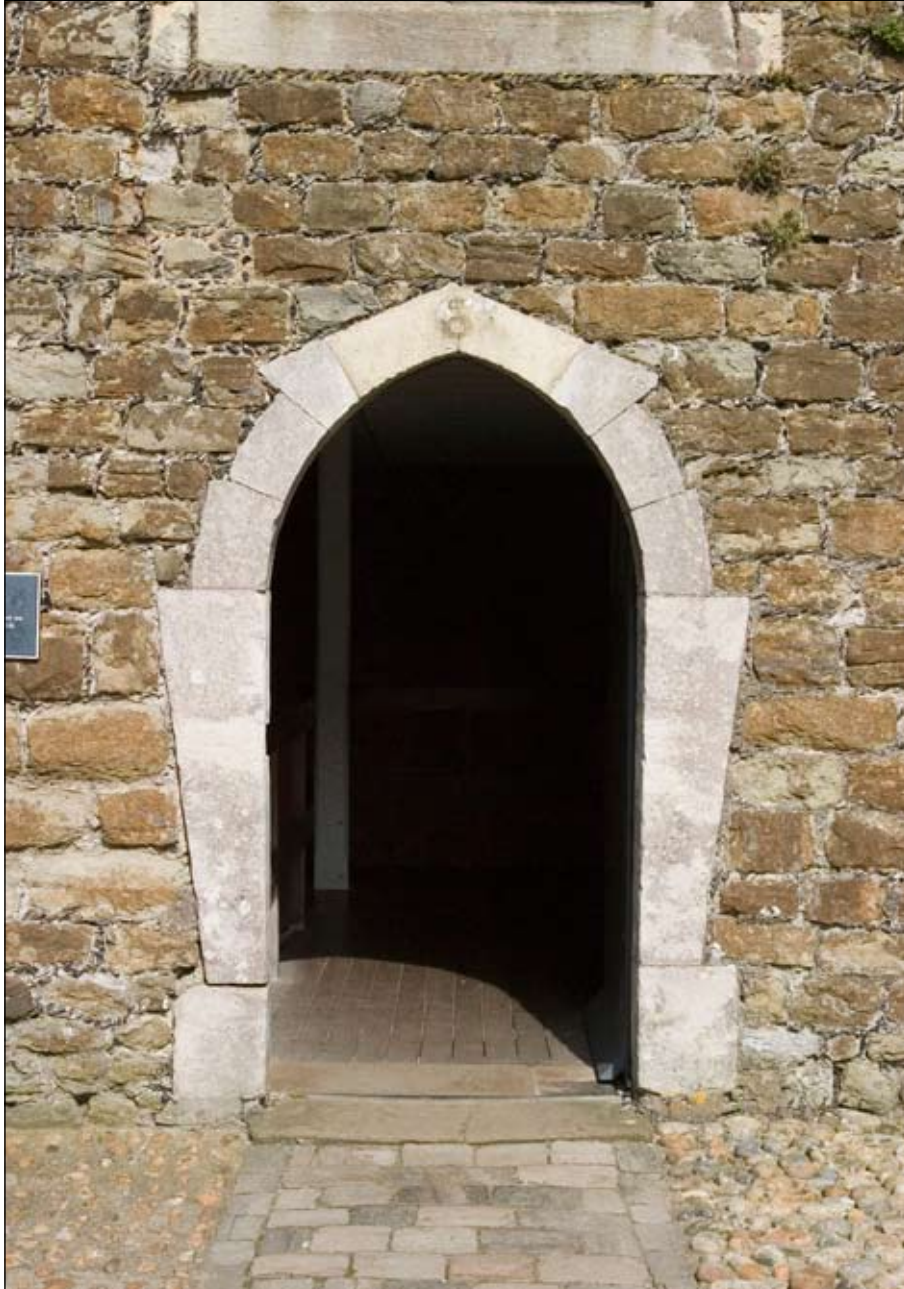
Figure 22. Door into Arthur's Hall, with reused stones in the jambs
