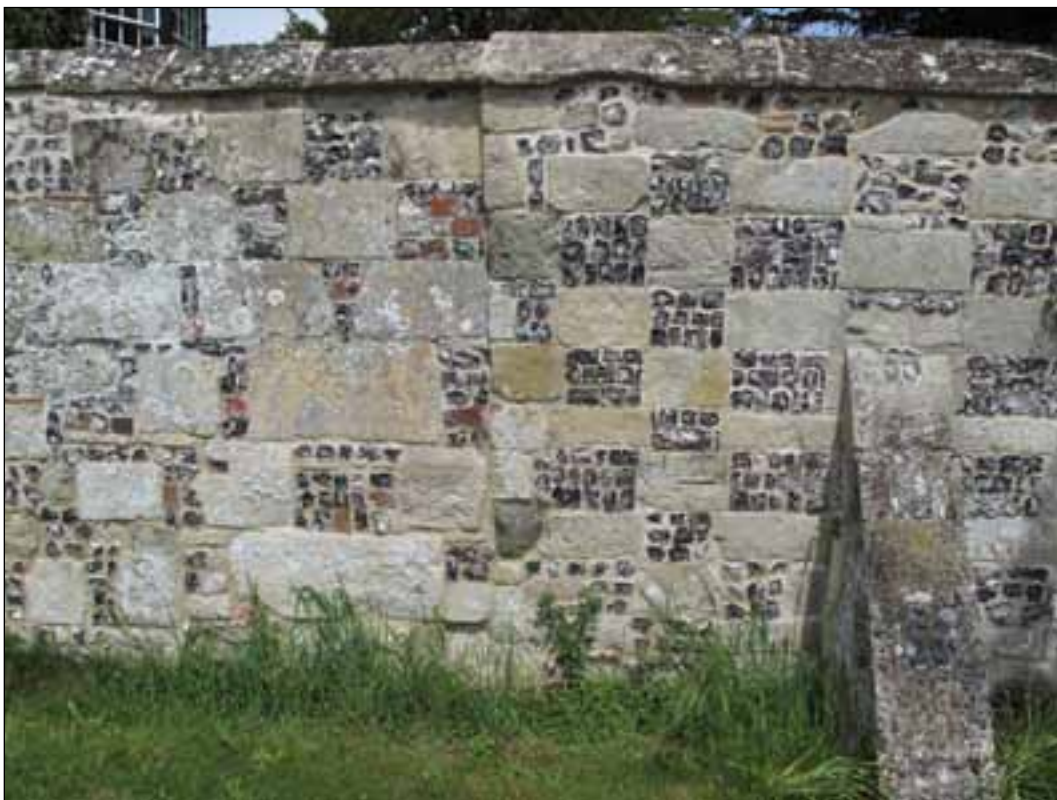
Figure 7. Surviving early flint and limestone chequer work in the garden wall of West Amesbury House
