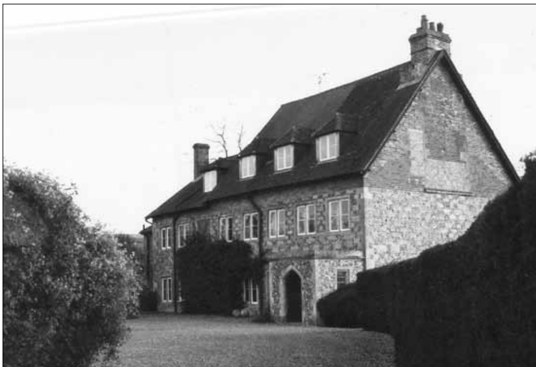
Figure 41. North and west elevations of Normanton House, showing evidence of the earlier chimney arrangement in the gable (NMR RCHME field photo, fire BF50941).
