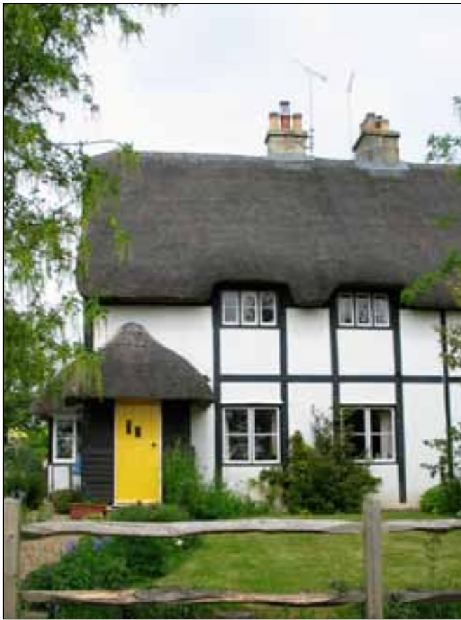
Figure 36. A concrete cottage, with applied timber frame elements, as built on the Lake Estate by Joseph Lovibond in the early 20th century
