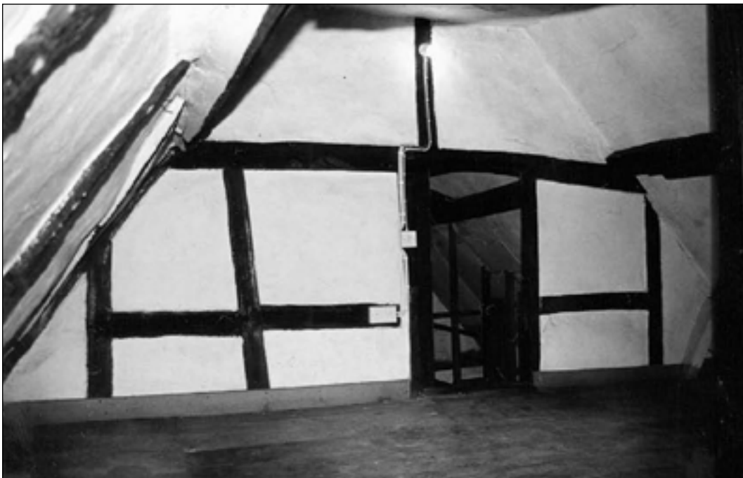
Figure 17. The attic storey of the earlier wing of Countess Farmhouse, showing the box framing of the internal partitions. Such framing may have also formed the original external walling for the house (Reproduced courtesy of the Wiltshire Buildings Record).
