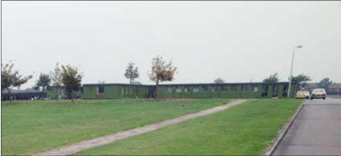
Figure 25: School Building (PIG 28850/034 © Crown copyright. NMR).
