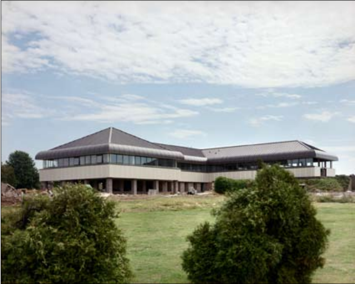
Figure 17: The main technical building (PIG 28793/001 © Crown copyright. NMR).
