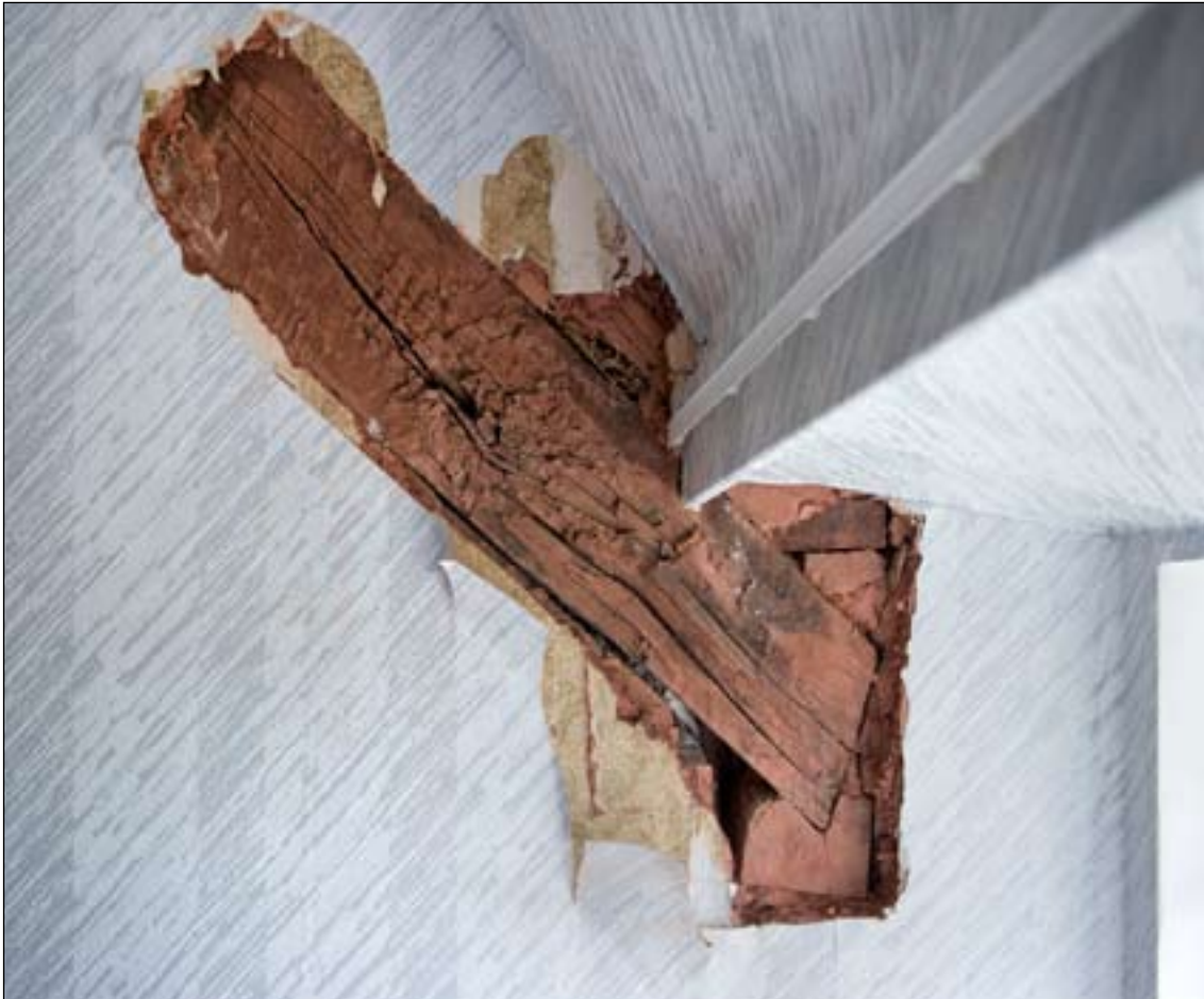
Figure 9. Southern foot of cruck C-C1, exposed at time of 2010 investigation (DPI13791).
