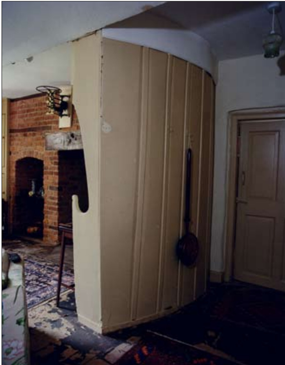
Figure 27. Interior of ground floor showing inserted brick chimney stack opening onto hall along B-B1, and settle (AA97/01519).
