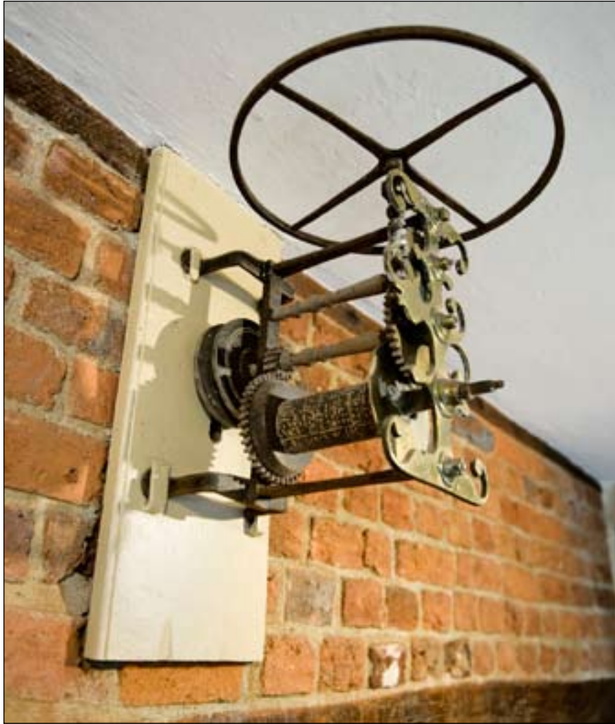
Figure 28. Turn-spit mechanism re-set above inserted fireplace at B-B1 (DP113776).
