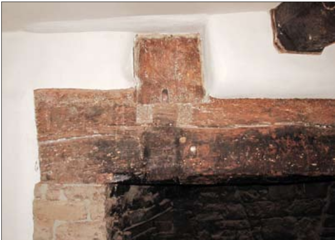
Figure 16. Chimney breast along A-A1, showing timber bressumer with chamfer and broach stops (DPI13785).
