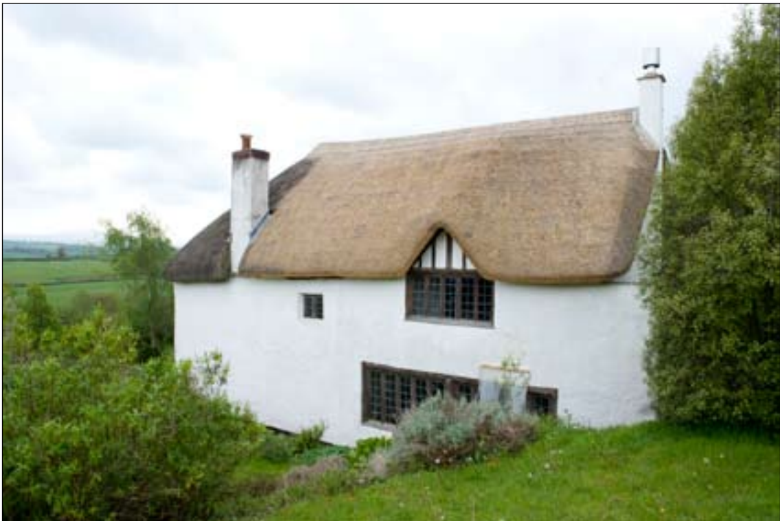
Figure 18. Exterior view from north-east showing small timber-framed gable (reconstructed in 1980s) above mullioned timber windows of north wing (DPI13772).
