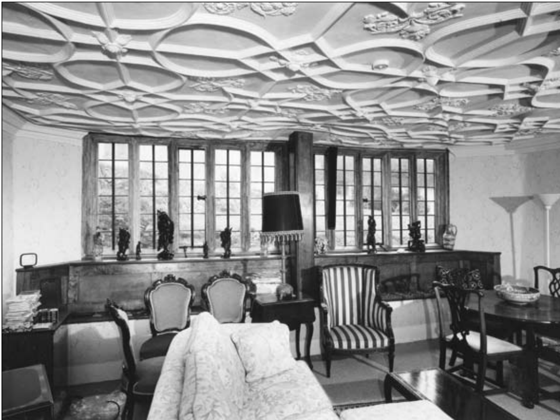
Figure 20. Ground-floor room of north wing showing ten-light mullioned window and plasterwork ceiling (BB96/03907).
