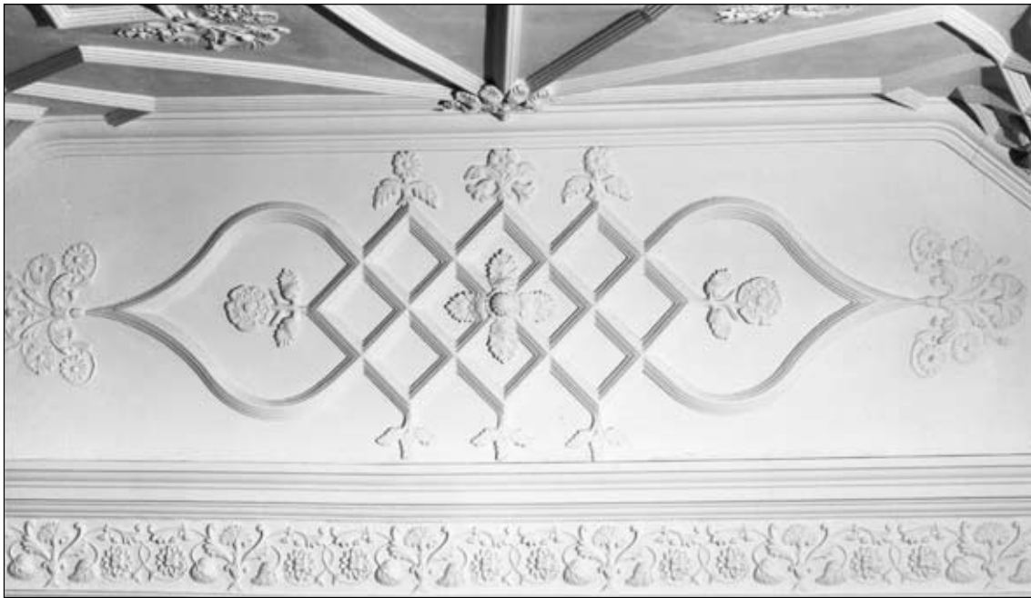
Figure 25. Detail of plasterwork on north wall of first-floor room of north wing (BB96/3912).
