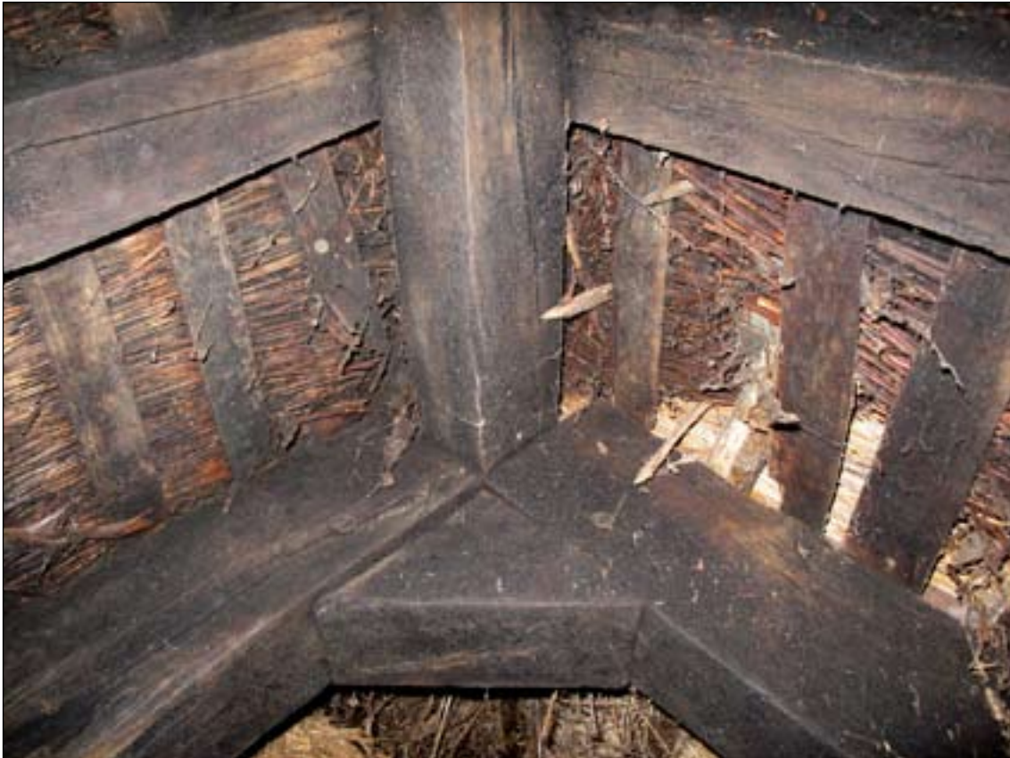
Figure 5. Diamond-set ridge piece, showing cruck blades abutting ridge purlin and joined by yoke (DPI13783).
