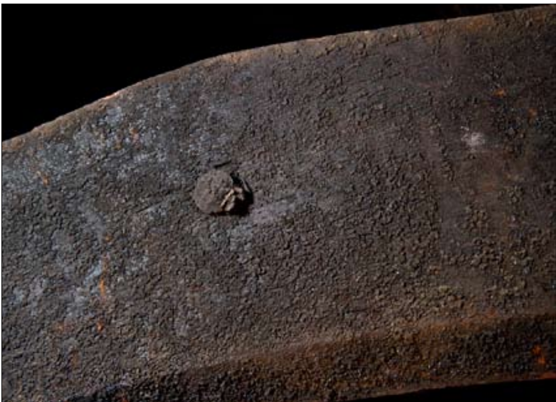
Figure 7. Detail of collar truss C-CI, showing chamfer, pegging and smoke encrustation (DPI13796).
