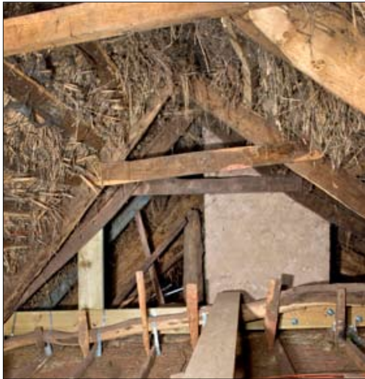
Figure 4. Roof space looking west to former position of cruck truss B-B1, showing inserted chimney stack (DPI13792).
