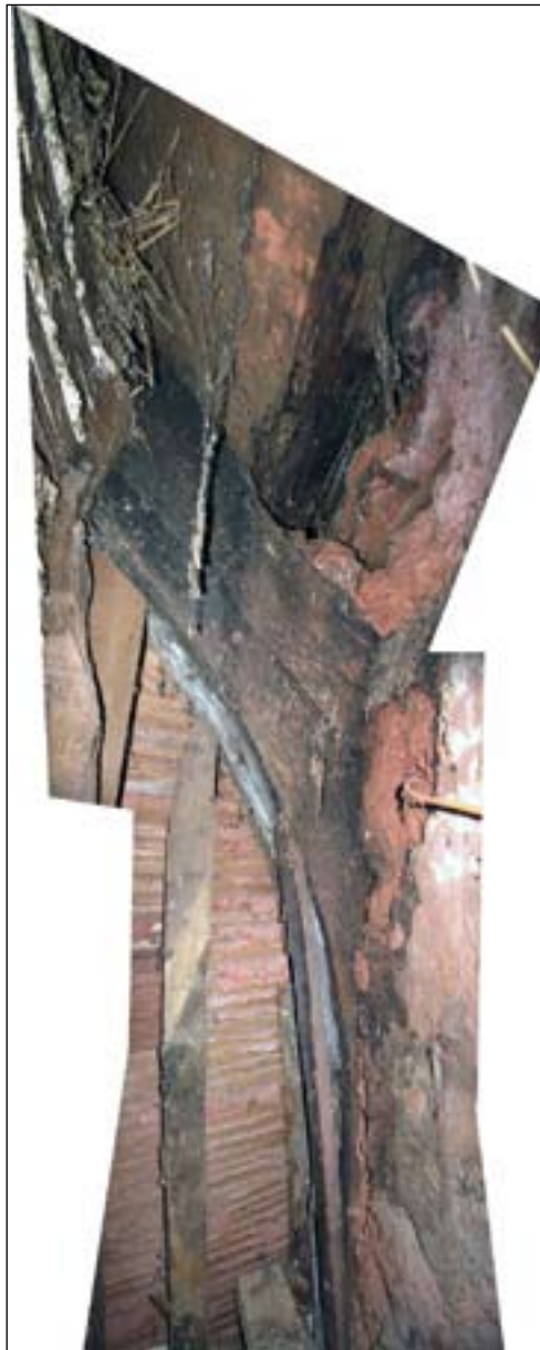
Figure 10. Northern foot of cruck C-CI, showing jointed-cruck construction (composite photograph) (DPI13802).
