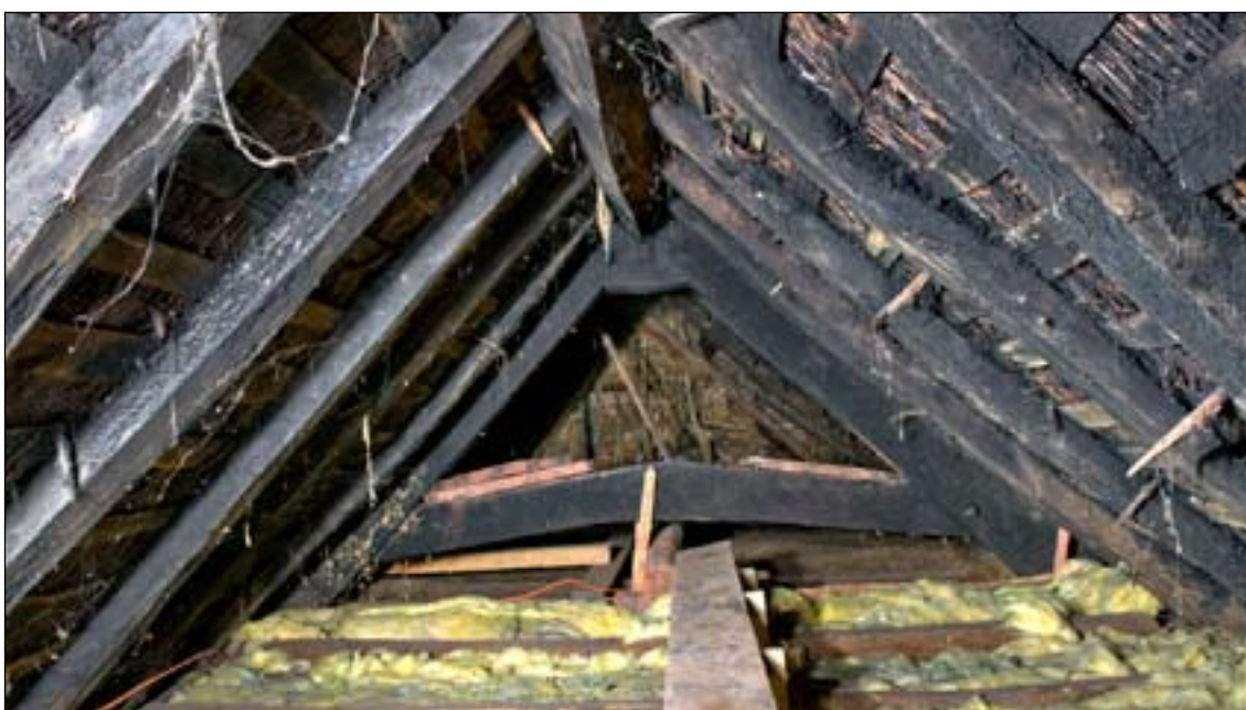
Figure 2. Roof space looking east towards cruck D-D1 showing smoke-blackened timbers and thatch (DPI13795).
