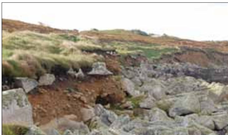
Figure 16. An example of active erosion of the low cliffs just below the breastwork to the south-west of King Charles' Battery. Photograph by Abby Hunt.
