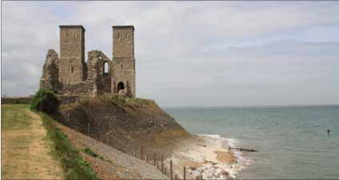
Figure 11. View of Reculver from the east, showing the present defences at the foot of the Towers and illustrating the amount of coastline already lost here. Photograph by Abby Hunt.
