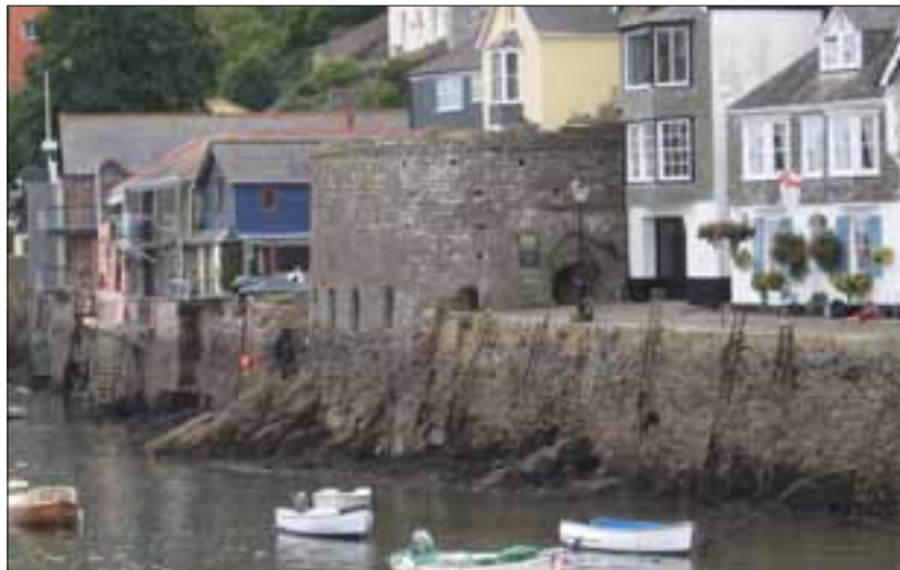
Figure 40. Bayard's Cove Fort, Dartmouth showing the apron wall on the estuary frontage. Photograph by Abby Hunt
