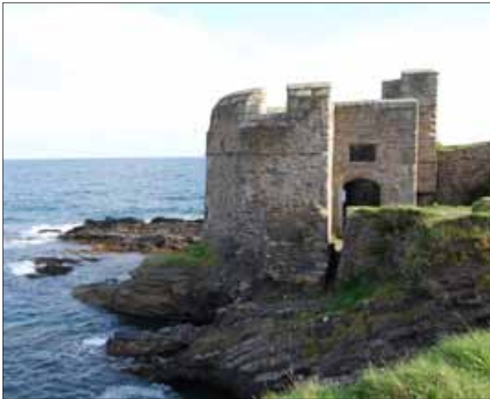
Figure 45. Little Dennis Blockhouse to the south-east of Pendennis Castle, viewed from the north. Photograph by Abby Hunt.
