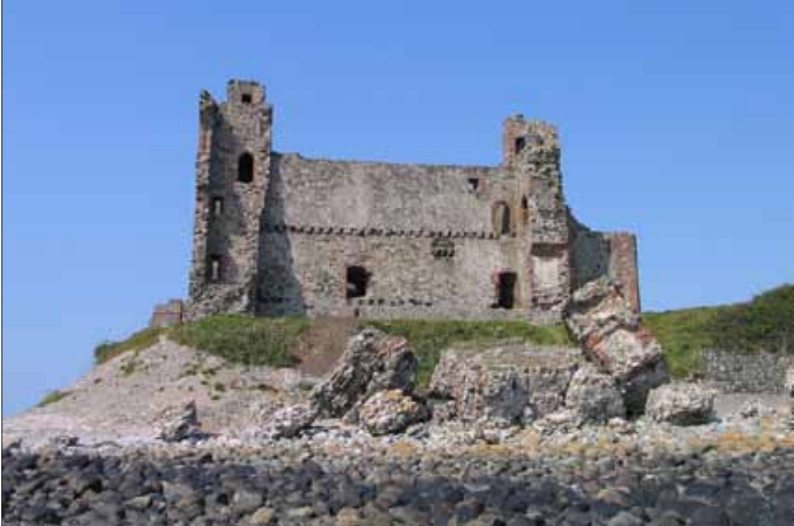
Figure 50. The eastern elevation of Piel Castle. Large chunks of collapsed masonry can be seen on the beach in the foreground, a result of erosion in the 18th century. Photograph by Abby Hunt.
