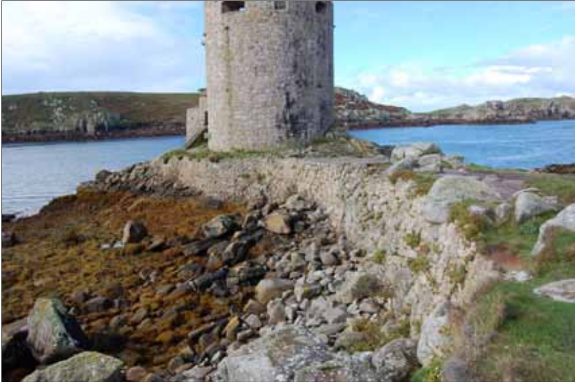
Figure 41. Cromwell's Castle, Tresco, viewed from the east. Various repairs and revetment along the neck of land joining the castle to the island are visible. Photograph by Abby Hunt.
