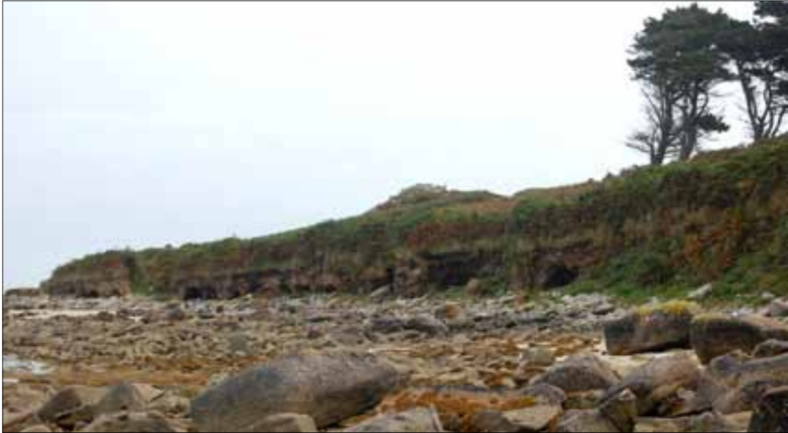
Figure 20. The coastline below Innisidgen Burial Chambers. The low cliffs are being eroded, with wave action undercutting them and creating 'caves', visible along the foot of the cliff. Photograph by Abby Hunt.
