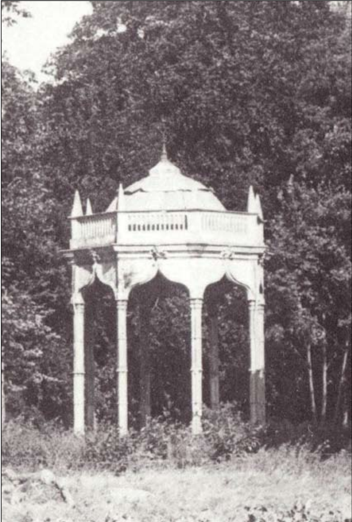
Figure 4. The 'Umbrello' photographed in the 1960s and showing the original domed roof.
