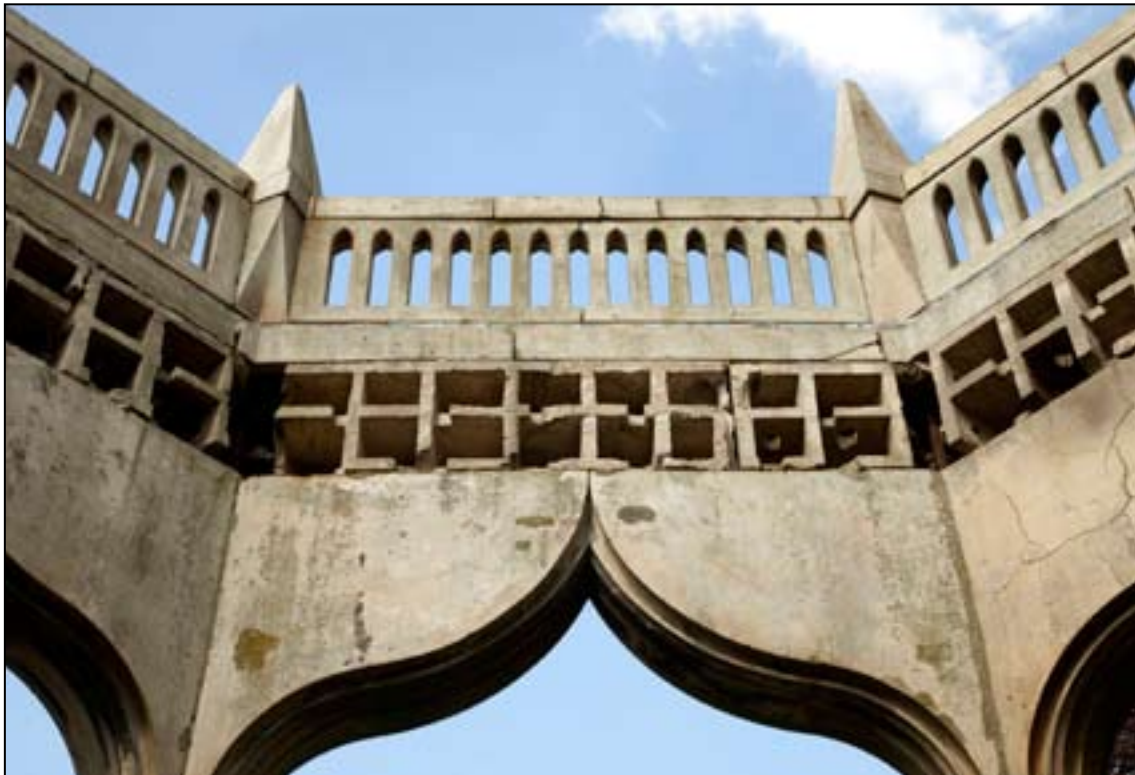
Figure 12. The 'Umbrello' showing the now exposed hollow internal structure of this Coade stone building. Pat Payne DPI41286.JPG
