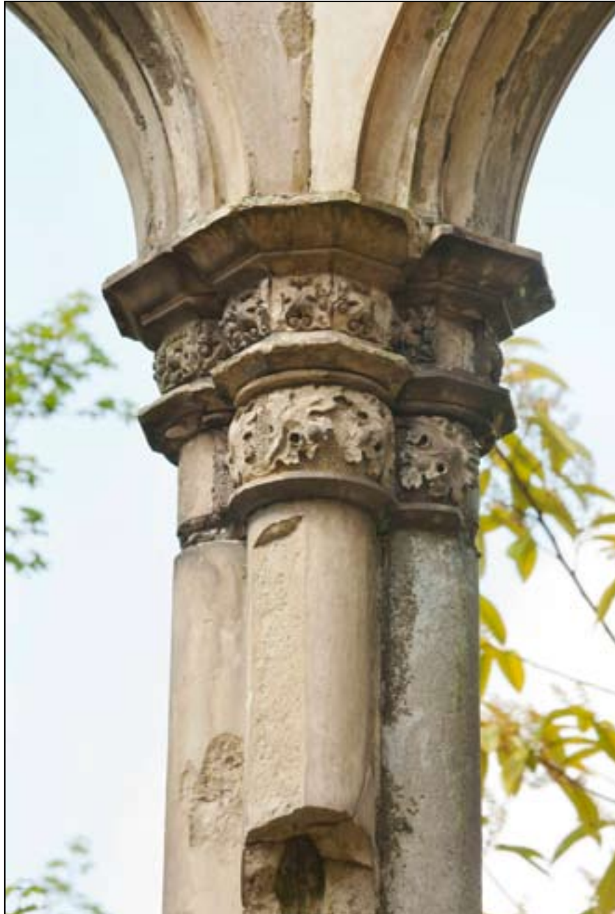
Figure 8 The 'Umbrello' showing the damaged foliate capitals and one of the broken hollow column shafts. Pat Payne DPI41292.JPG
