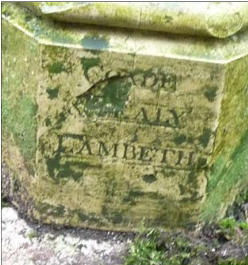
Figure 3. The 'Umbrello'. The base of one of the columns embossed 'COADE & SEALY LAMBETH.'
