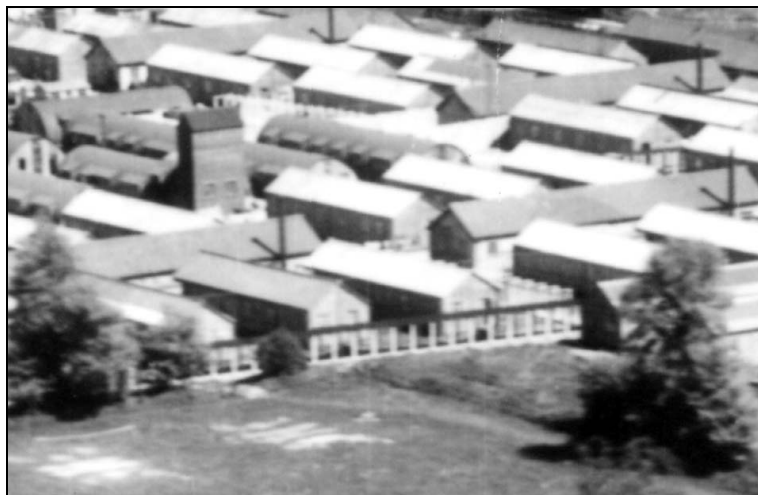
Figure 44 New buildings at Devizes barracks, part of the southern hospital (with rounded roofs and a wooden tower) connected to the existing barrack buildings (pitched roofs) by a network of covered walkways, in the foreground. Detail of US/31GR/LOC50 5125 30-April-1944. English Heritage USAAF Photography
