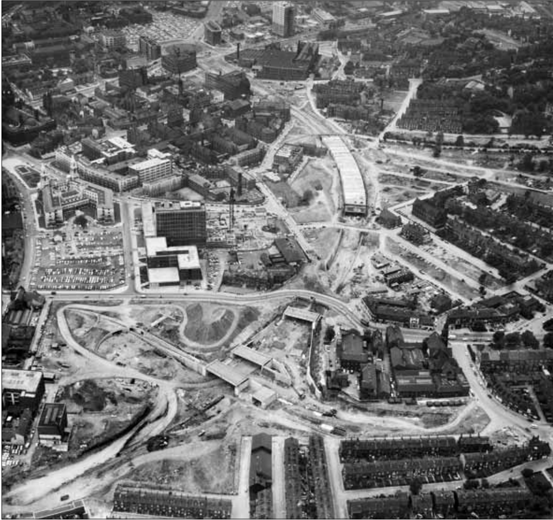
Figure 7 - Leeds inner ring road under construction, 1964 (AFL03/Aerofilms/A146965 © English Heritage.NMR. Aerofilms Collection)
