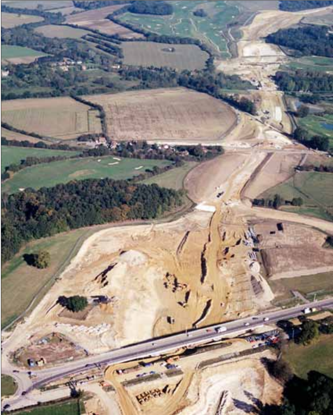
Figure 18 - The Newbury Bypass under construction in Berkshire, 1997, looking north-east, with the A4 in foreground (© English Heritage NMR 15811/03 NMR 23-Oct-1997).
