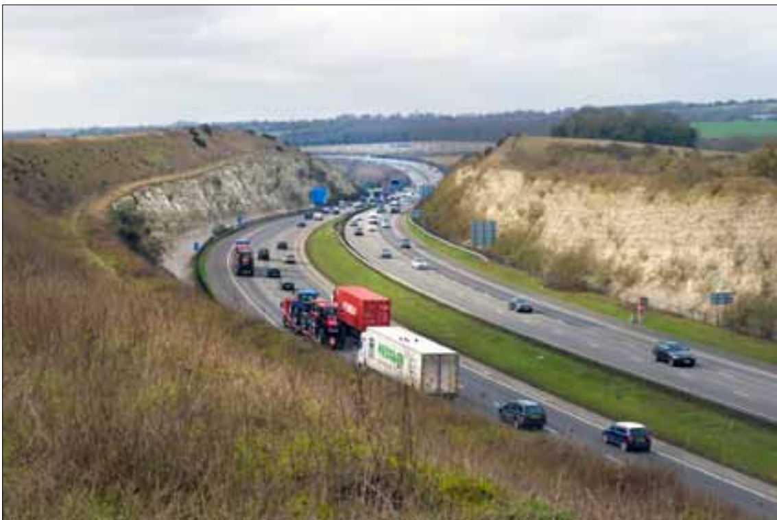
Figure 24 - The M3 cutting looking south, February 2011 (Peter Williams © English Heritage DPI39175)
