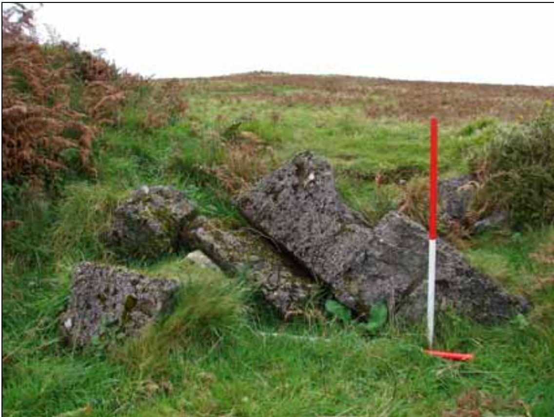
Fig 9: The concrete blocks left from the blondin pylon footings on platform D.
