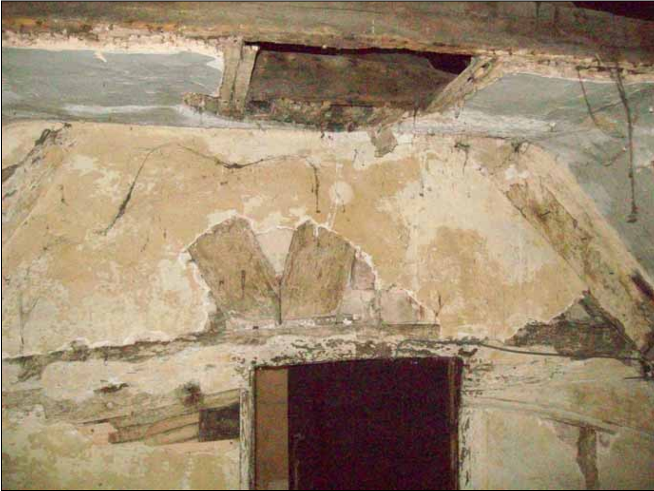
Figure 5: Central truss (south face)
