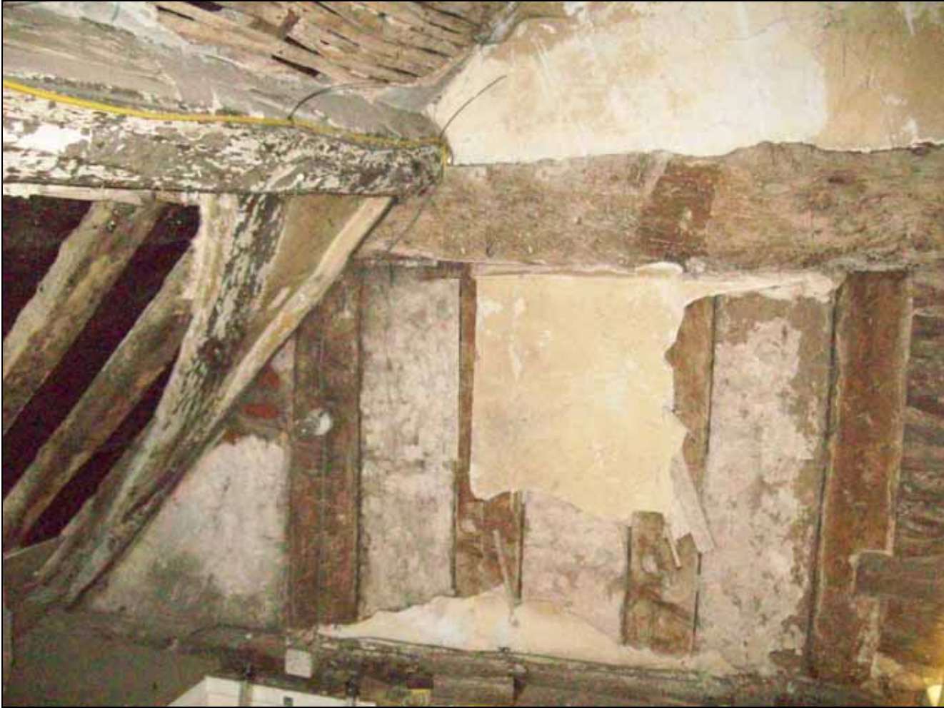
Figure 4: South gable truss (north face)
