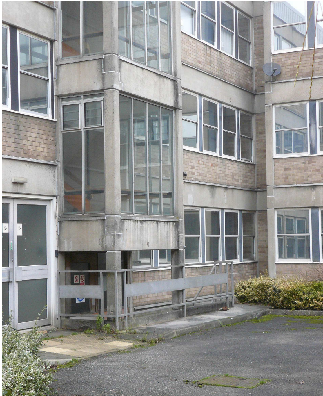
Copenacre, Wiltshire, office building built in about 1959 to accommodate many of the 400 personnel moved from Risley to Copenacre in 1960. © English Heritage
