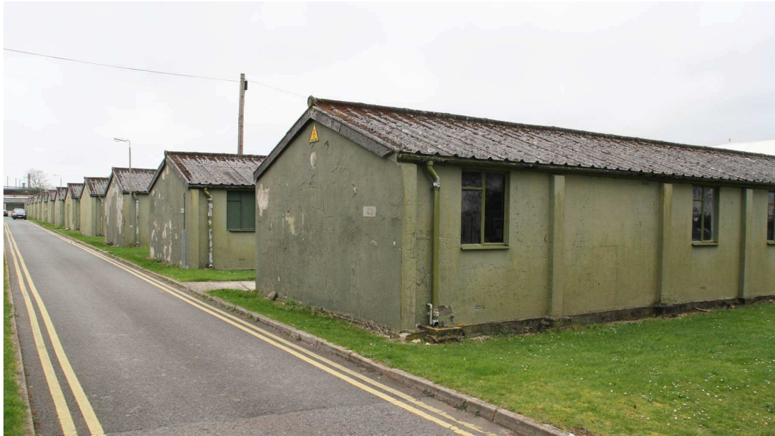
RAF Lyneham, Wiltshire, barrack blocks probably refurbished during the 1950s. © English Heritage
