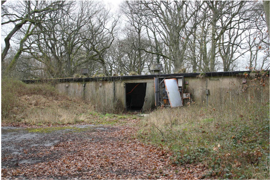
RAF Chilmark, Wiltshire, magazine in Moses Wood, later air conditioning plant was probably installed for the storage of guided missiles. © English Heritage
