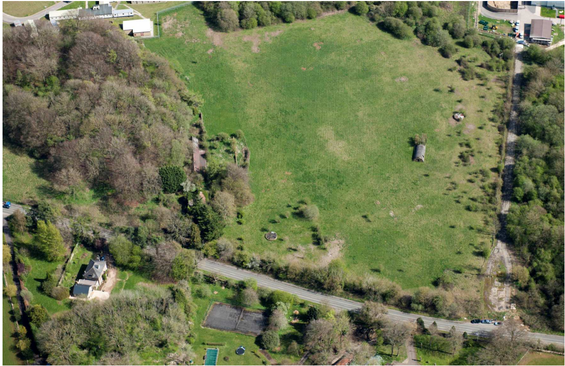
Gorse Farm, Corsham, Wiltshire, Gorse Farm house is to the centre left, also visible in this field is an air vent for the underground working and a curved asbestos hut. © English Heritage NMR 26907-002
