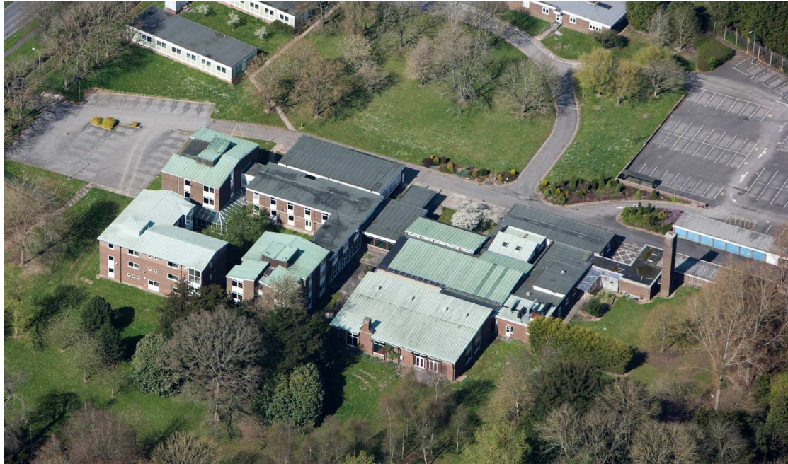
Erskine Barracks, Wilton, Wiltshire, late 1950s or early 1960s officers' mess, attributed to the Salisbury architectural practice of the Brandt, Potter, Hare Partnership. Its large size probably reflects the high percentage of officers stationed at the head quarters. © English Heritage NMR 26912-046
