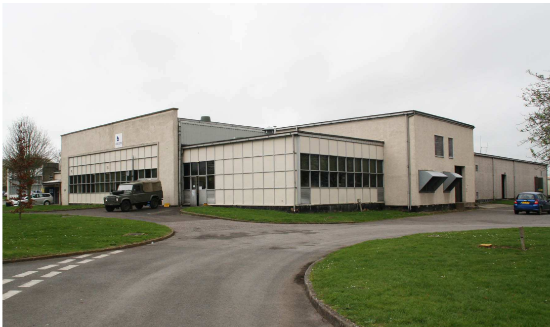
RAF Lyneham, Wiltshire, late 1950s avionics building, this was probably built to coincide with the introduction of the Comet airliner. © English Heritage
