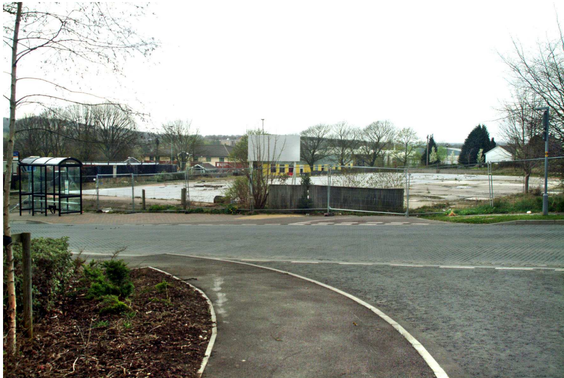
Tidworth, Wiltshire, floor slab of former NAAFI complex. © English Heritage
