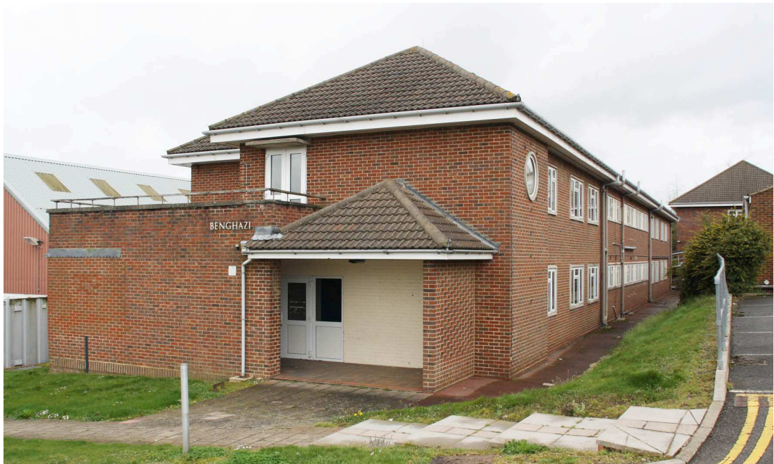
Erskine Barracks, Wilton, Wiltshire, early 1950s barracks with later pitched roof. © English Heritage
