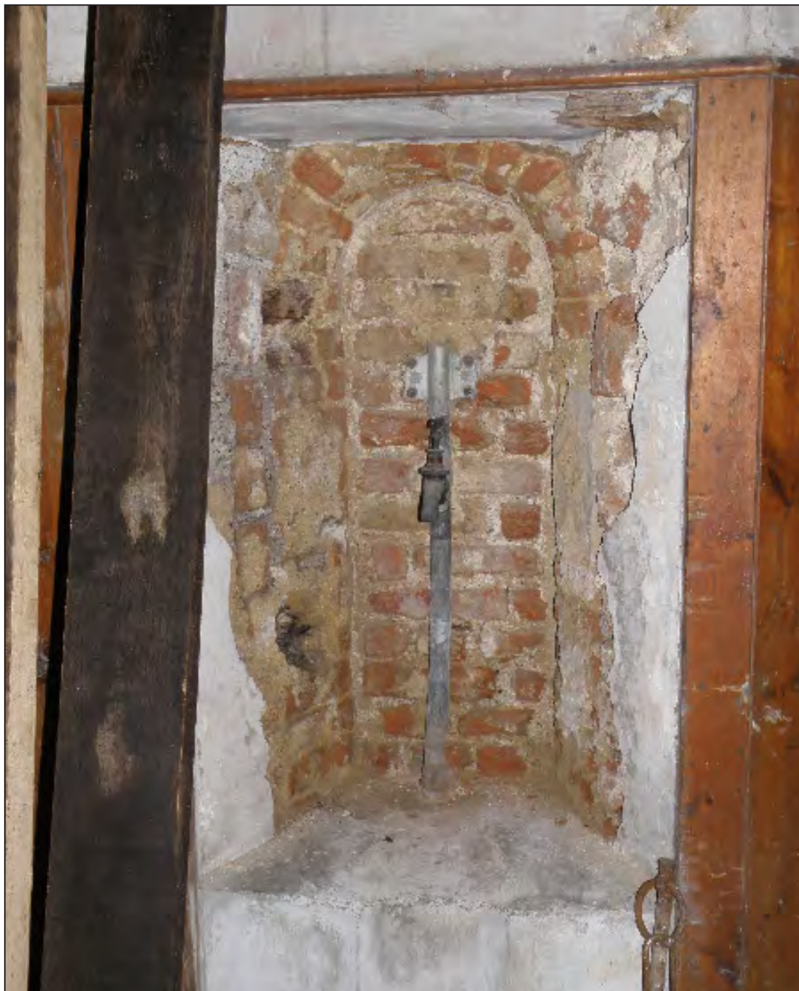
Figure 2I. The niche on the south wall of the West Stable showing the blocked central light of the original three-light mullion window.
