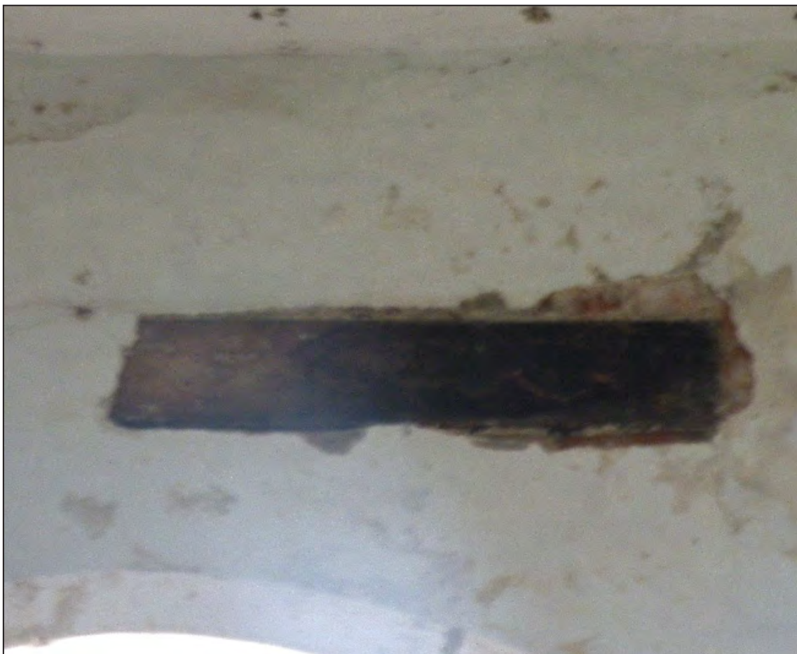
Figure 20. The former lintel to the original three-light mullion window which existed at first-floor level before the bays were added when the building was converted into a stable. Pete Smith P1010016A.JPG
