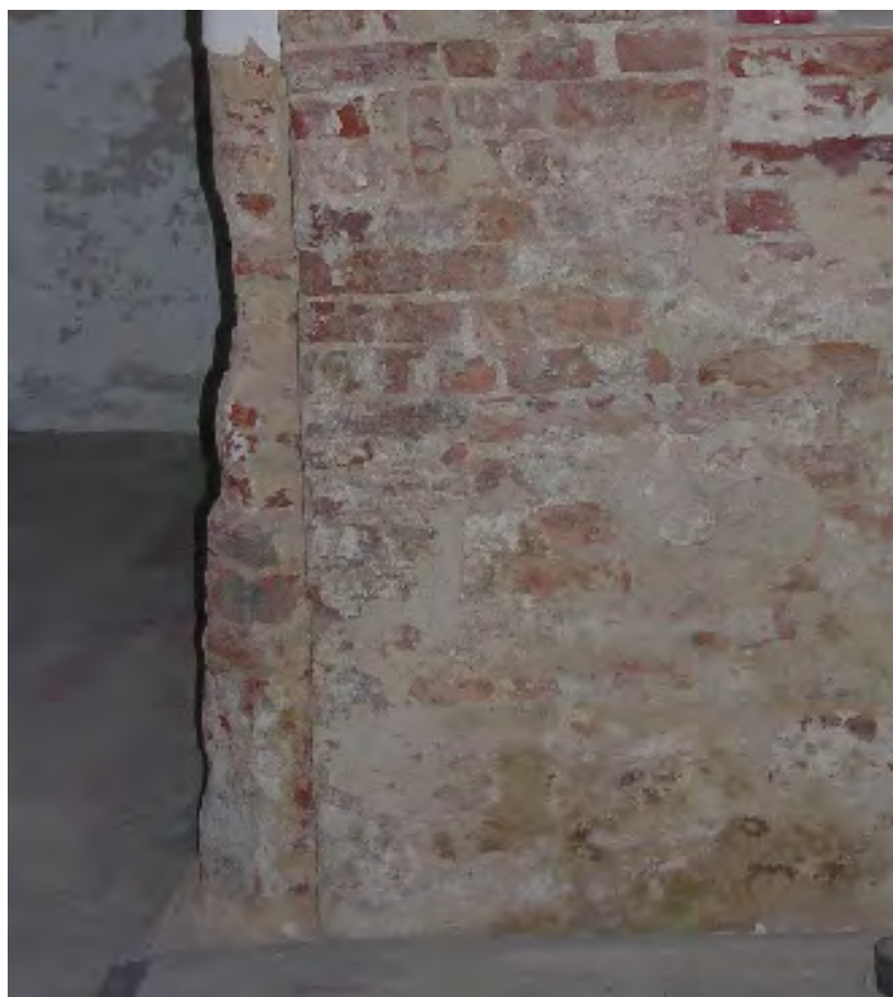
Figure 12. The west respond of the south arch with the plaster removed.
