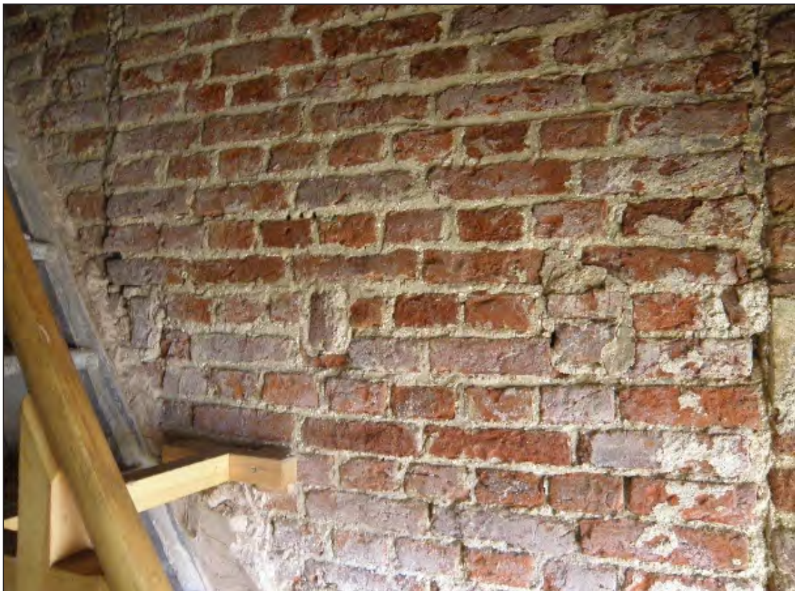
Figure 25. The northern section of the west wall, now within the stair compartment, showing the north blocked doorway at first-floor level. The blocked sockets for floor beams correspond in level with those found across the remainder of this wall. The plaster was not renewed as part of the repairs. Pete Smith PI010023.JPG
