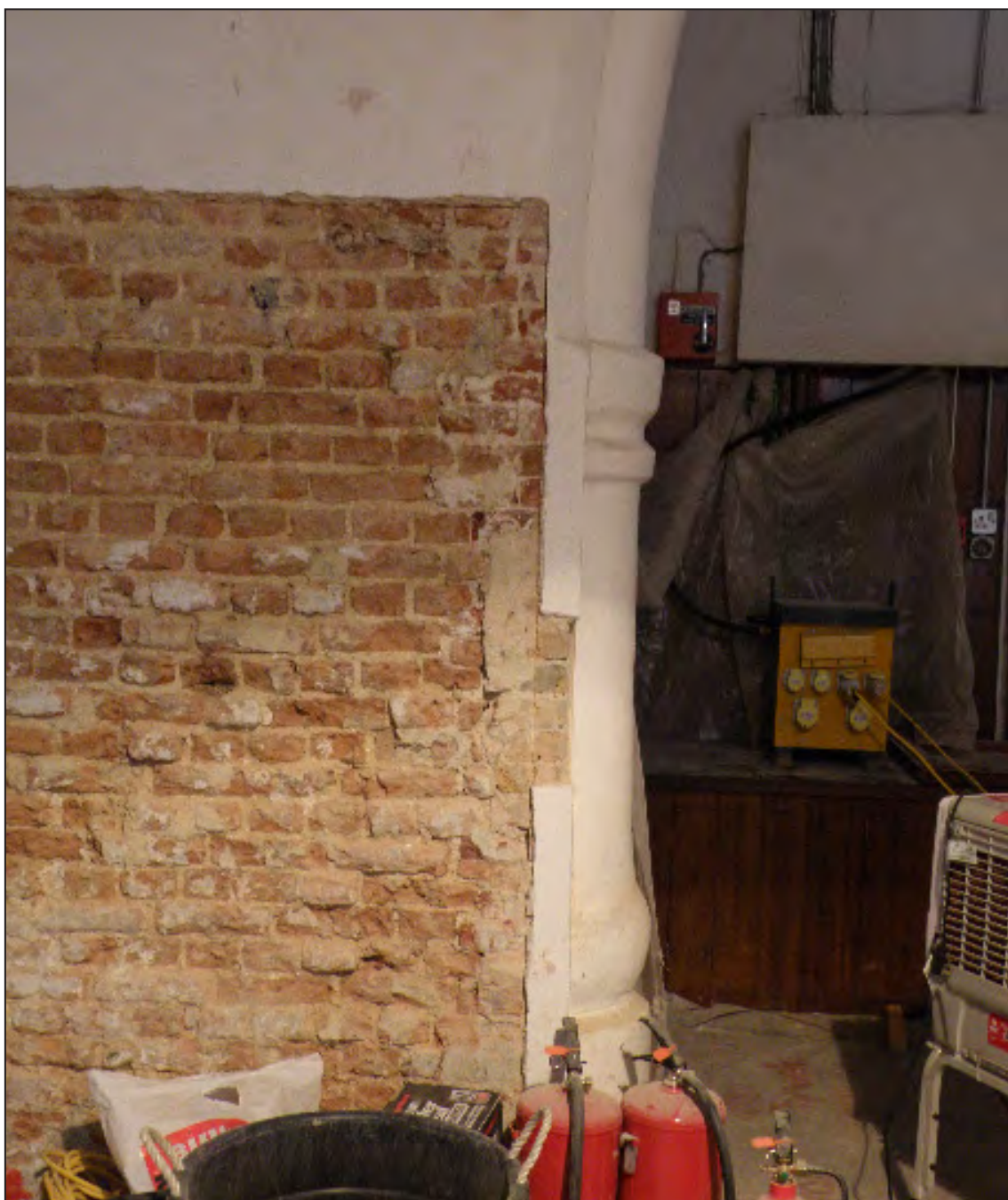
Figure 8. The wall to the west of the west respond to the north arch with the plaster removed. Pete Smith PI010033.JPG
