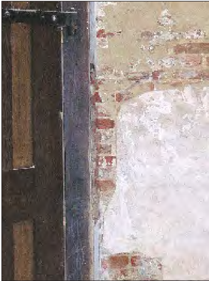
Figure 14. A detail of the jamb of the central doorway inserted into the north wall of the central crosswing with the plaster partially removed.
