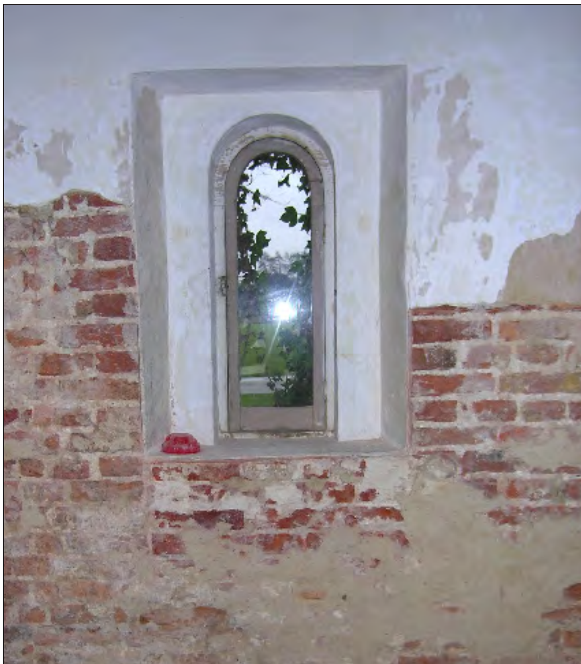
Figure 17. The single-light porter's window on the south wall, showing the cill raised in darker red brick. DSCN6714A.JPG
