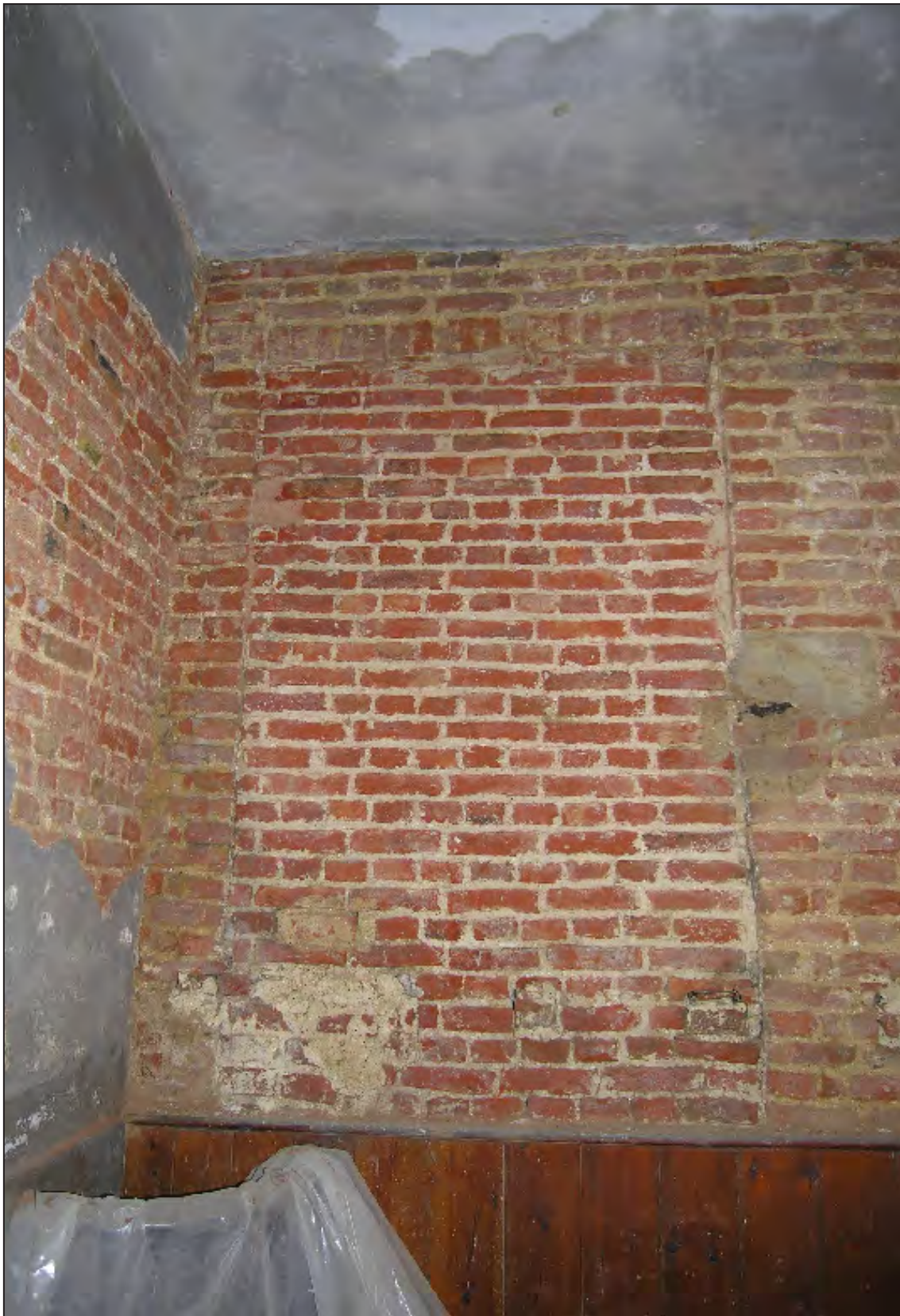
Figure 24. The southern section of the west wall of the West Stable after the plaster had been removed showing the south blocked doorway at first-floor level. Pete Smith DSCN6730.JPG
