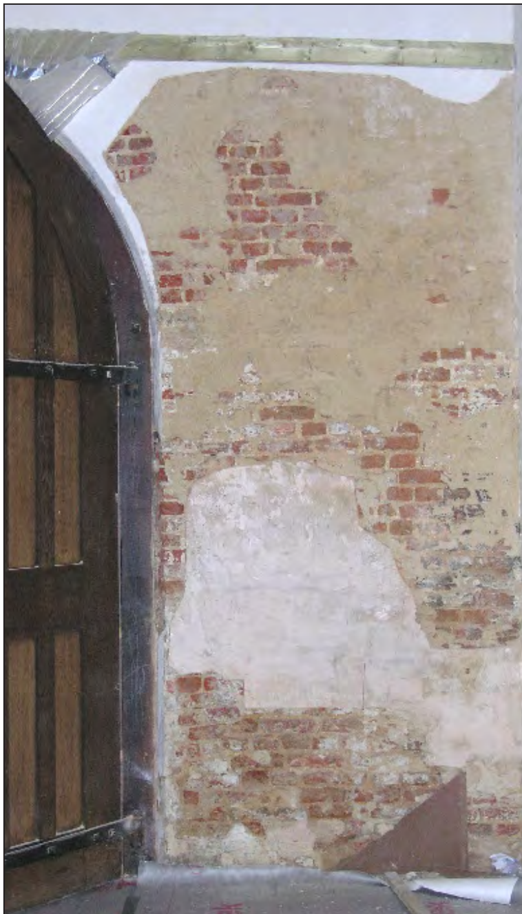
Figure 13. The north wall of the central crosswing, showing the partial removal of the plaster from the wall to the east of the central coach house doorway.
