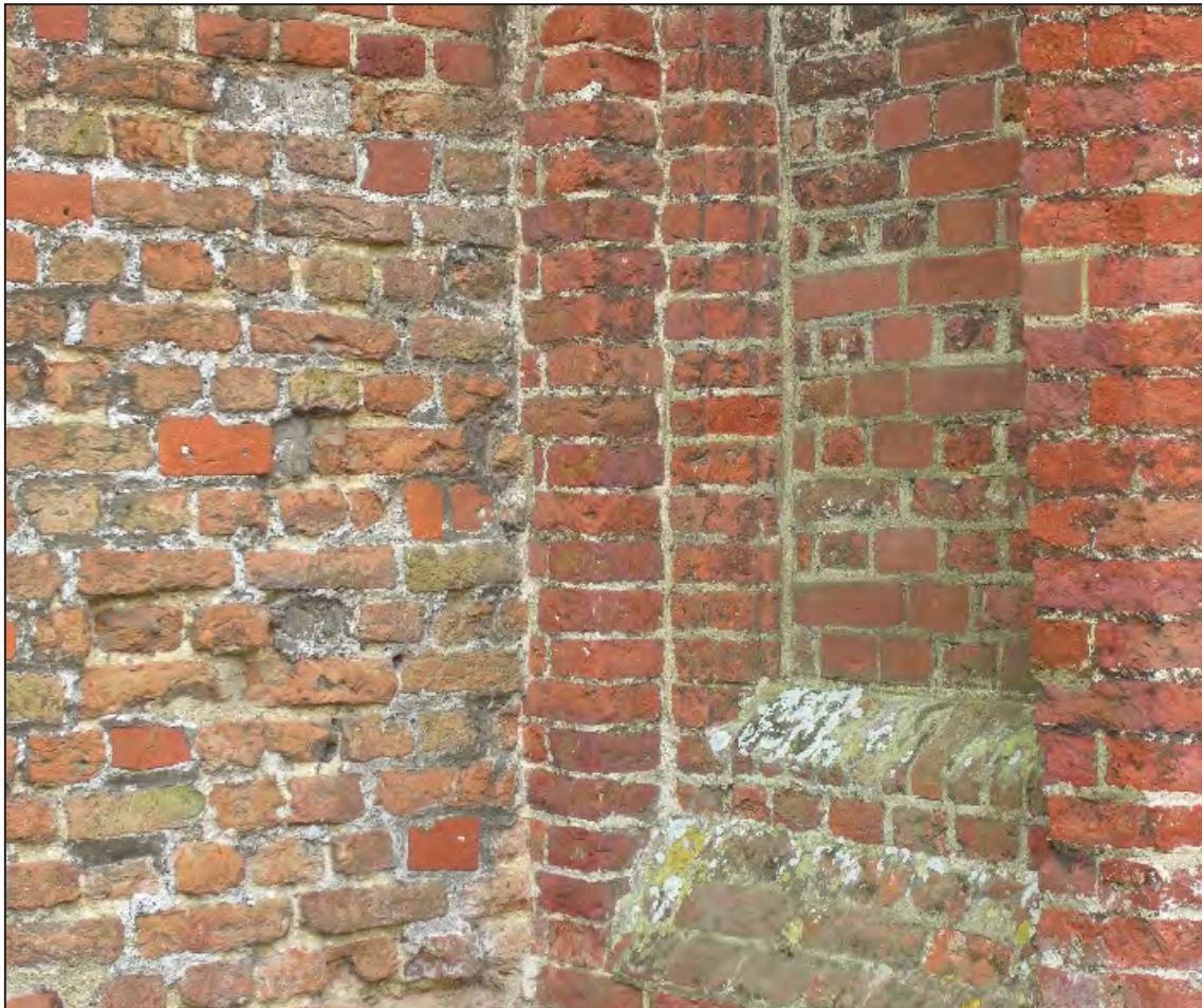
Figure 29. A detail of the north front showing the junction of the orange brick of the original walling (left) and the added western bay constructed of darker red brick (right). The brick coursing does not carry through.
