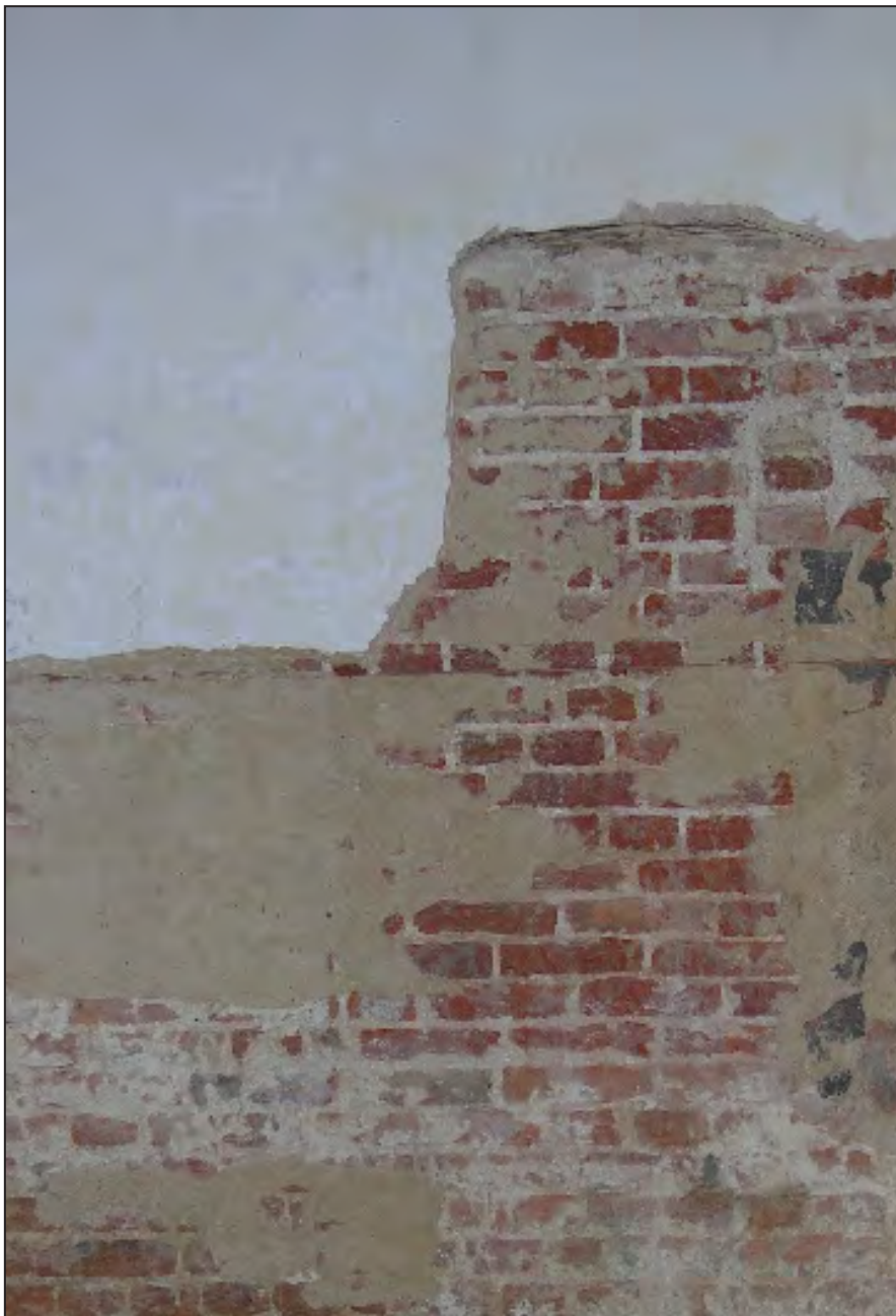
Figure 18. The south wall of the coach house, showing the timber lintel and the inserted darker red brick blocking the former three-light window to the west of the central crosswing.
