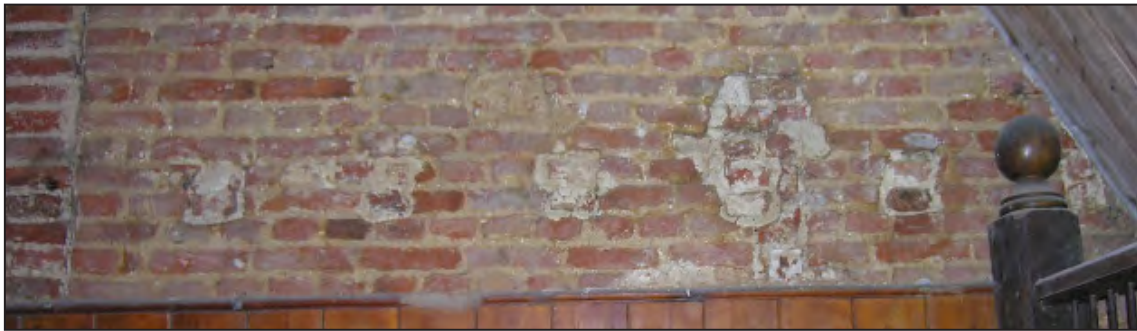
Figure 27. The southern section of west wall of the West Stable showing the blocked sockets for floor beams. Pete Smith DSCN6735A.JPG
