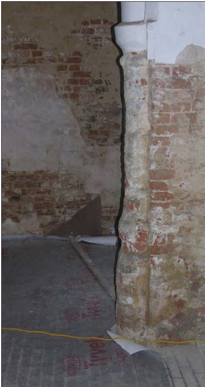
Figure 10. The east respond to the north arch with the plaster removed.
