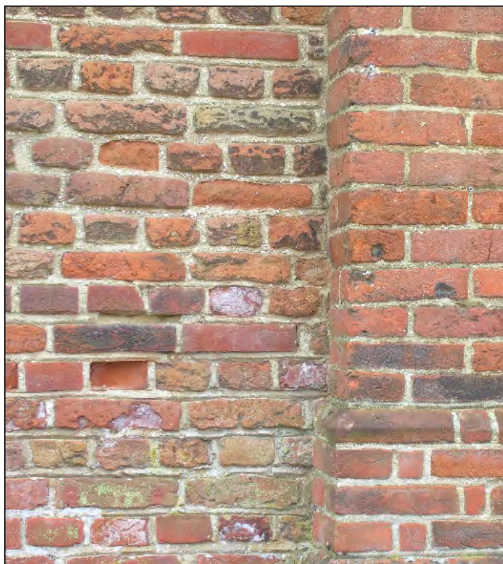
Figure 15. A detail of the exterior of the north wall of the central crosswing showing the clear difference in brick used for the original walling (left) and the darker red coloured bricks of the inserted central door surround (right).
