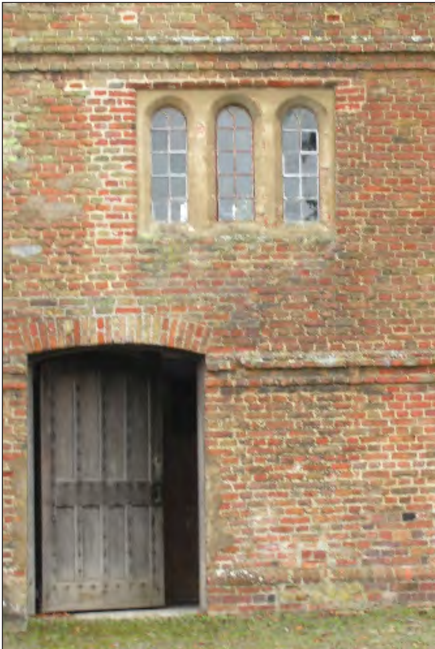
Figure 22. The north front showing the door to the West Stable and the surviving upper three-light window. The internal niche, which survives from original three-light ground floor window is sited immediately below the central light of the first floor window.
