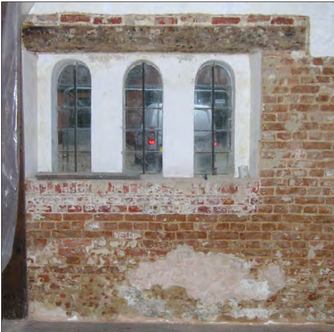
Figure 16. The three-light mullion window on the north wall, showing the cill raised in darker red brick. Pete Smith DSCN6716A.JPG
