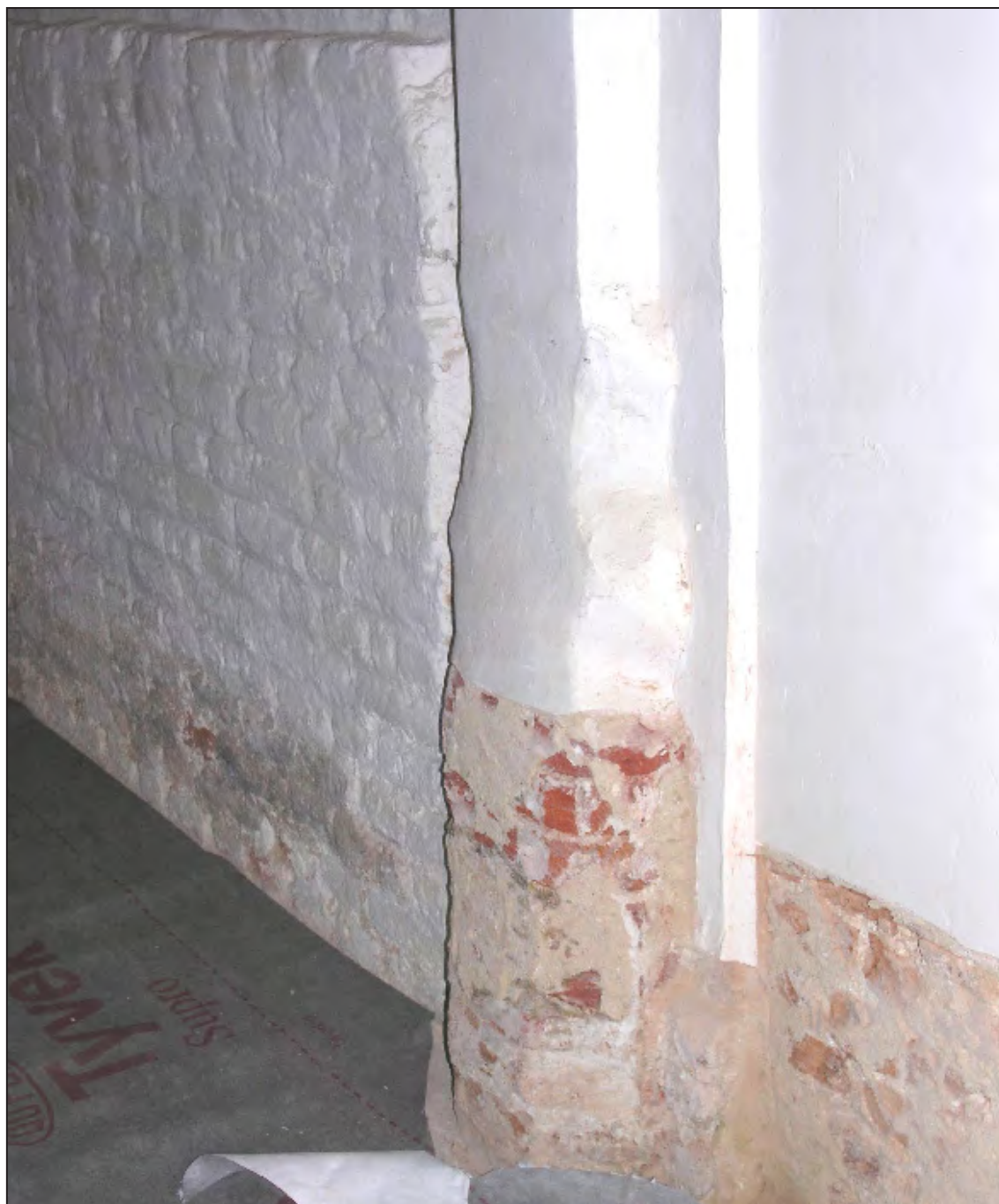
Figure 11. The base of the east respond to the south arch with the plaster removed.
