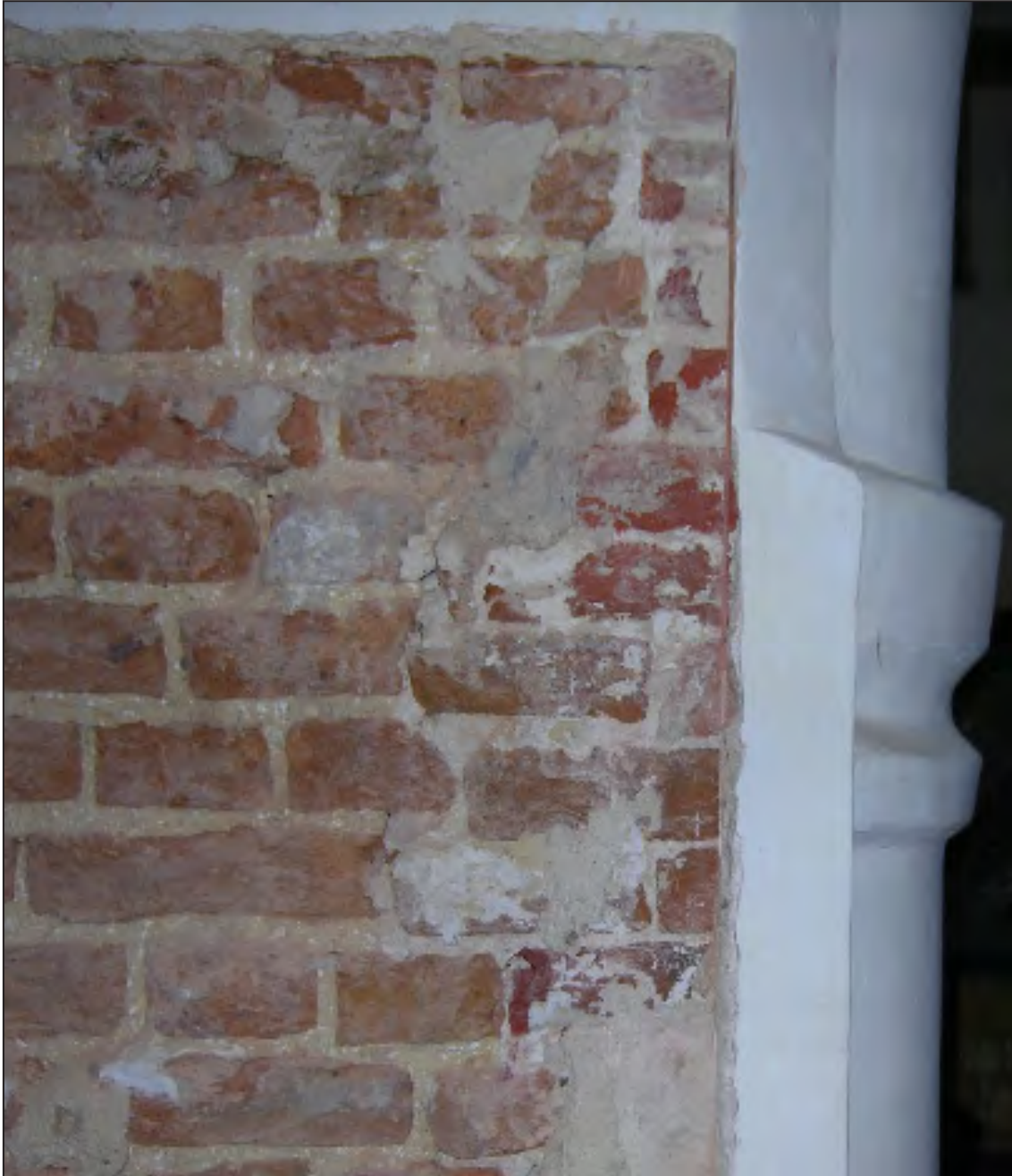
Figure 9. A detail of the exposed wall to the west of the west respond on the north arch showing the much darker red brick used to construct the respond to the arch and the original orange brick with cream mortar of the pre-existing wall.
