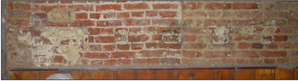
Figure 26. The northern section of west wall of the West Stable showing the blocked sockets for floor beams continuing across the north blocked doorway. Pete Smith DSCN6733A.JPG
