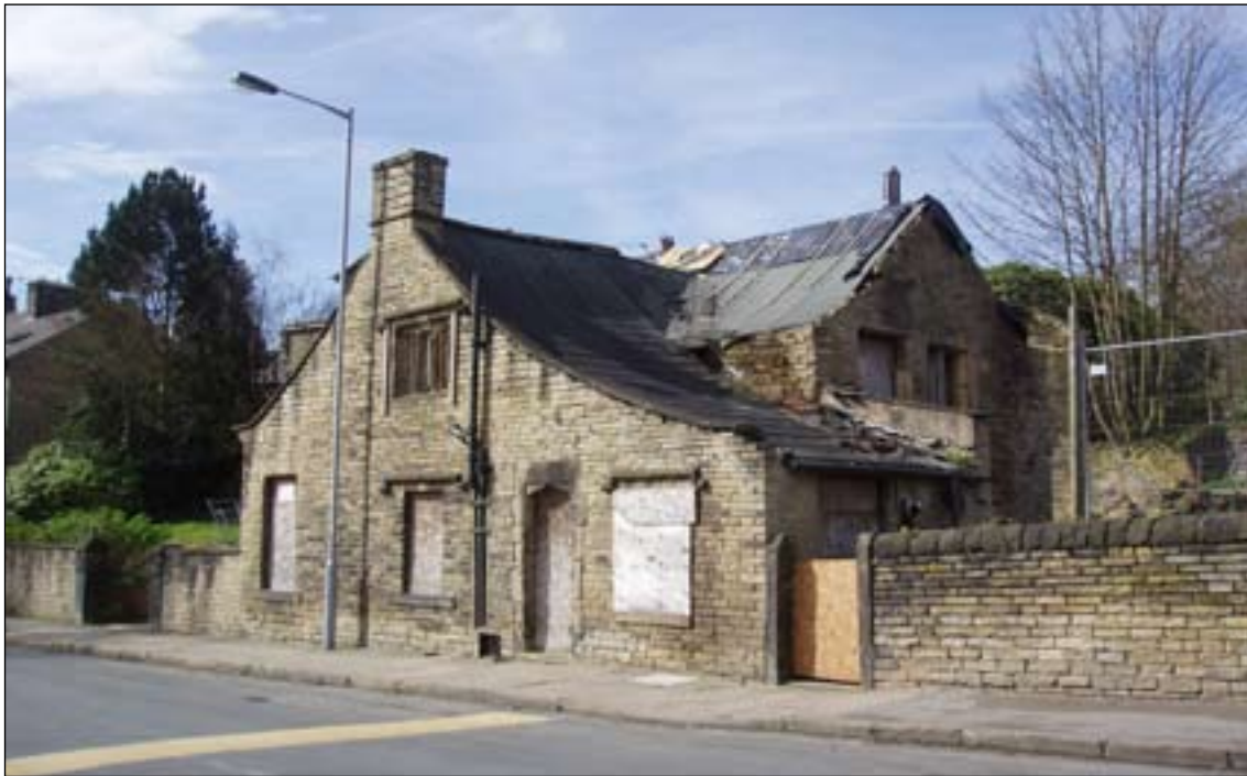
Fig 19: Old Manor House from north-east: the aisled structure of the medieval house was retained in the 17th century rebuilding in the area of the housebody: the roof sweeps down to single-storey height to both north and south (© English Heritage)
