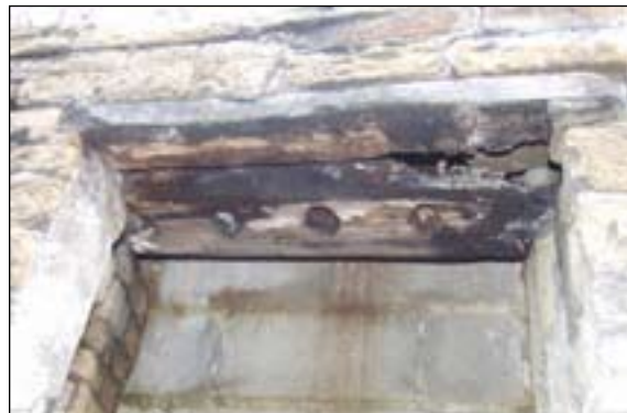
Fig 15: lintel of timber-mullioned window, west cross wing, west wall north end (© English Heritage)
