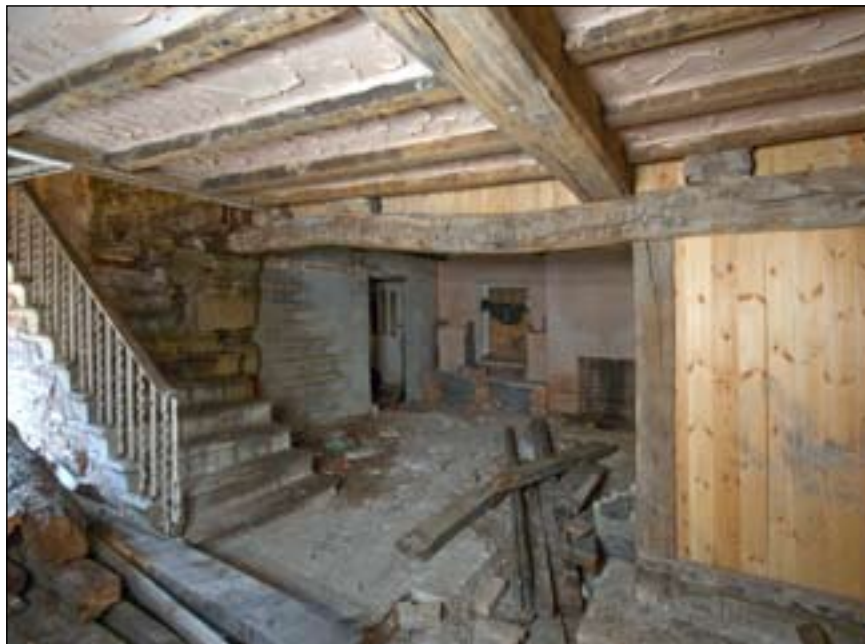
Fig 23: west wing, view to north-east showing inserted stone stair with iron balusters (DP071458 © English Heritage)
