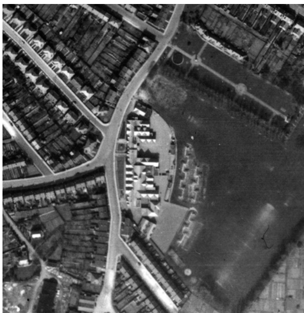
Figure 66 Civil defence structures in Naunton Park, Cheltenham. Detail of RAF 106G/UK/1354 7390 02-APR-1946. English Heritage (NMR) RAF Photography
