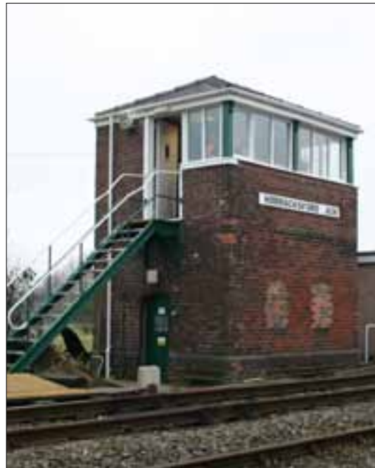
Figure 11a Horrocksford Junction after renovation. © Charles Weightman
