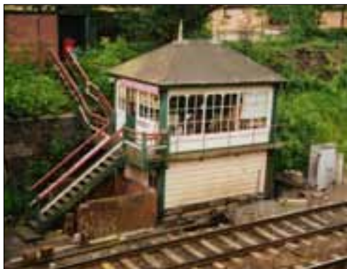
Figure 1 Totley Tunnel signal box in 2003 before renovation. © John Minnis
