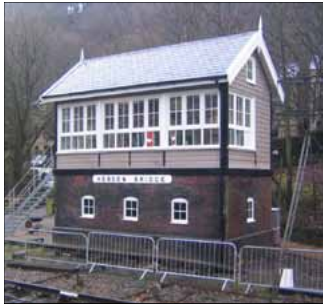
Figure 31 Hebden Bridge. © Construction Marine Ltd.
