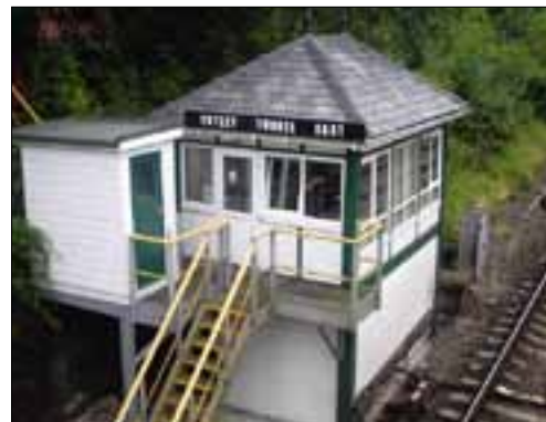
Figure 2 Totley Tunnel signal box after renovation. © John Tilly
