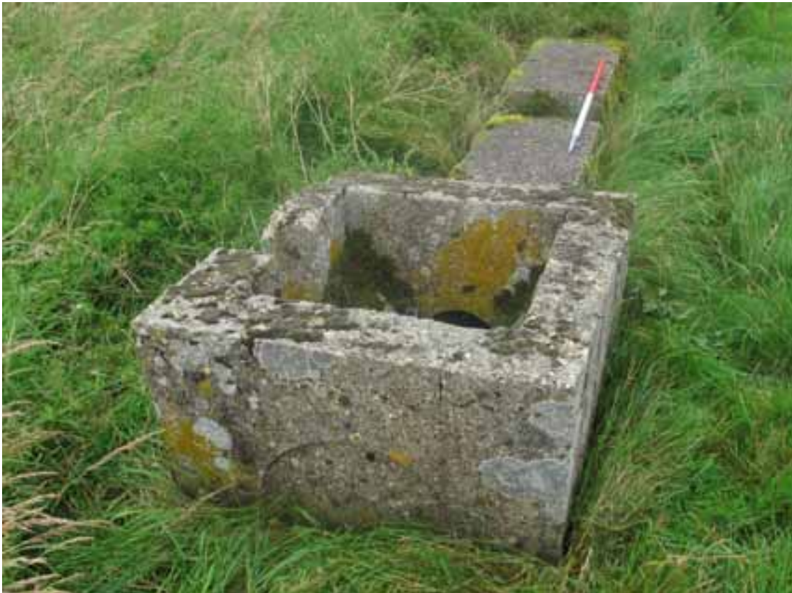
Fig 17: Concrete box and section of pipe casing, part of the military sewage works in Stonehenge Bottom.
