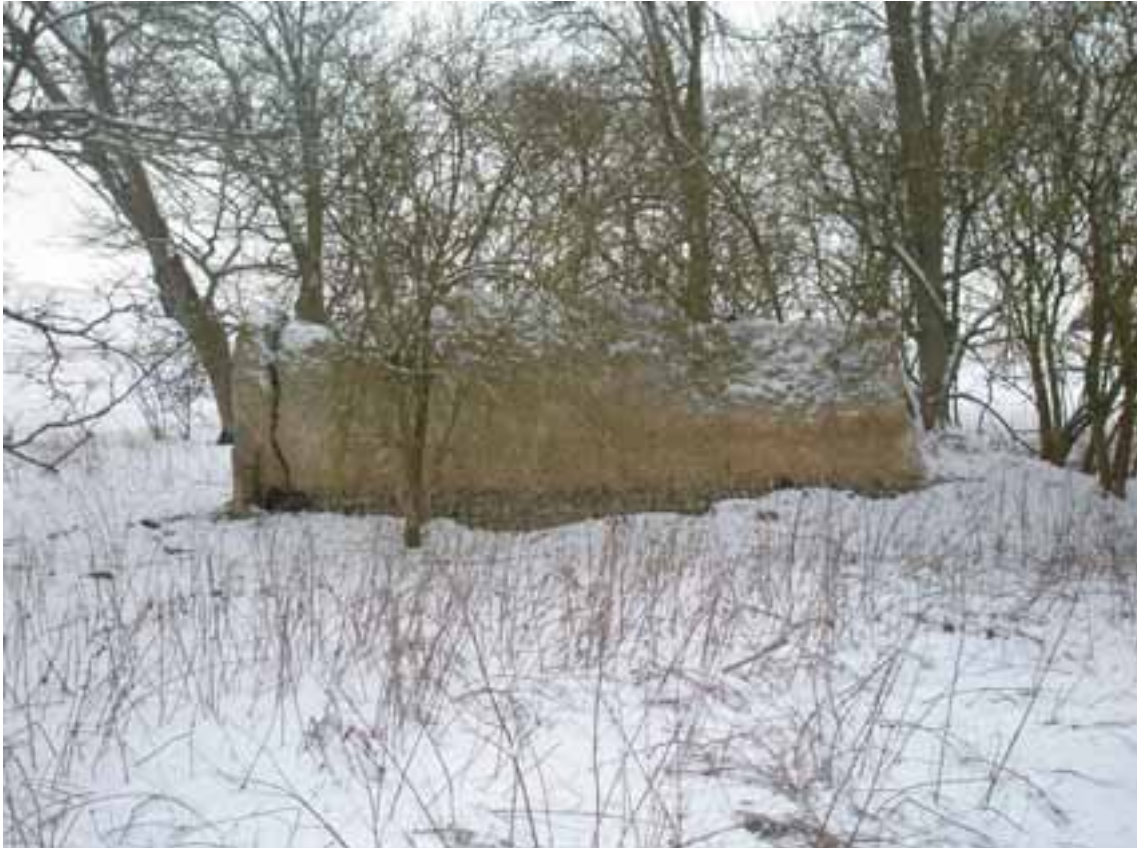
Fig 4: Remains of the well house in Spring Bottom south of Springbottom Farm, near Lake, built of cob and clunch with brick facings; the well house in Stonehenge Bottom to the south of the Cursus was probably similar.
