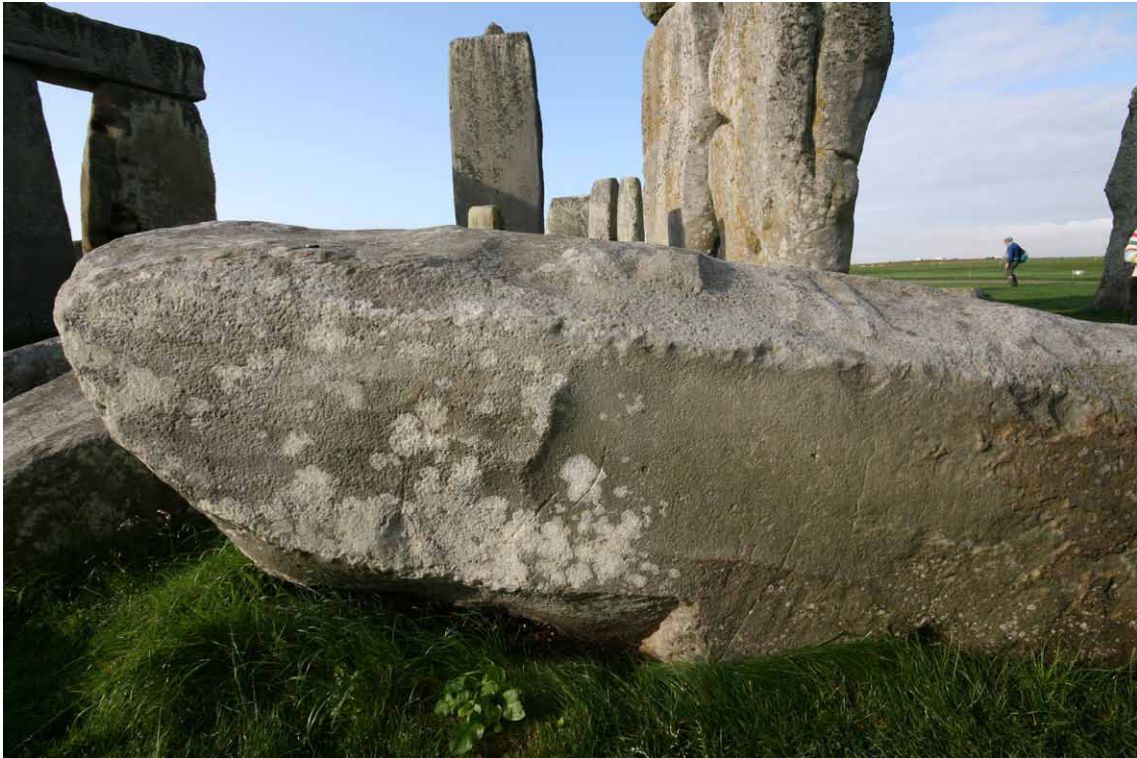
Figure 7. Very coarse pick dressing on a rebate in Lintel 102. The rebate is the rectangular depressed area directly above the upright. (Photograph Hugo Anderson-Whymark)
