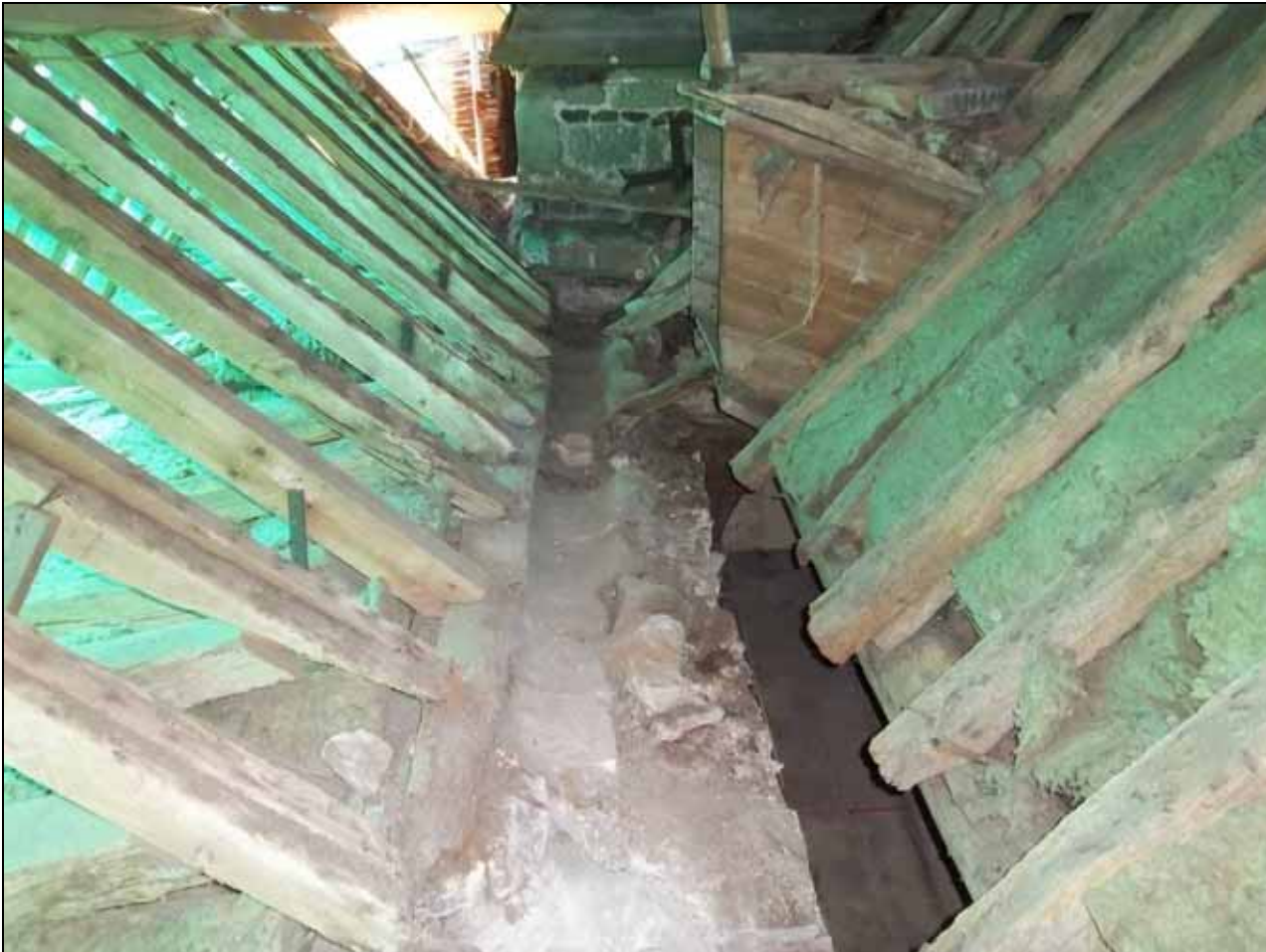
Figure 7: Stone gully between south aisle (to left) and nave (to right) roofs. Photograph Robert Howard
