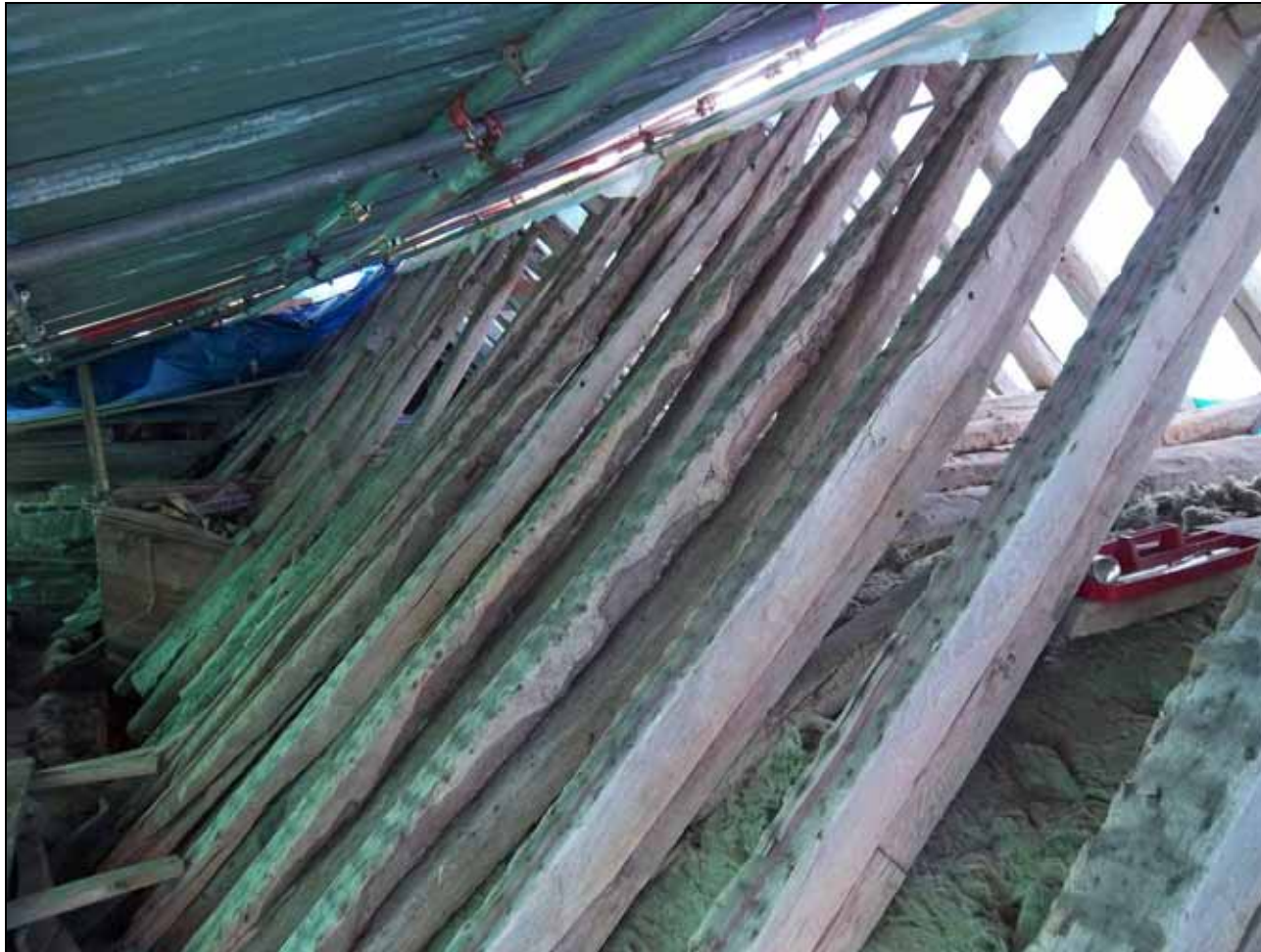
Figure 4: Nave roof showing the backing rafters (photograph taken from the south-east). Photograph Robert Howard
