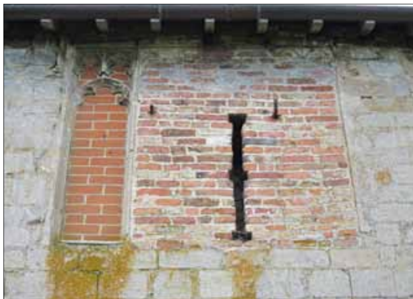
Figure 21. Blocked window, at upper level on south façade.
