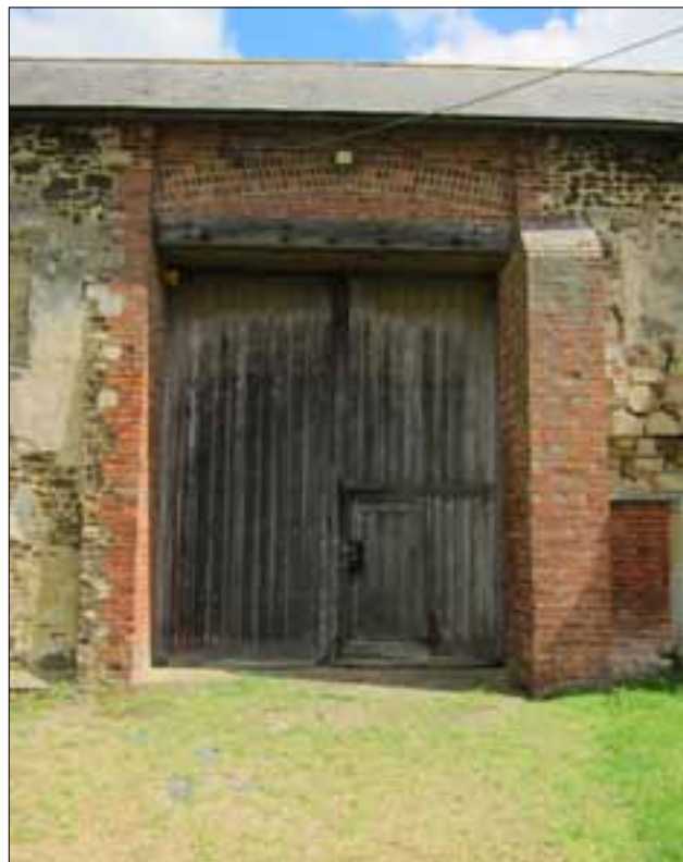
Figure 10. Taking-in door, west façade.
