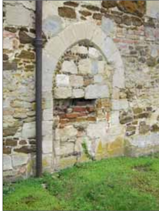
Figure 8. Infilled doorway on west façade.
