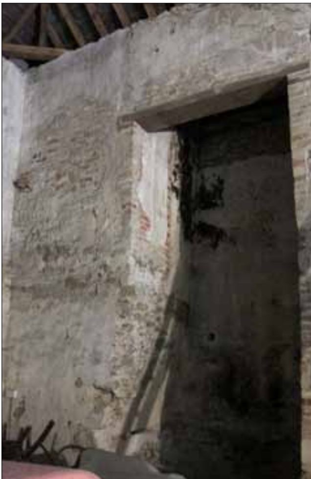
Figure 13. West wall, wing, interior.
