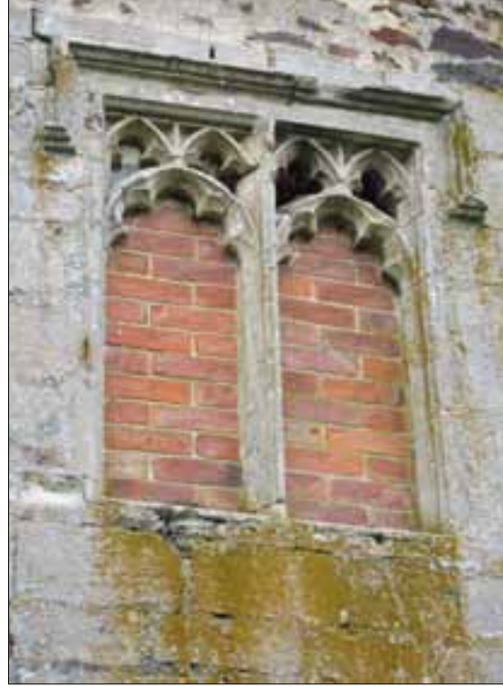
Figure 24. Blocked two-light traceried window with cut-down tracery at upper level on east façade.
