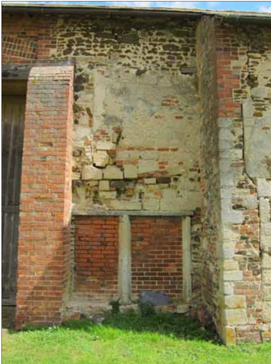
Figure 11. Re-used mullions and worked stone in west façade.
