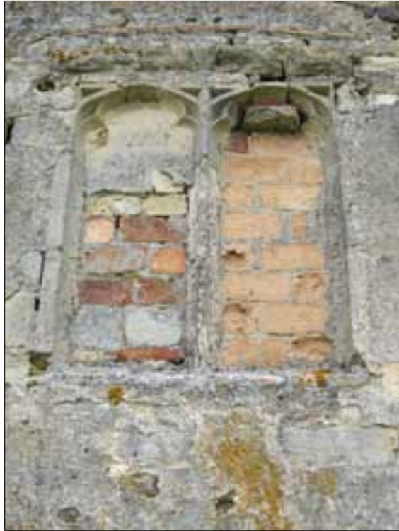
Figure 6. Blocked two-light window at upper level on west façade.
