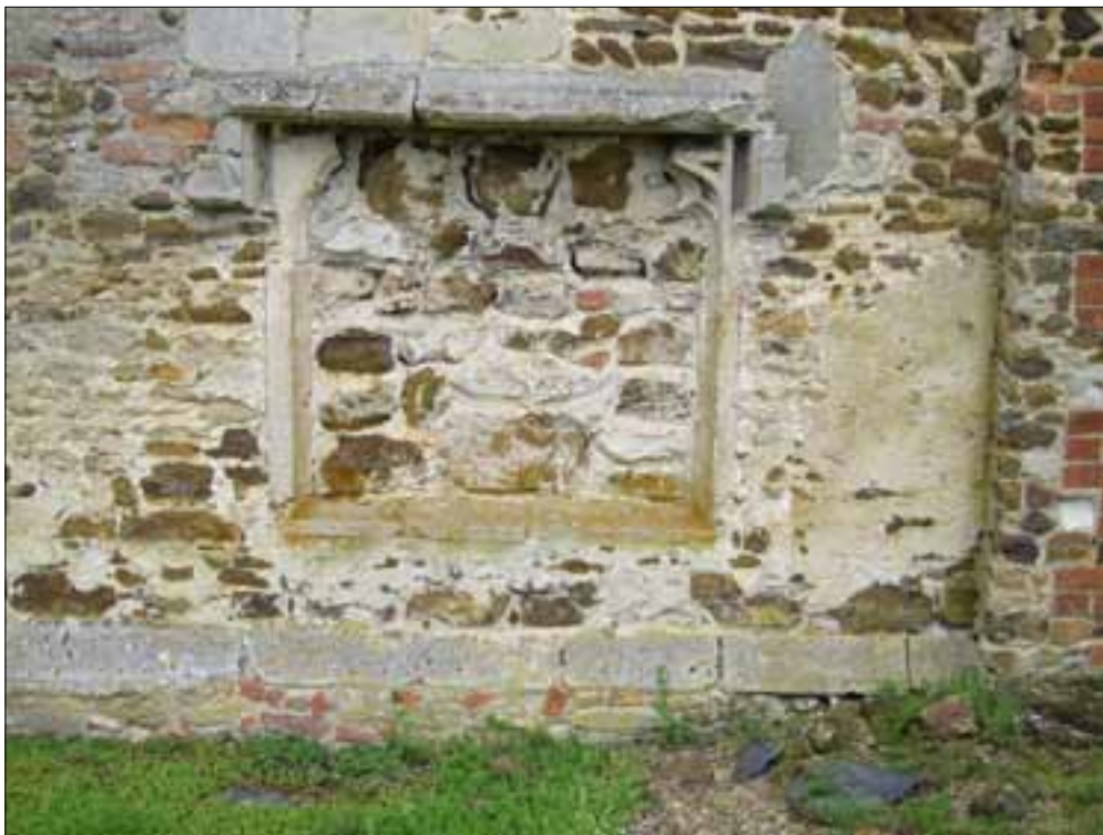
Figure 9. Infilled window at ground level on west façade.
