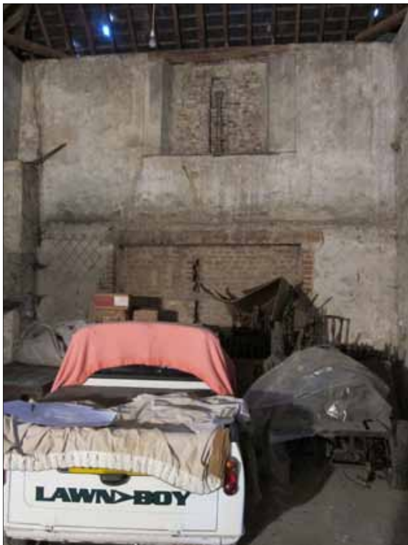
Figure 16. South wall, interior, showing evidence of earlier aperture.
