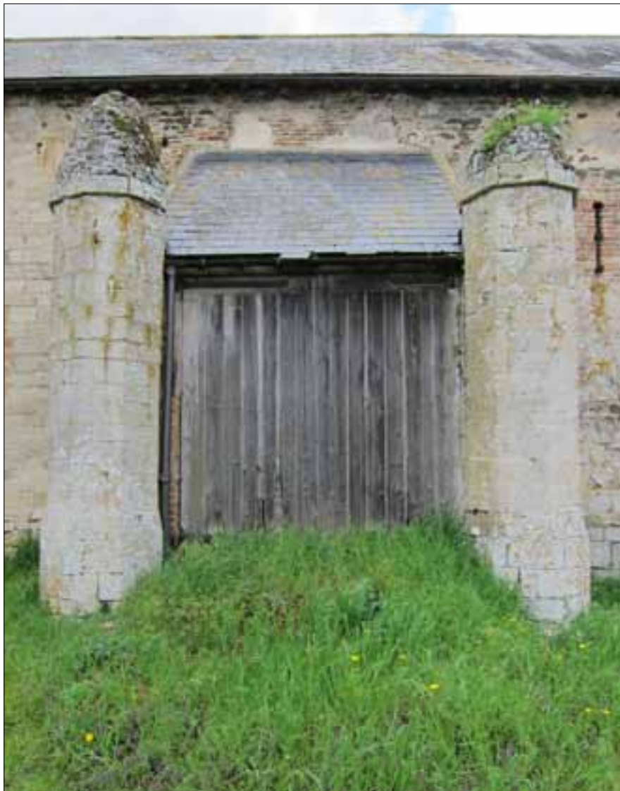
Figure 22. Porch, east façade.
