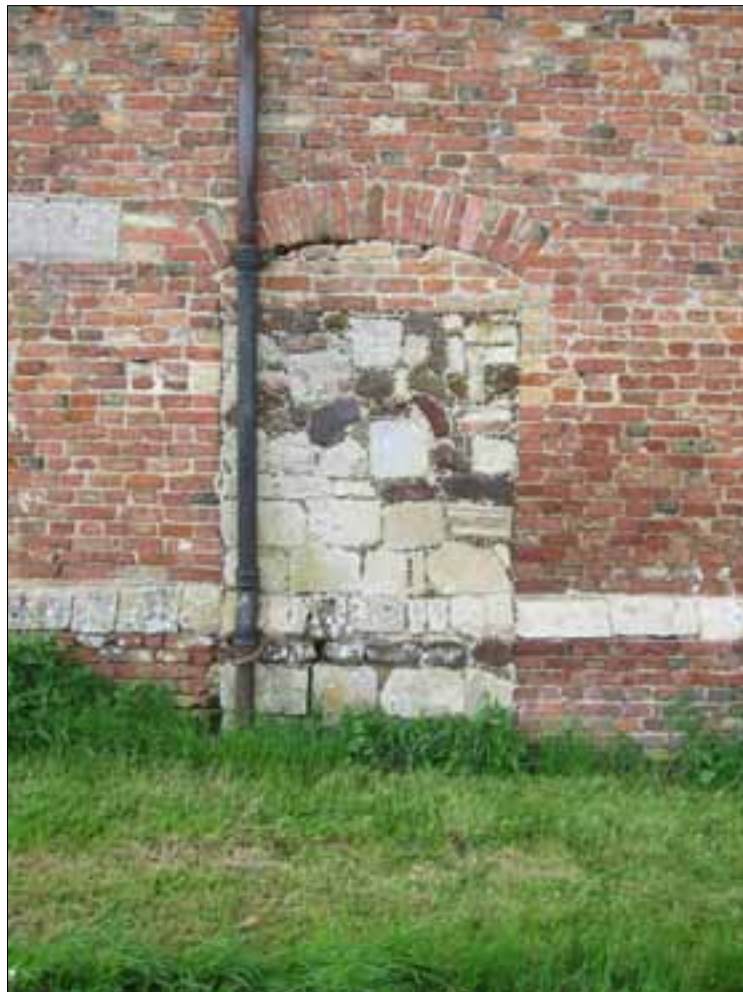
Figure 19. Blocked doorway, east façade.
