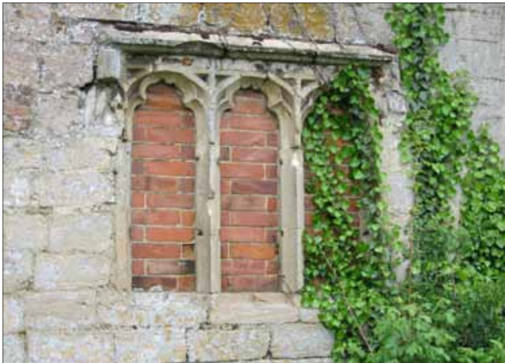
Figure 25. Blocked three-light traceried window at ground level on east façade.
