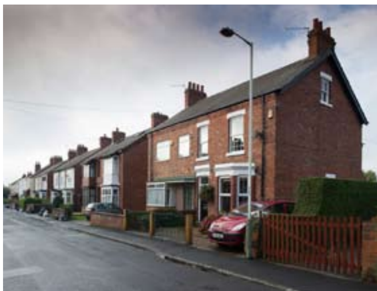
Figure 73 Semi-detached houses on the west side of Milton Street (DPI43802)
