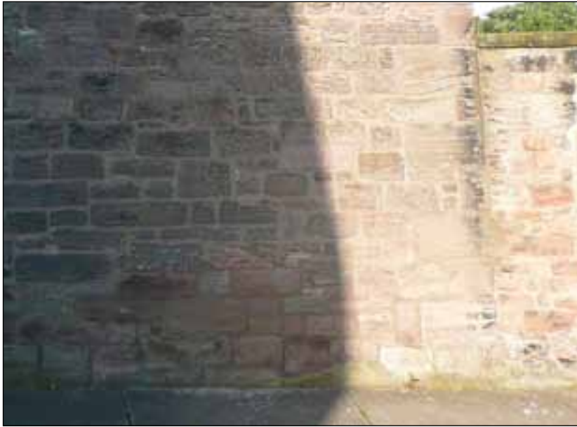
Figure 12. Possible ragged joint on the western elevation (Photograph: Kirsty Tuthill 2011 © English Heritage).
