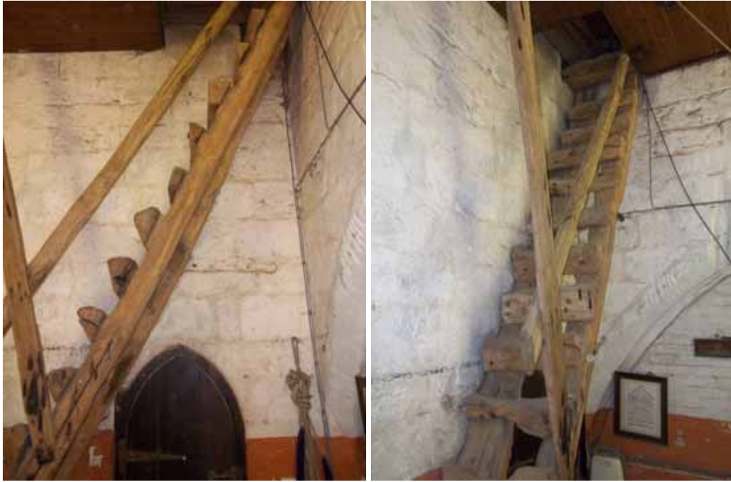
Figure 3a/b: General views of the wooden ladder
