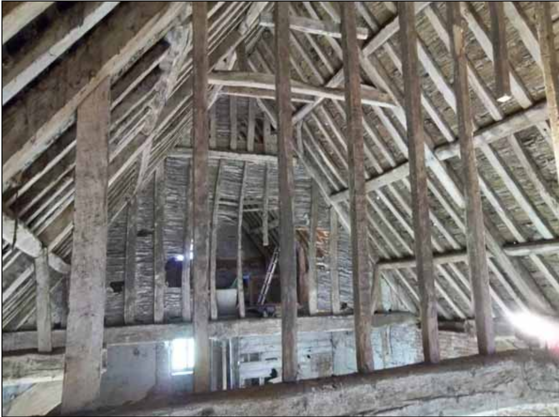
Figure 5: Godwick Great Barn partitioning at truss 5 in the foreground (photograph taken from the south-west) Photograph Robert Howard
