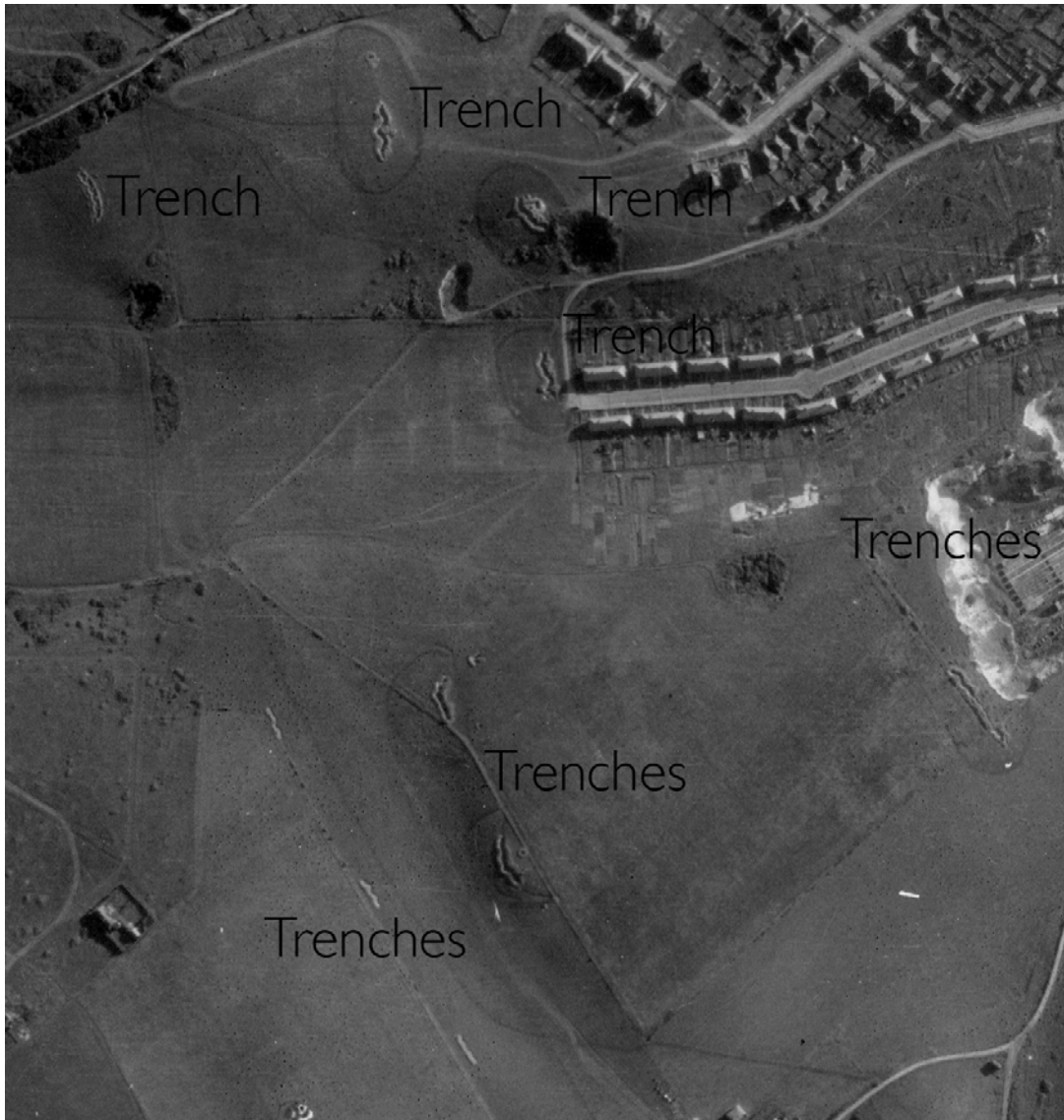
Figure 33 Trenches aligned approximately north-south and enclosing barbed wire defending the westward approach to Newhaven put in place in spring 1940. © English Heritage RAF Photography.
